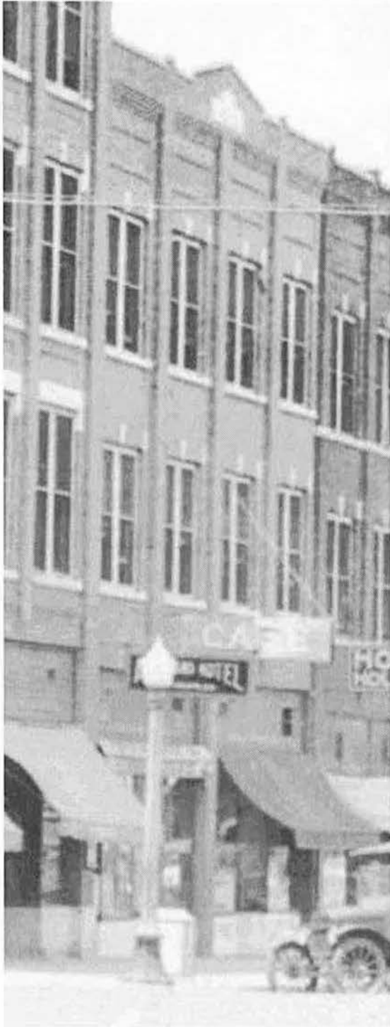
Figure 3: Undated Historic Image (prior to 1924 tornado)
