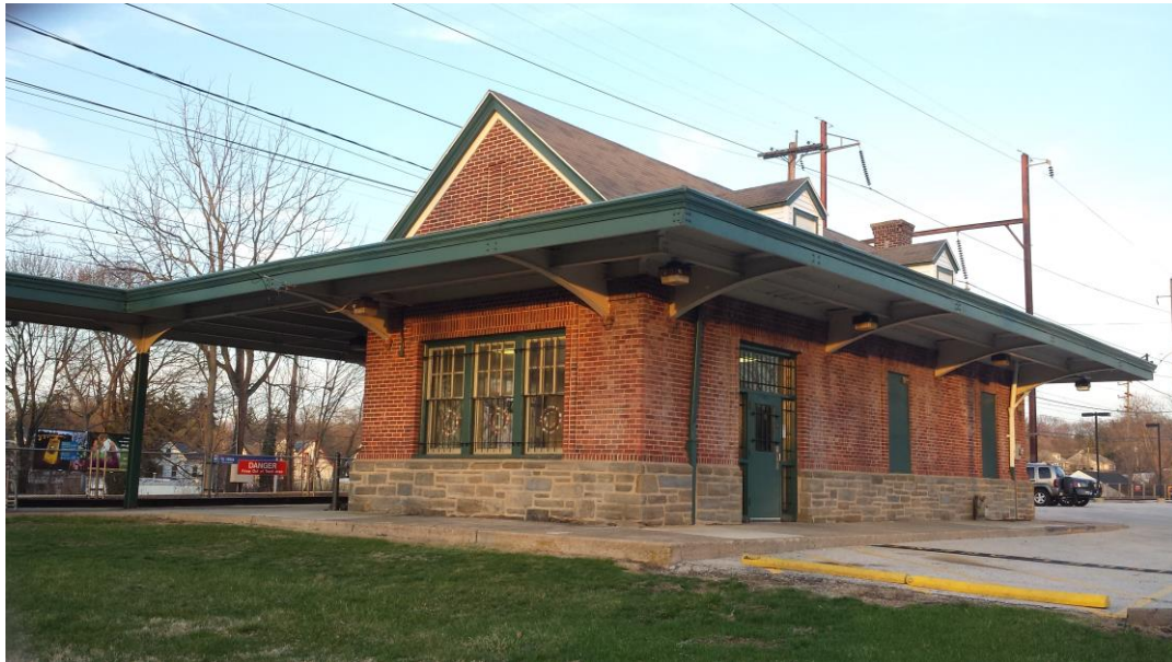
Figure 8, North Hills, View Northeast, Waiting Room
