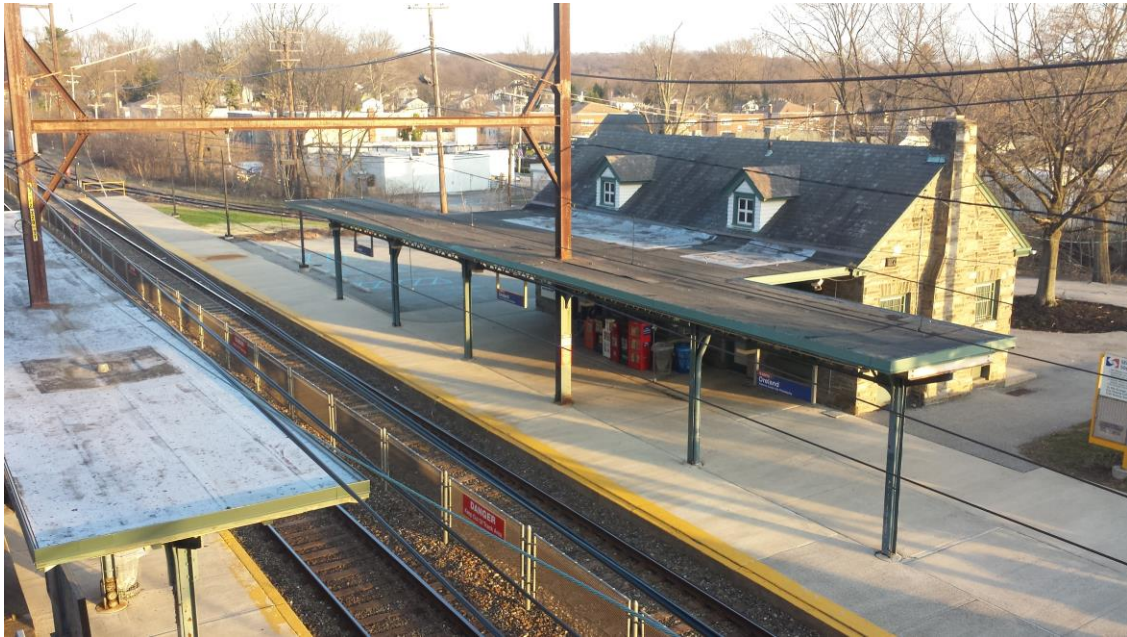
Figure 10, Oreland Station View Southeast
