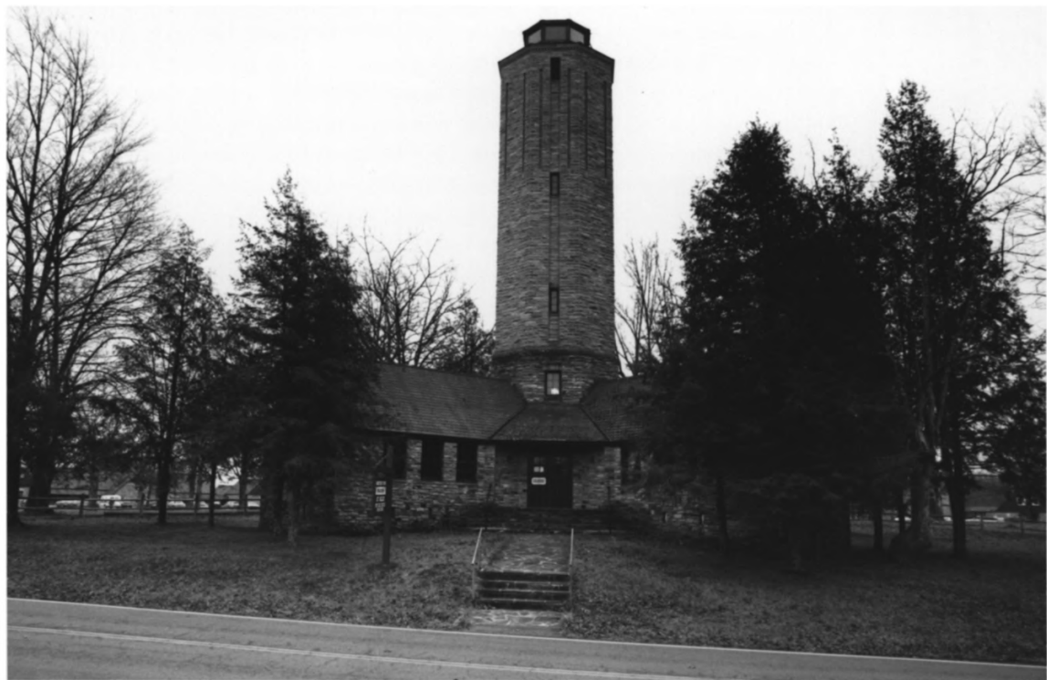
Cumberland Homesteads Historic District # 45 of 64 Cumberland County, TN
