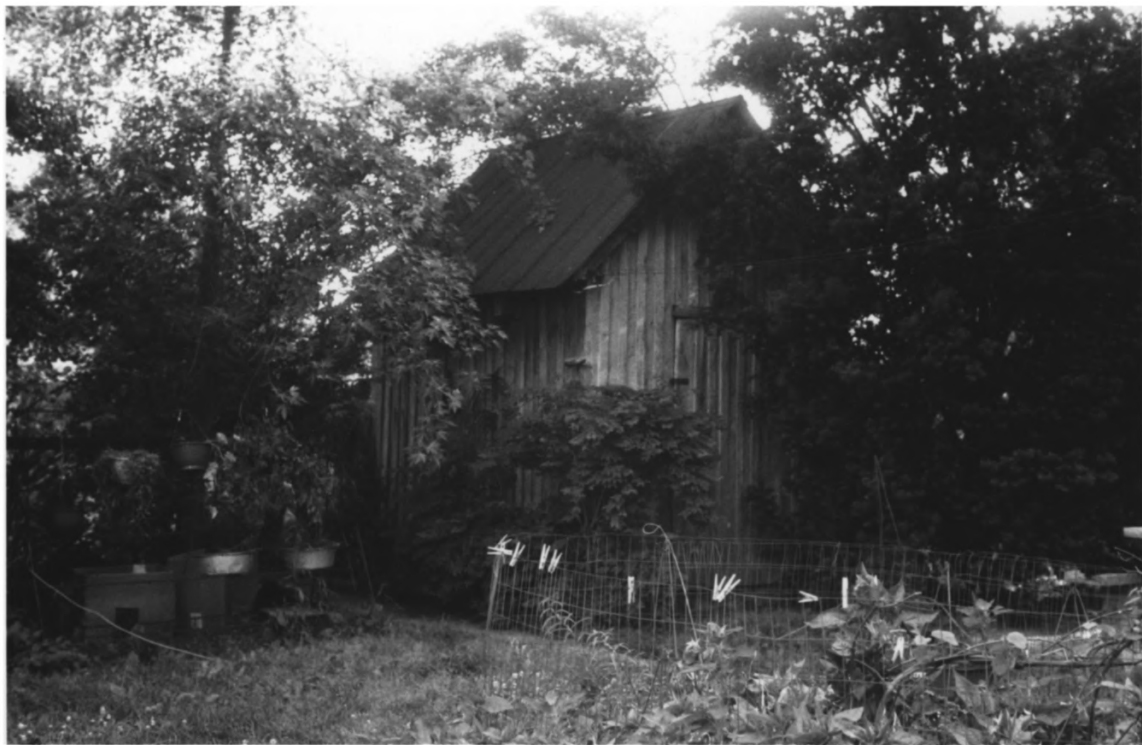
Cumberland Homesteads Historic District # 34 of 64 Cumberland County, TN
