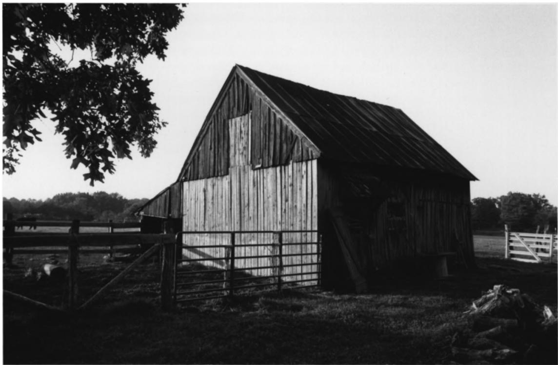
Cumberland Homesteads Historic District # 38 of 64 Cumberland County, TN
