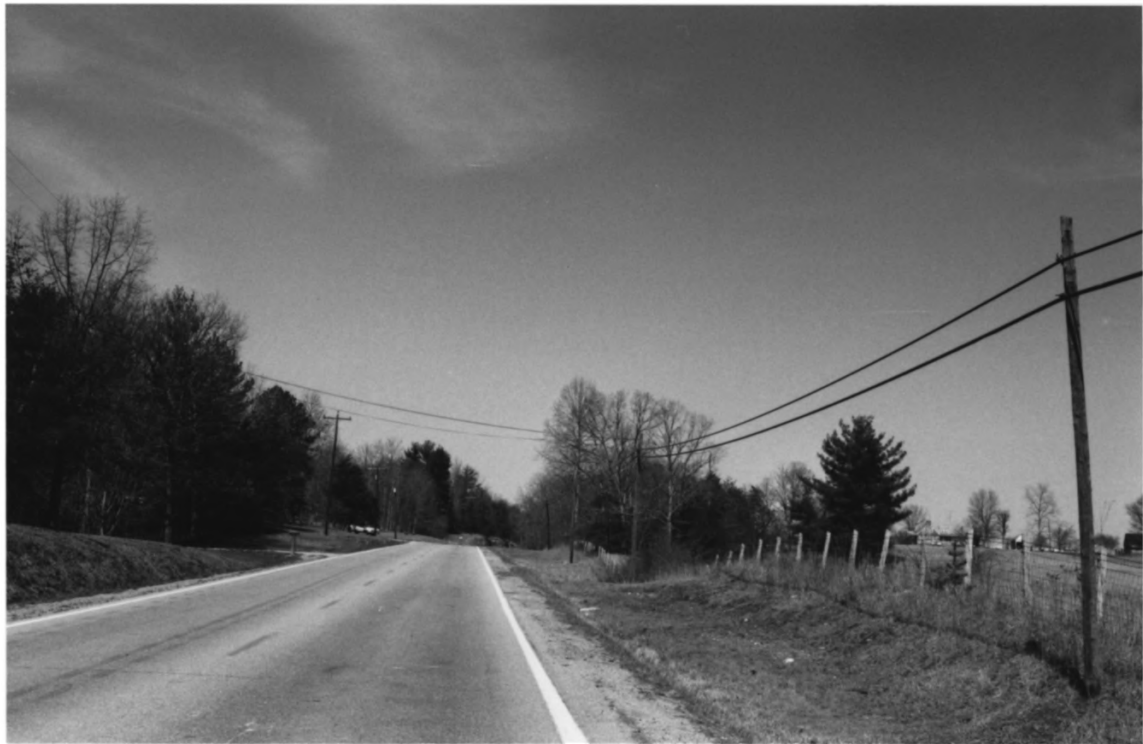
Cumberland Homesteads Historic District . # 4 of 64 Cumberland County, TN
