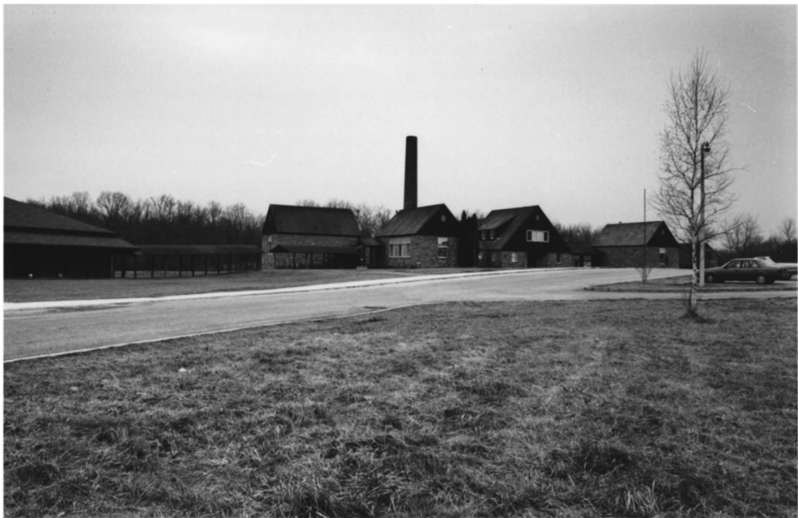
Cumberland Homesteads Historic District #47 of 64 Cumberland County, TN
