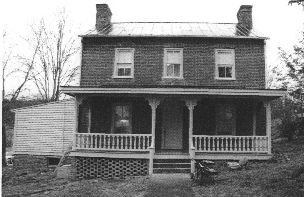
Figure 2. Main, south, elevation of Maden Hall while undergoing repairs (D. Brock, 03/2009).
