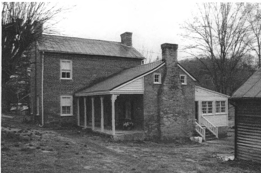
Figure 6. Looking southwest at Maden Hall, showing the original rear ell and recently repaired side porch, which faces Kingsport Highway (D. Brock 03/2009).
