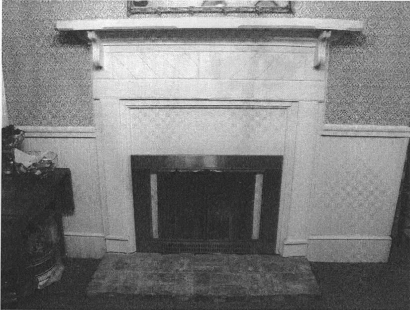
Figure 12. Looking west at the west parlor's 1910s fireplace mantel (D. Brock 03/2009).
