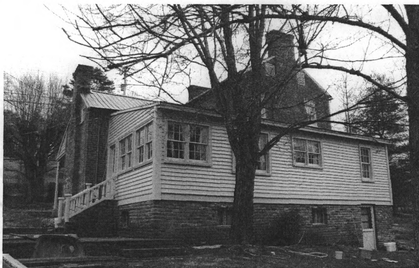
Figure 7. Looking southeast at Maden Hall, showing the kitchen/bathroom wing and brick patio added in the 1970s, which face away from the highway (D. Brock 03/2009).
