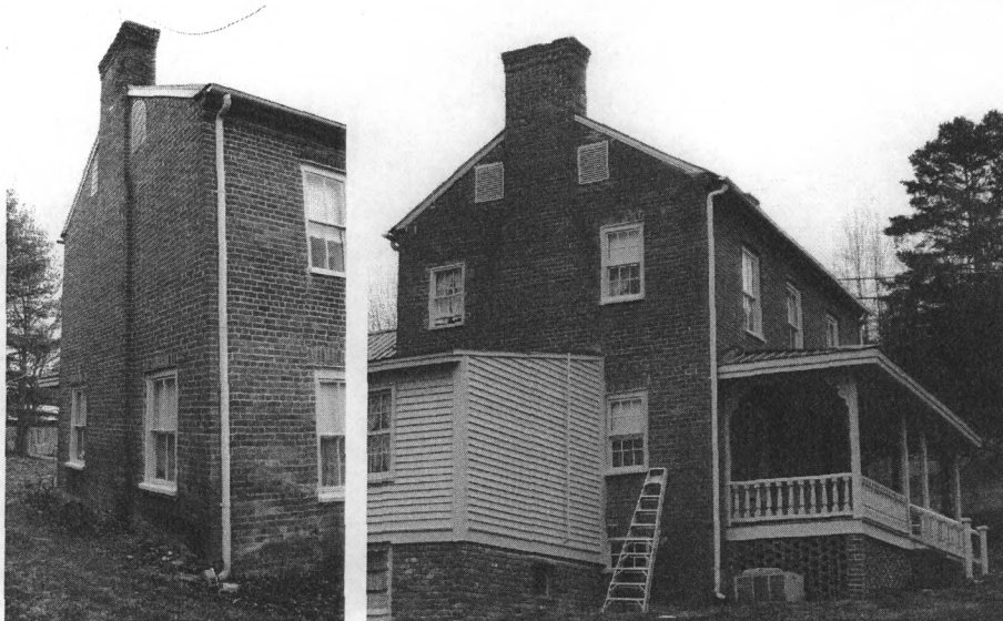
Figure 4. Maden Hall, looking southwest (left) and northeast (right), showing the different architectural designs of the east and west elevations. The east elevation, facing Kingsport Highway, exhibits more elaborate details and fewer windows (D. Brock 03/2009). Note: faux shutters and non-historic window trim were recently removed on the entire house as part of restoration work.
