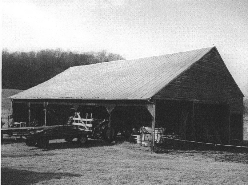
Figure 20. Looking southwest at the cantilever barn, constructed with double log cribs for William Ross II in the mid-nineteenth century; the tractor shed was renovated in 1956 (R. Jones, 01/2009).
