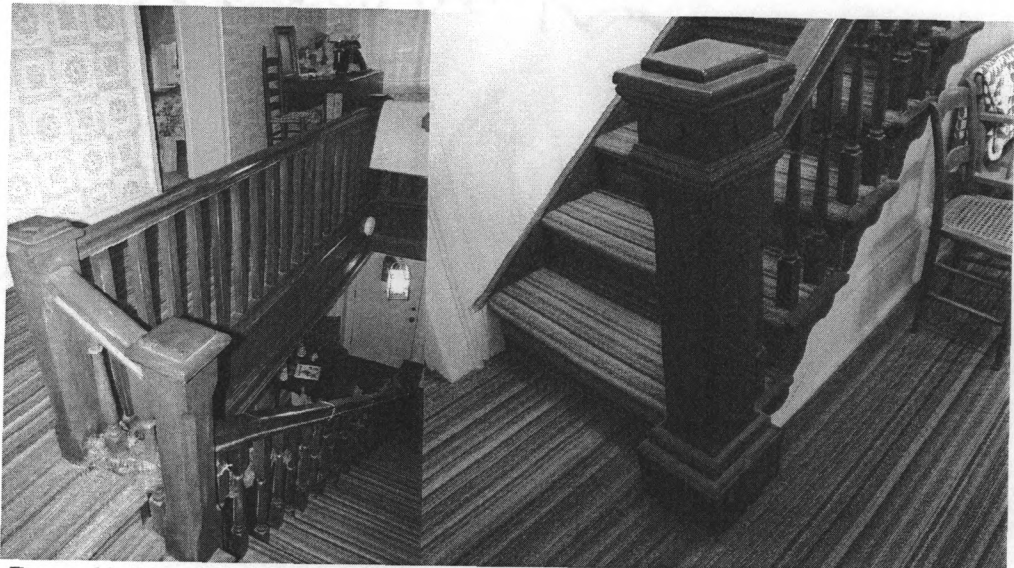
Figure 11. Views of the 1910s staircase railing and newel (D. Brock 01/2009 & 03/2009).
