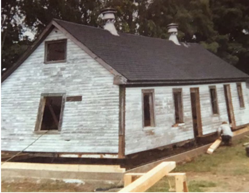
Figure 14: 1978 photograph of hatchery during remodeling (Collection of property owners)
