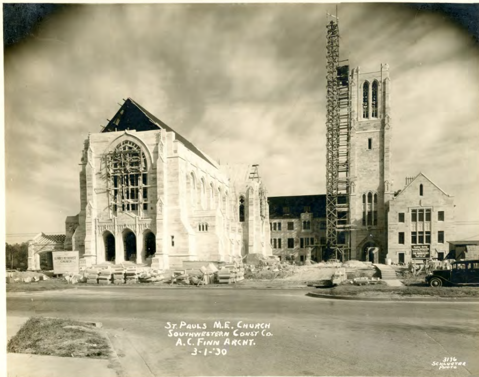
Figure 7 – St. Paul's under construction. March 1, 1930. Courtesy Houston Metropolitan Research Center.
