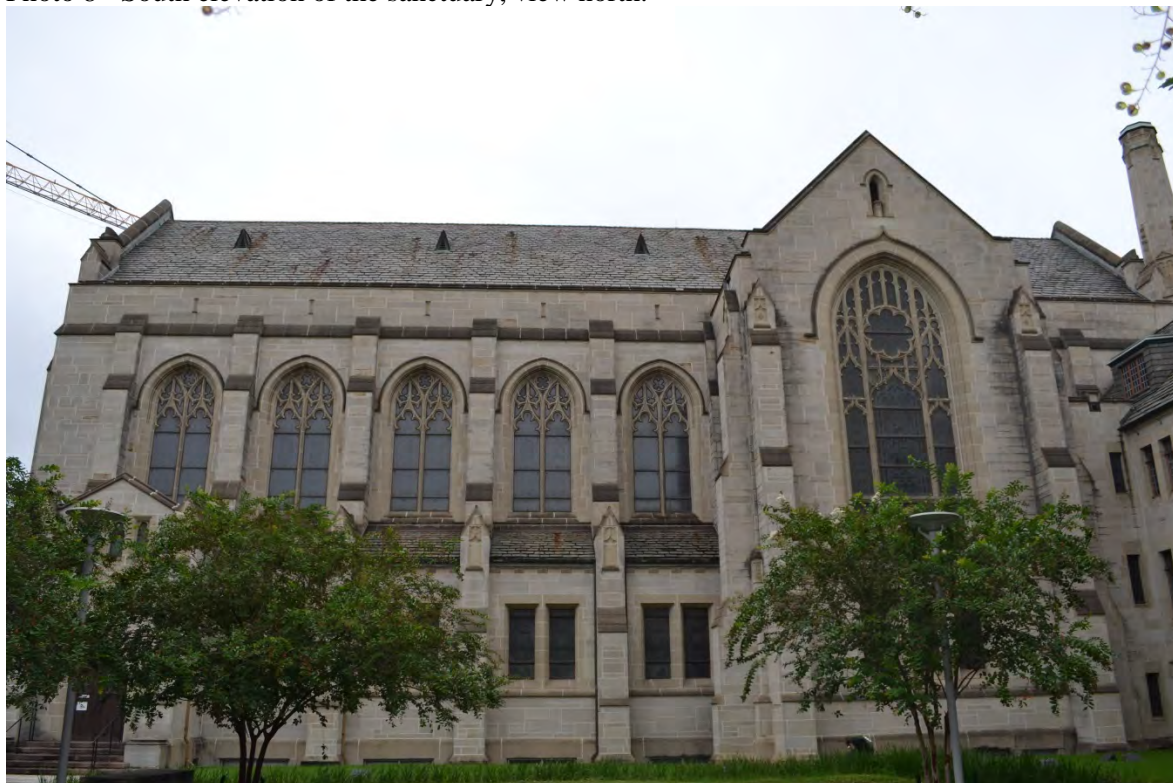
Photo 8 - South elevation of the sanctuary, view north.
