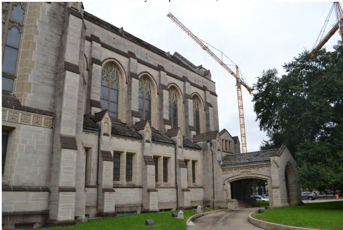
Photo 5 - North elevation of the sanctuary with porte cochere, view southwest.
