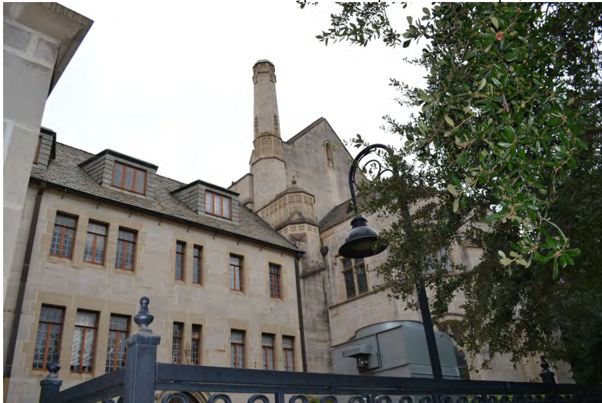
Photo 11 - East elevation of the administration hyphen with a partial view of the apse, view northwest.
