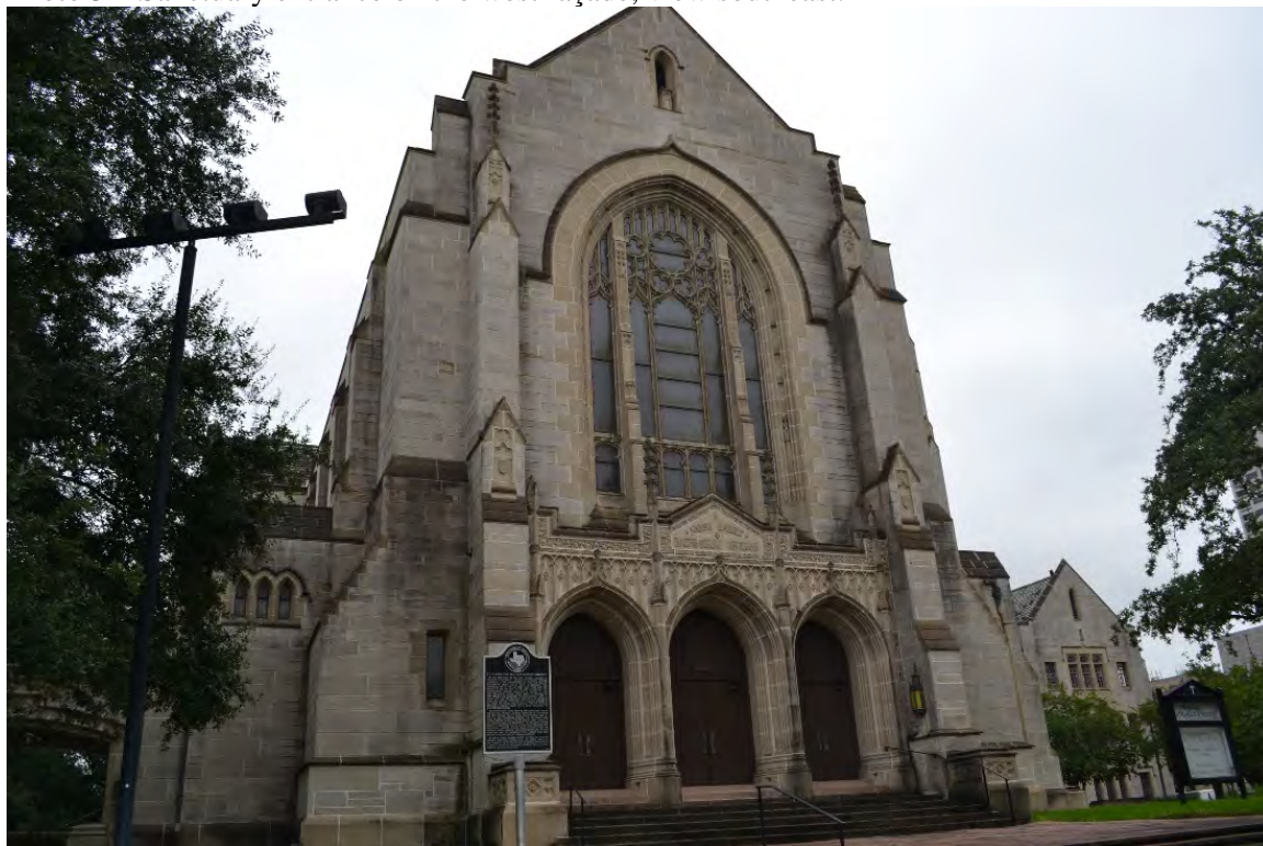
Photo 3 – Sanctuary entrance on the west façade, view southeast.
