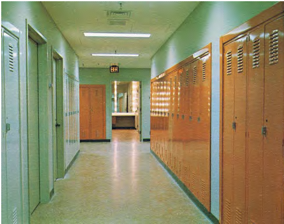
Figure 4: Historic photograph of backstage hallway, c. 1974
