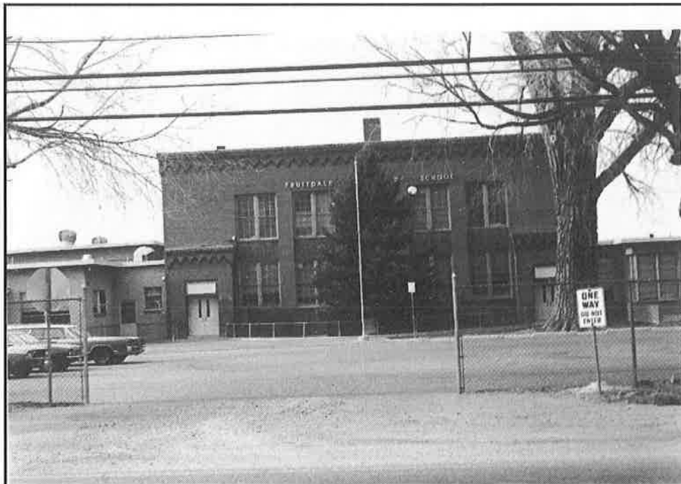
Figure 7: Fruitdale School of 1927 main section. Photo taken by Robert J. Olson, May 22, 1999, in the files of the Office of Archaeology and Historic Preservation, Denver, Colorado
