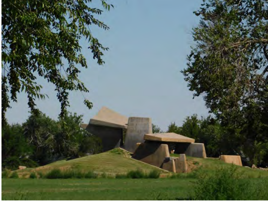
1 of 17. The Henge and its landscaped setting, photographer facing north.
