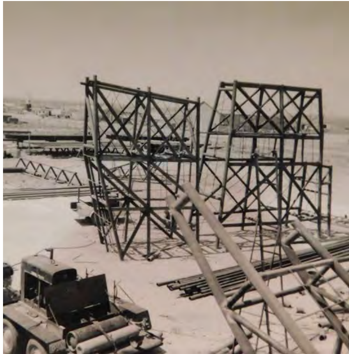
Figure 14. Construction of steel-frame megaliths, photo by Herbert Goldman, June 1963.
