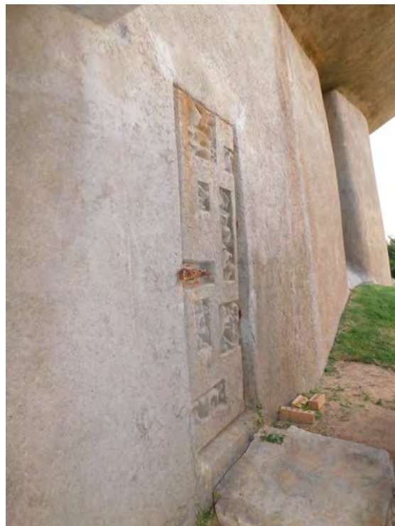
16 of 17. Southeast concrete door, photographer facing southwest.
