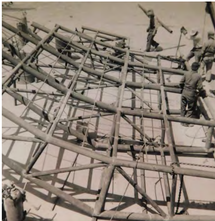
Figure 13. Construction of steel-frame, photo by Herbert Goldman, 1963.
