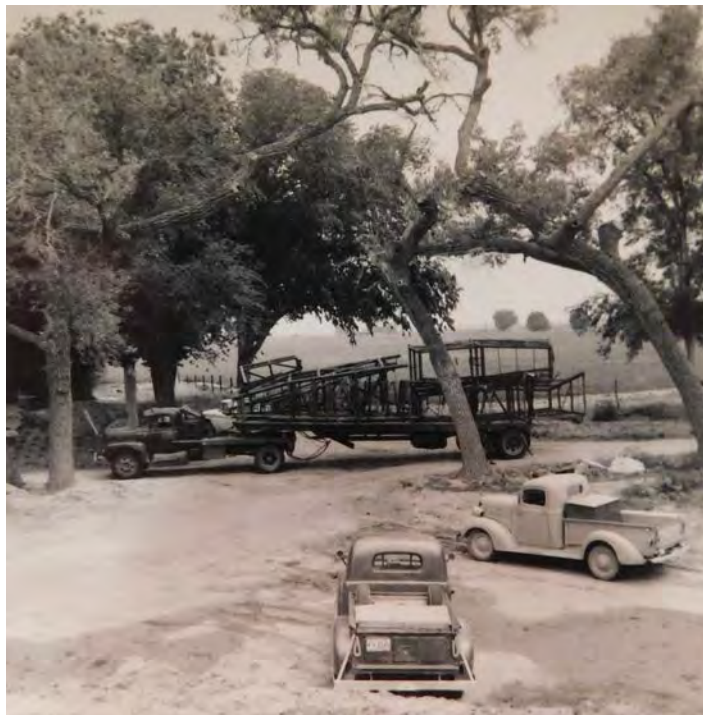
Figure 15. Transporting prefabricated steel frame to site, photo by Herbert Goldman, 1963.
