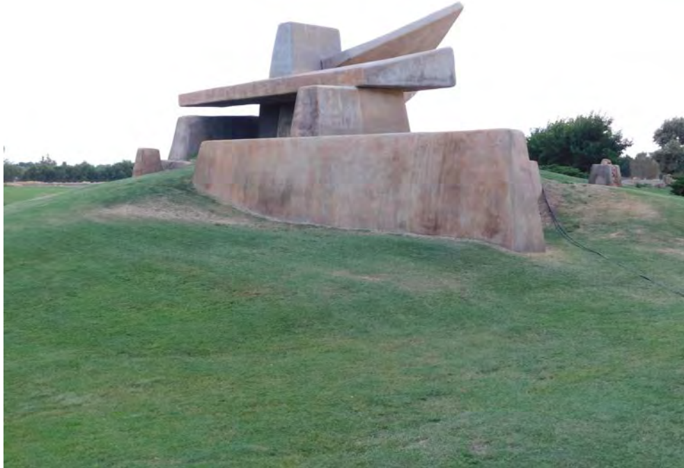
11 of 17. Large northeast wall in foreground, photographer facing southwest.
