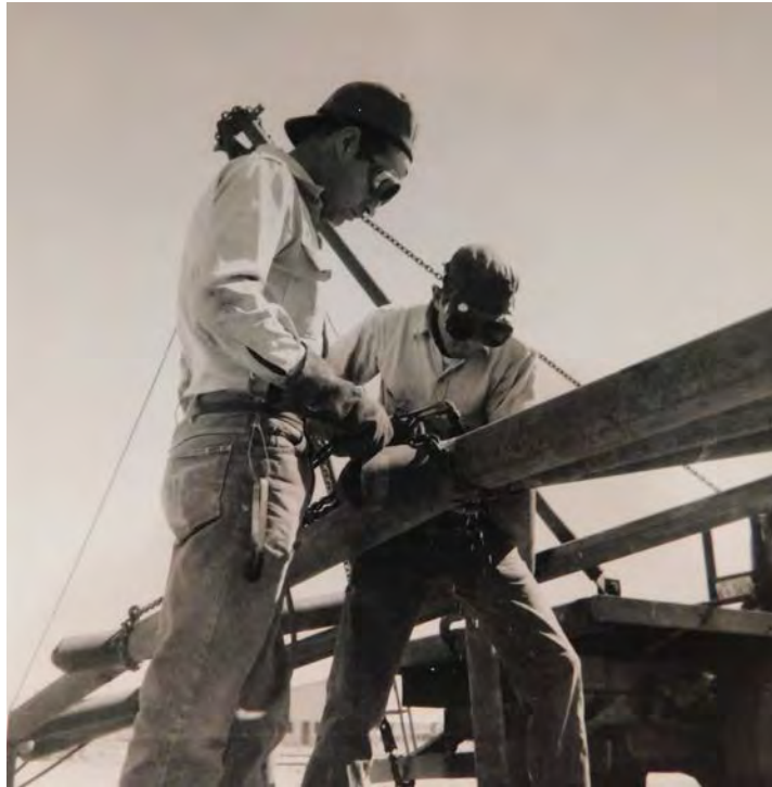
Figure 12. Welding of steel frame, photo by Herbert Goldman, June 1963.
