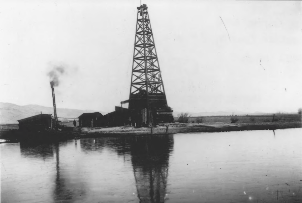
THE MCKENZIE OIL WELL NEAR BOULDER, COLO., 1902. DERRICK AVERAGE IN HEIGHT FROM 76 TO 80 FT., 20 FT. AT BASE.
