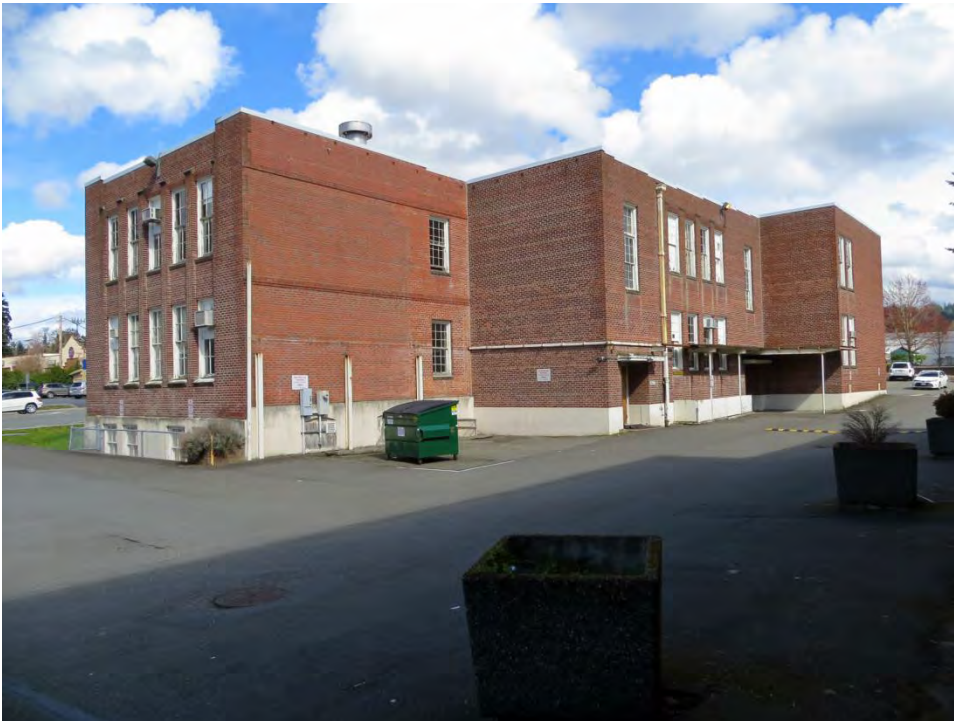
7) Southwest corner showing 1909 wall section (note brick color).
