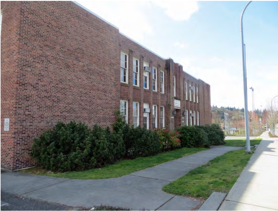
2) Entrance façade north elevation. View from northeast.
