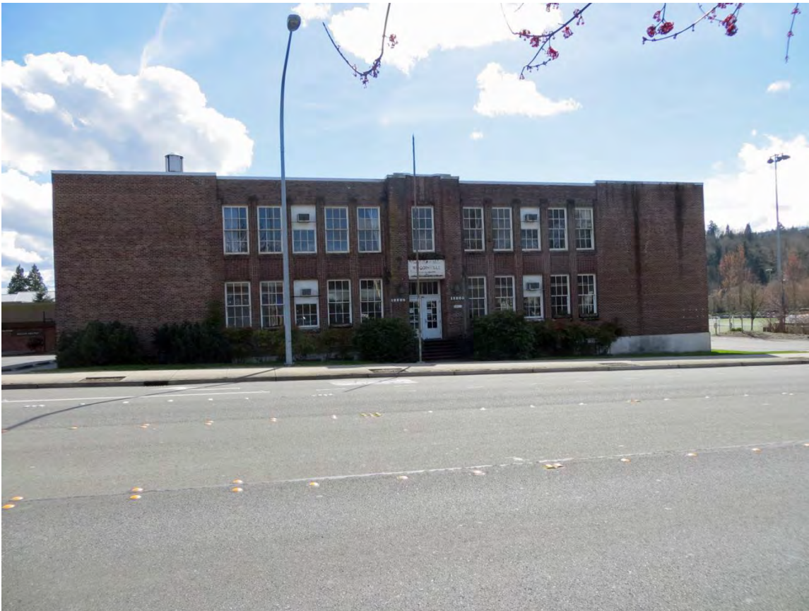
1) Entrance façade north elevation. View from north.
