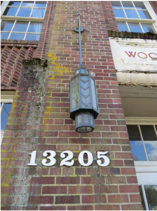
4) Detail of fixture and brickwork, north elevation.
