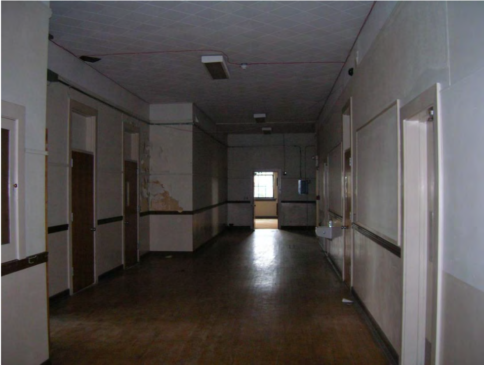
12) Hall first floor corridor. View to west.
