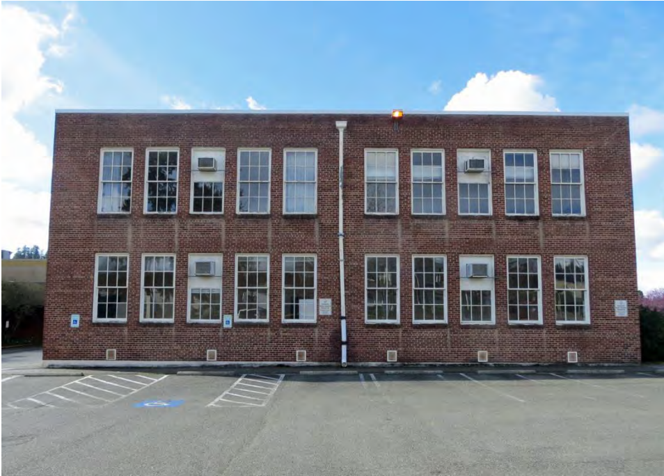
6) East elevation – 1948 addition.
