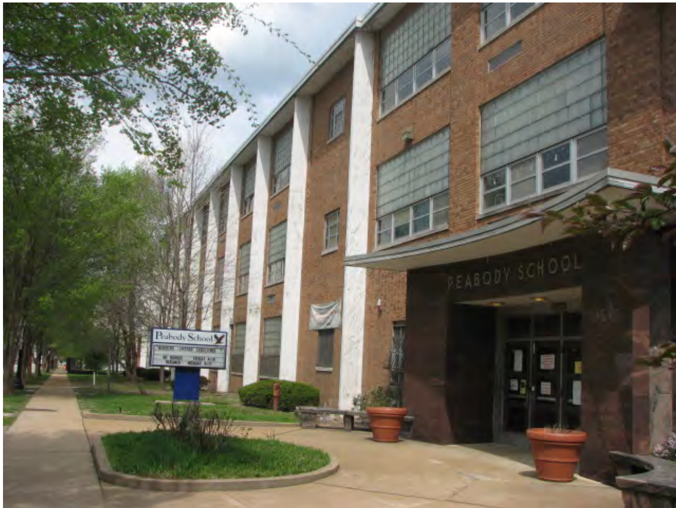
Figure 14. Peabody School, located at 1224 S. 14 th Street, was constructed in 1957 for the Darst-Webbe public housing project. Photo: Ruth Keenoy, 24 March 2017).
