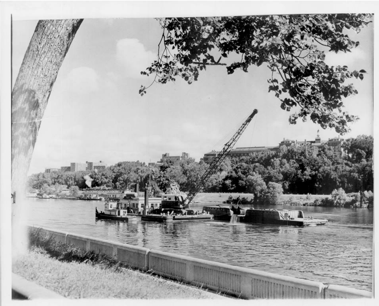
Three tenders were used to assist the William A. Thompson in dredging the Upper Mississippi River. Shown next to the crane is the tender Daniel Bates. In the far left below the building and the boat with the smoke stack is the Joseph Throckmorton - now the Elizabeth Lea . The third tender not shown was the David Smith Harris. Date unknown (Courtesy of the Army Corps of Engineers)
