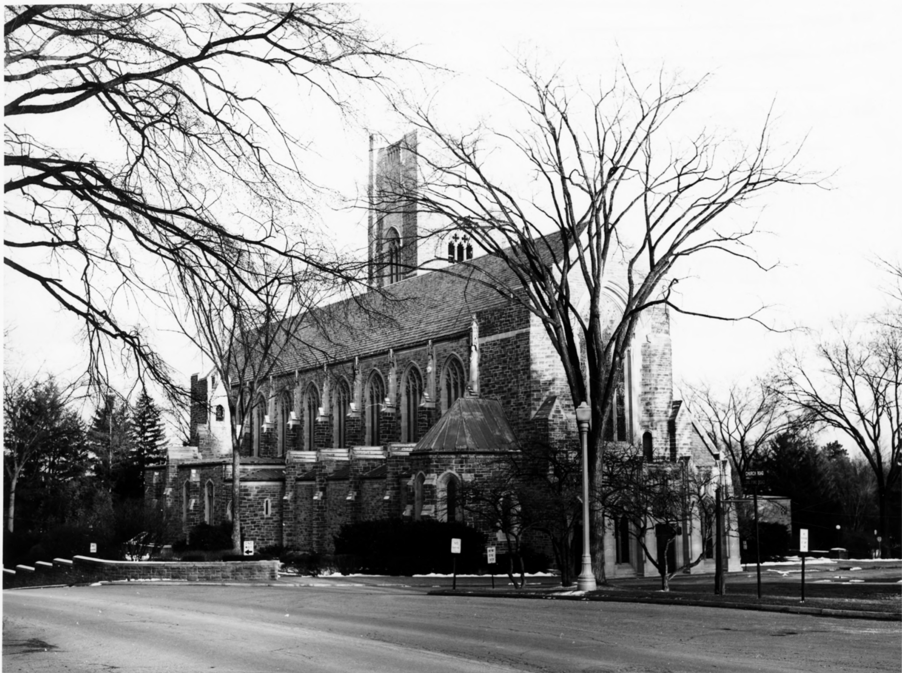
CRANBROOK, Bloomfield Hills, Michigan Christ Church, Cranbrook 1959 Photo credit: Cranbrook
