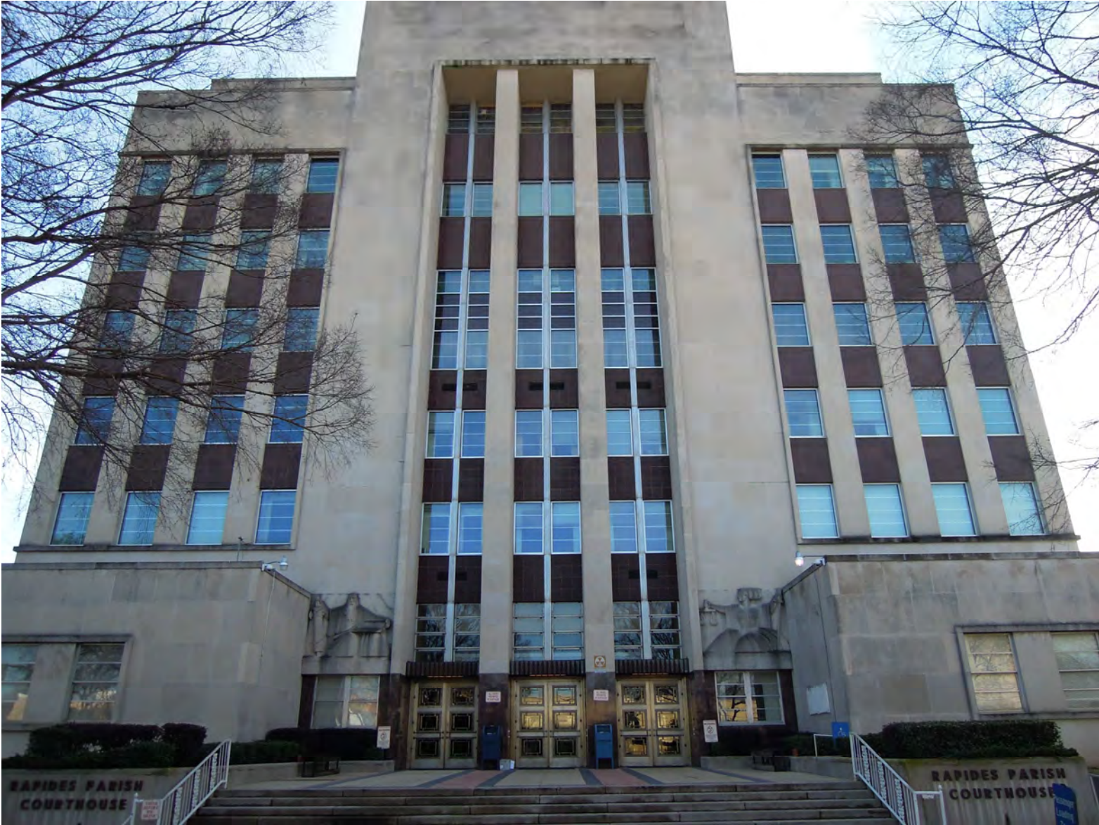
Figure 11. Rapides Parish Courthouse; camera facing east. Image courtesy of the author.
