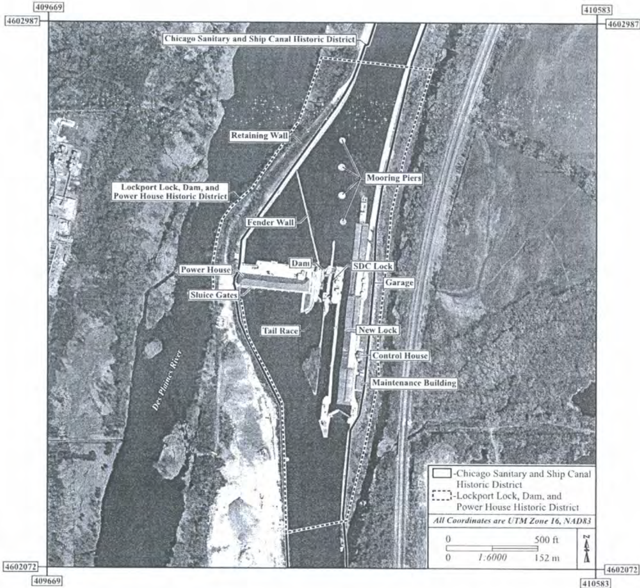
Figure 29: The Lockport Lock, Dam, and Power House Historic District.
