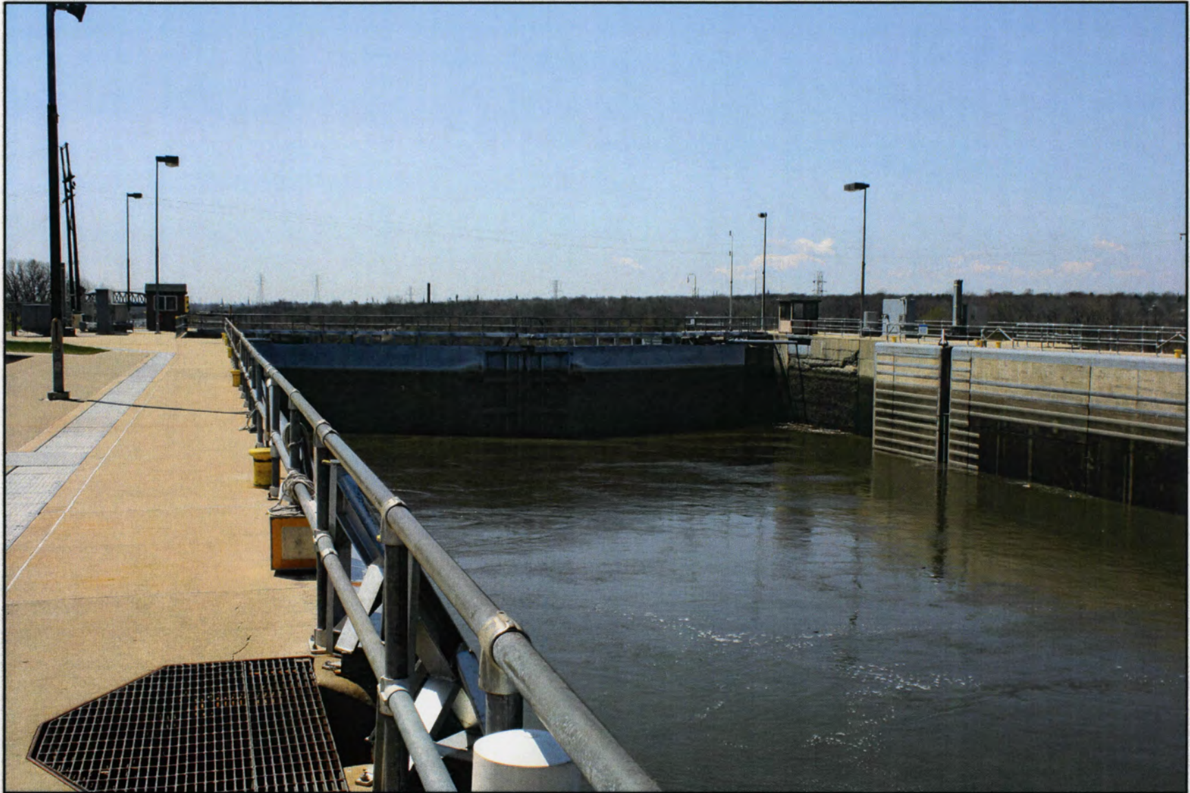
IL_Cook County_Chicago Sanitary and Ship Canal Historic District_0057
