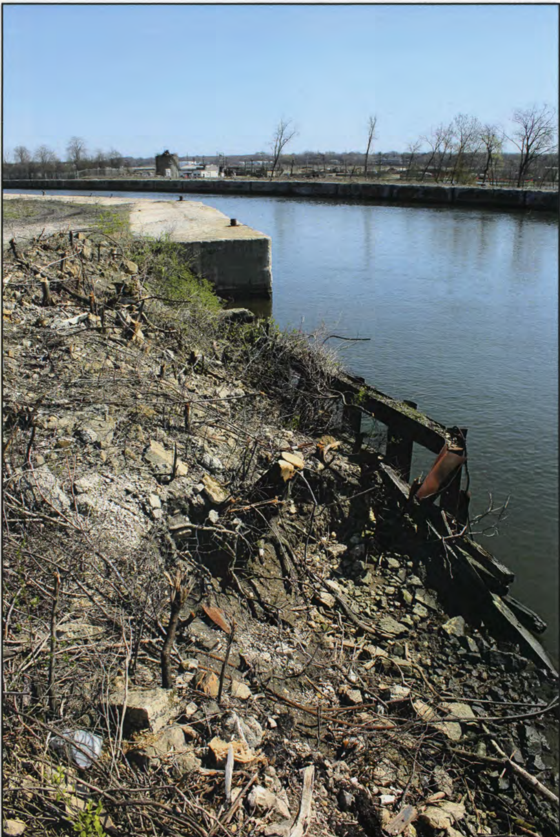
IL_Cook County_Chicago Sanitary and Ship Canal Historic District_0027
