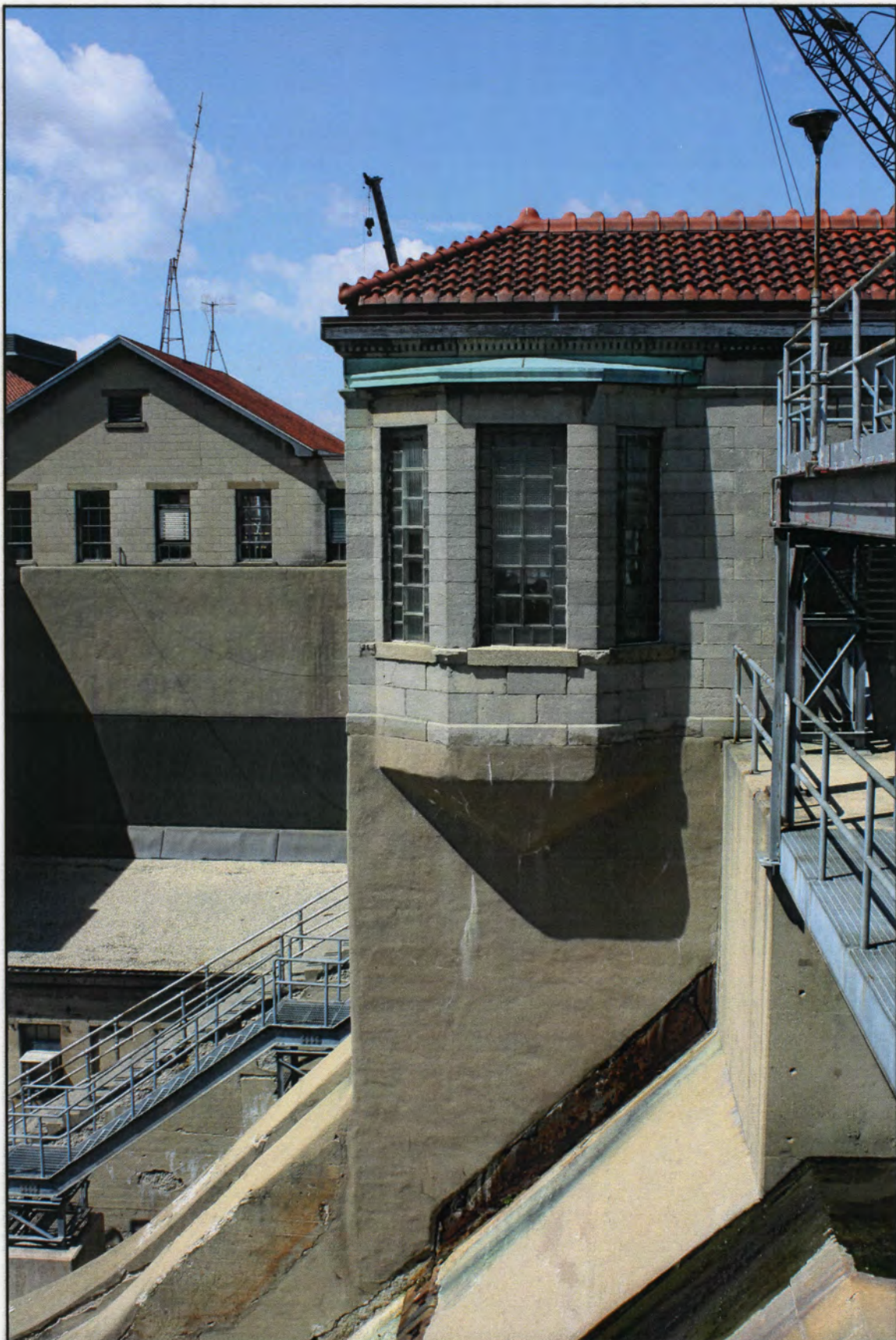
IL_Cook County_Chicago Sanitary and Ship Canal Historic District_0061
