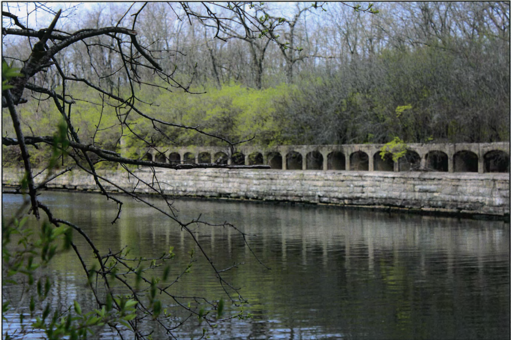
IL_Cook County_Chicago Sanitary and Ship Canal Historic District_0124
