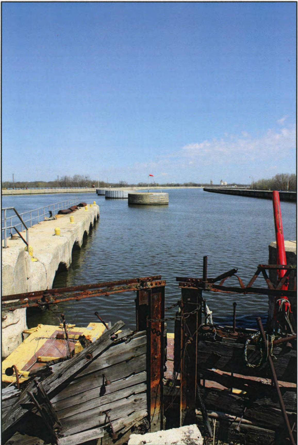
IL_Cook County_Chicago Sanitary and Ship Canal Historic District_0047
