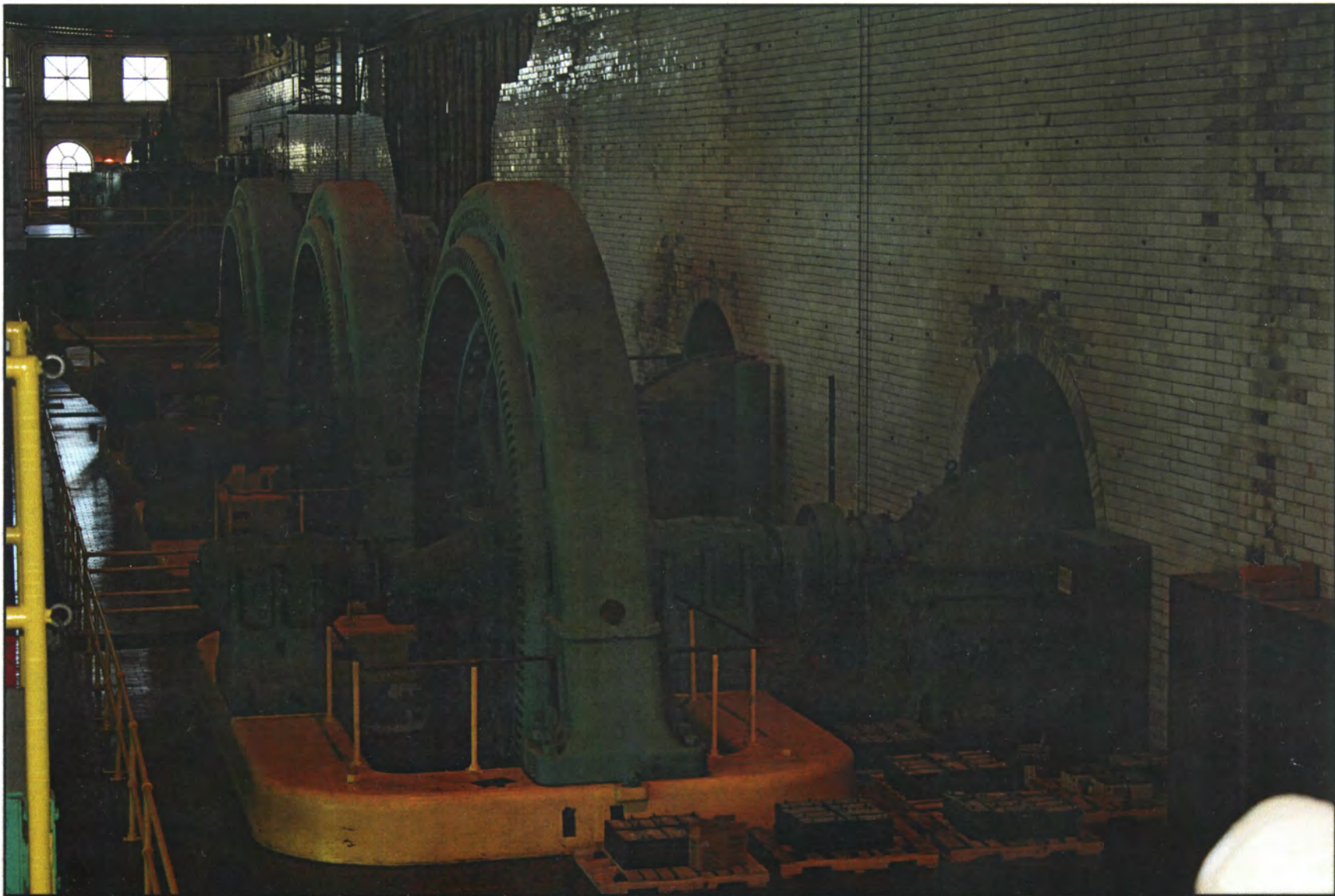
IL_Cook County_Chicago Sanitary and Ship Canal Historic District_0038
