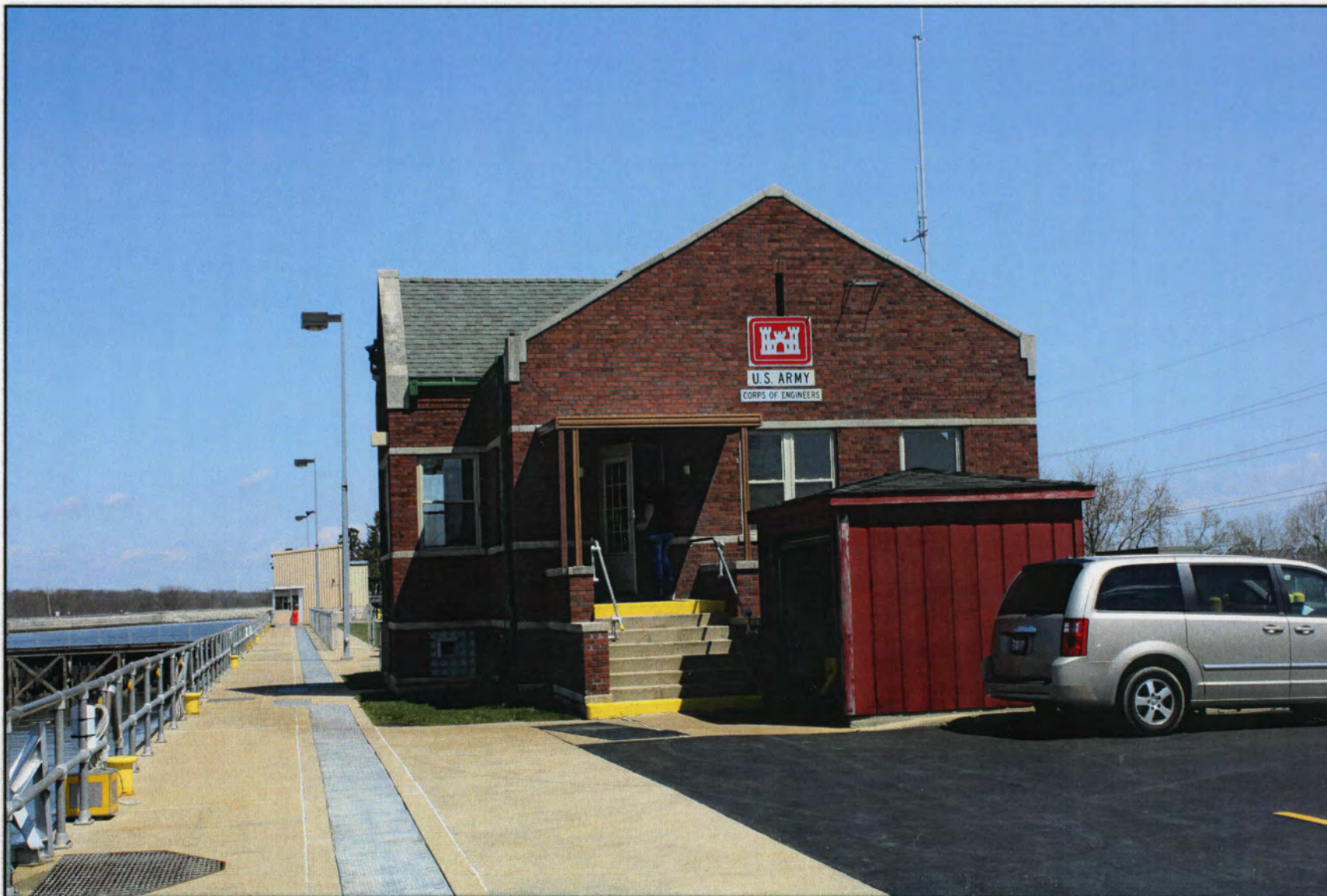
IL_Cook County_Chicago Sanitary and Ship Canal Historic District_0059
