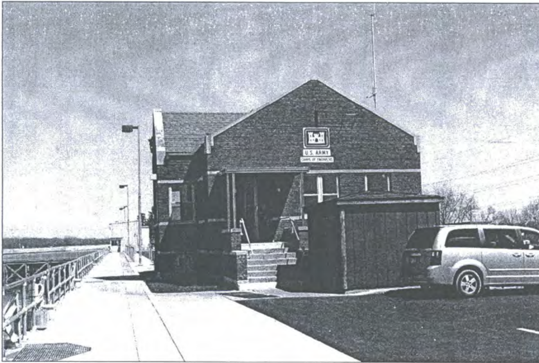
Figure 38: South façade of the Lockport Control Station, Will County, Illinois. View to the north. (Photographed by Eyan Bond, April 22, 2009). Digital image on file at Bear Creek Archeology, Cresco, Iowa.
