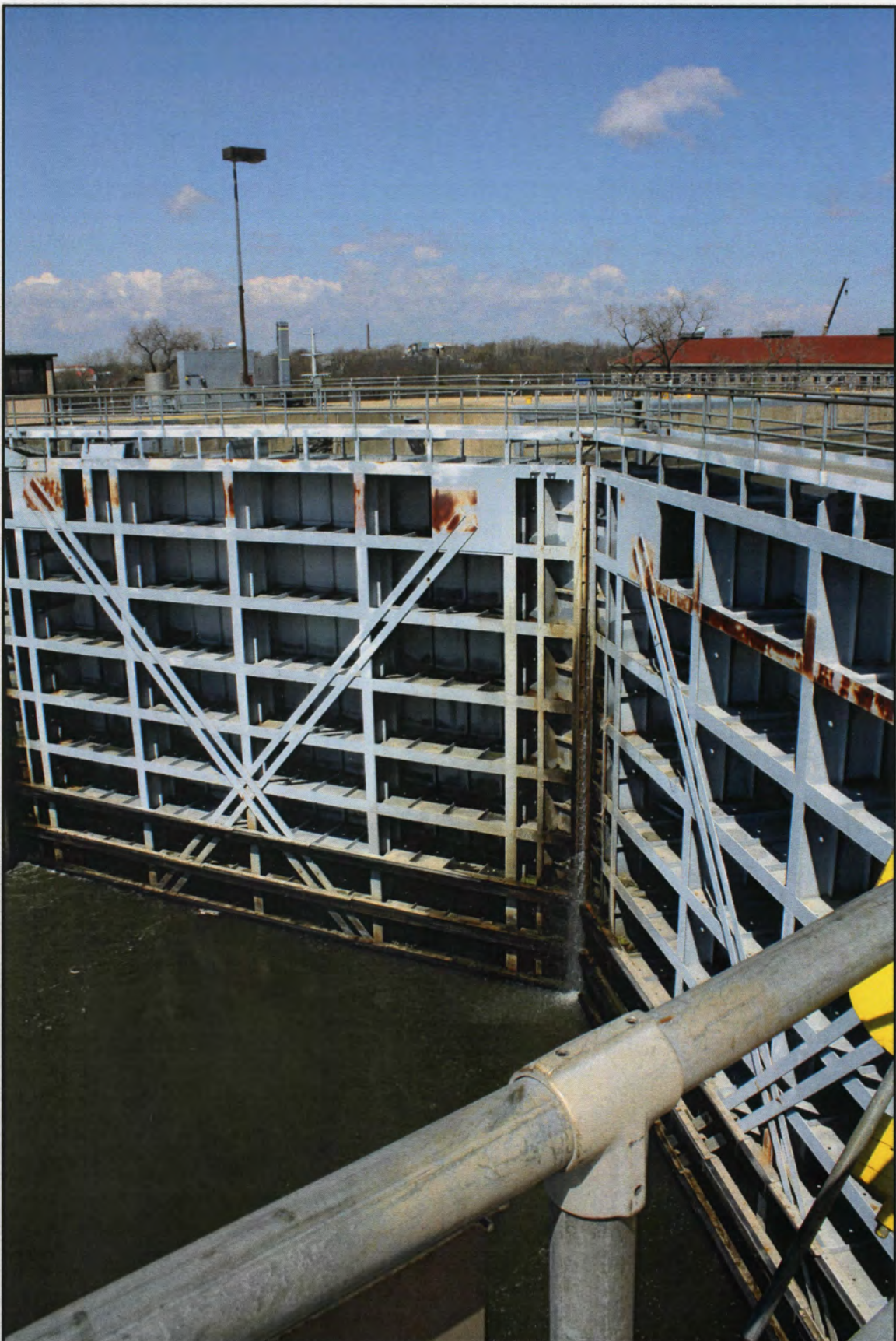
IL_Cook County_Chicago Sanitary and Ship Canal Historic District_0060
