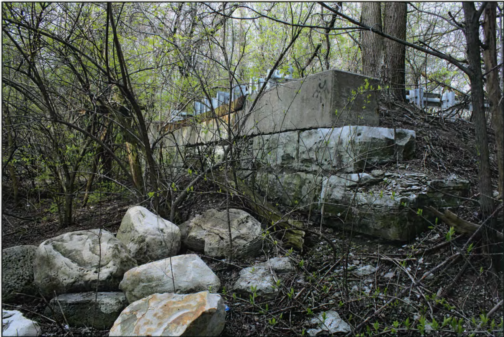
IL_Cook County_Chicago Sanitary and Ship Canal Historic District_0106
