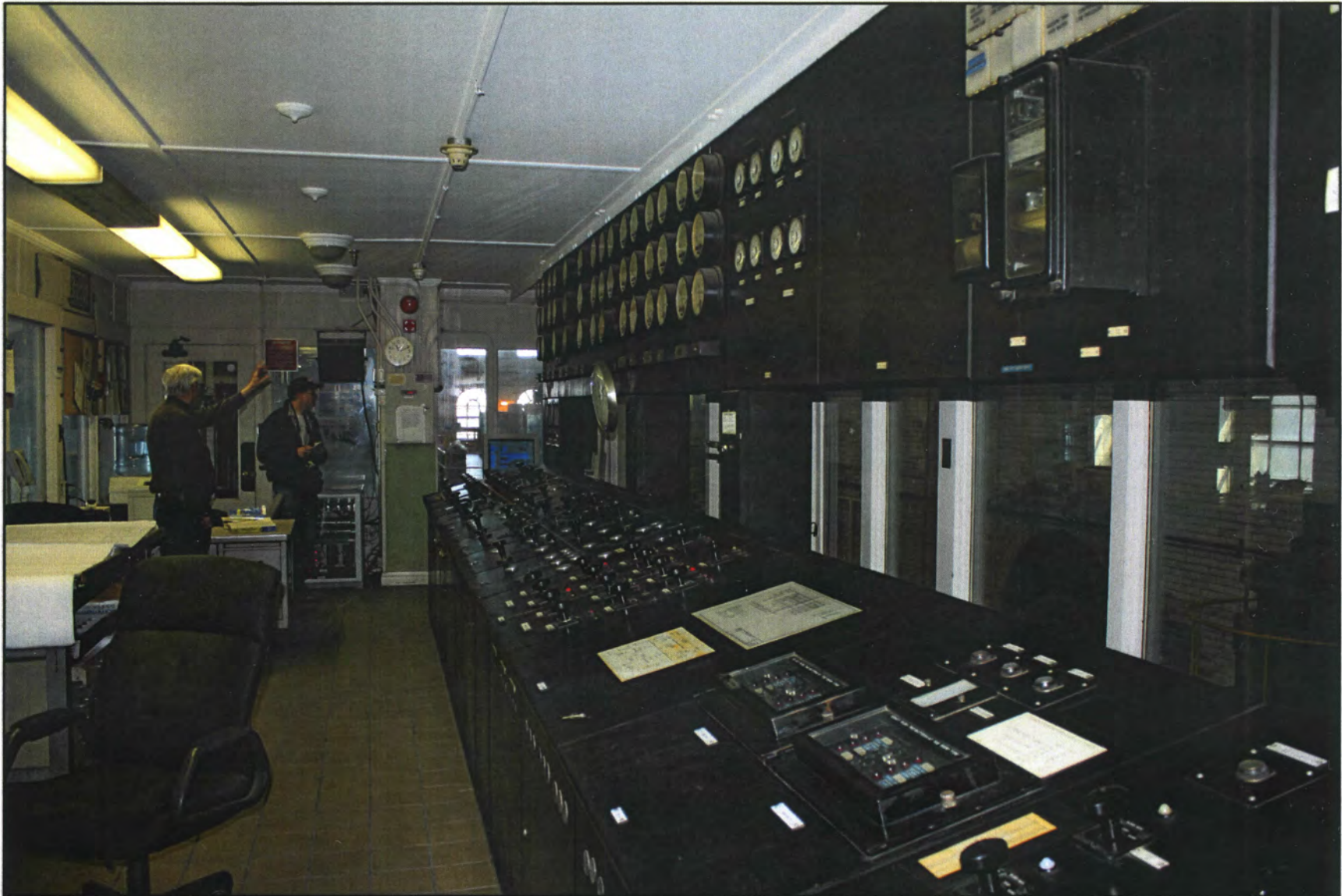
IL_Cook County_Chicago Sanitary and Ship Canal Historic District_0040
