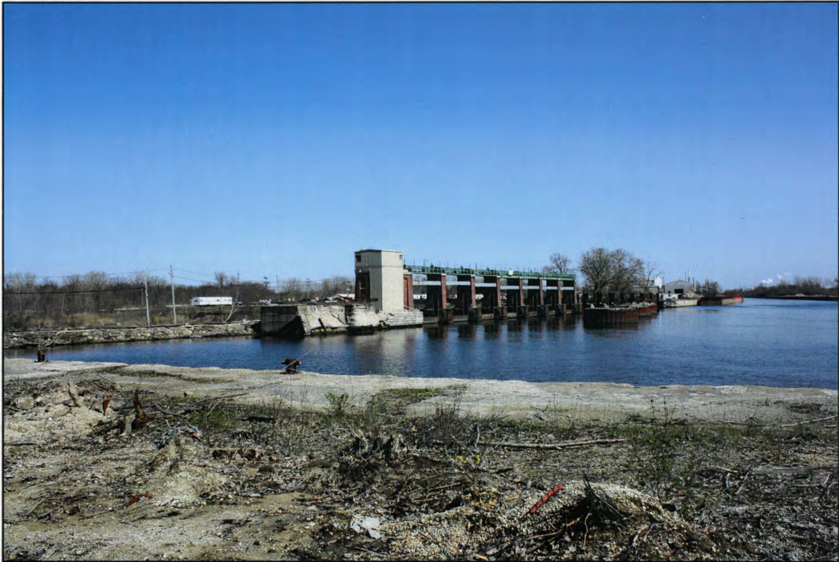
IL_Cook County_Chicago Sanitary and Ship Canal Historic District_0024
