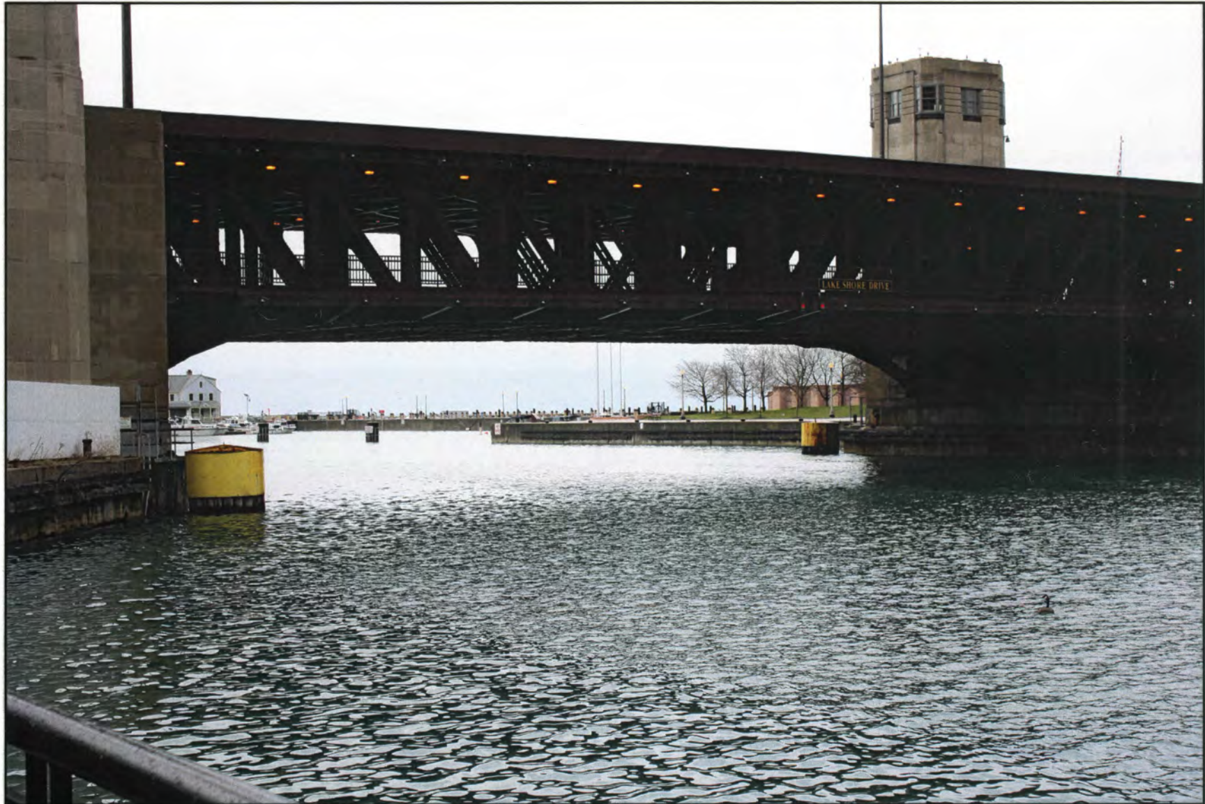
IL_Cook County_Chicago Sanitary and Ship Canal Historic District_0007
