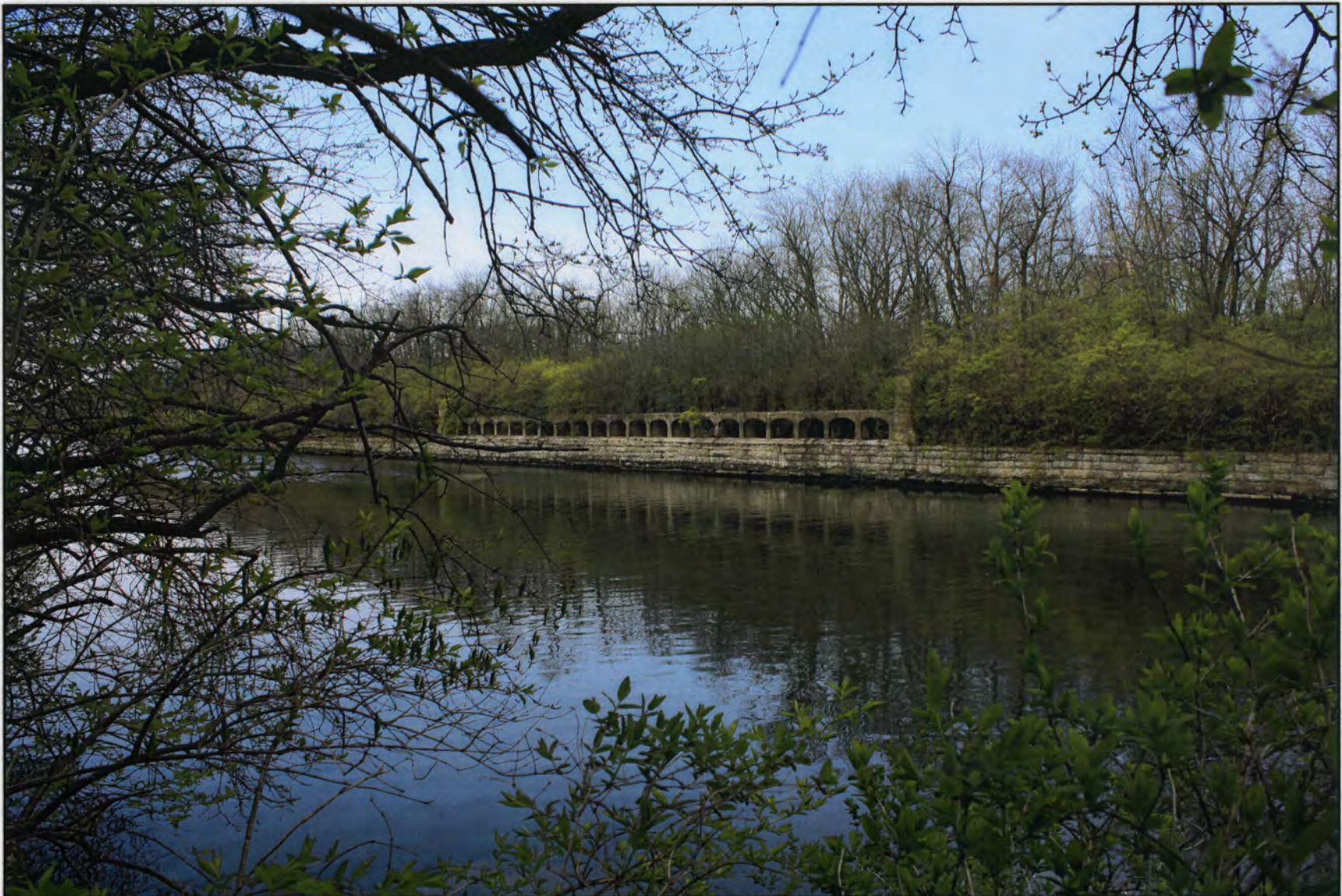
IL_Cook County_Chicago Sanitary and Ship Canal Historic District_0123
