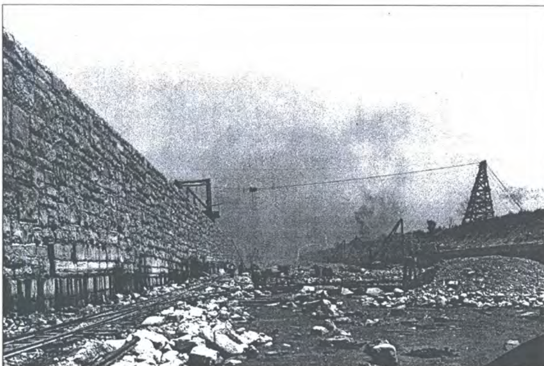
Figure 3: Historic photograph of the rock segment with a cableway in the background, Will County, Illinois. Unknown view. (Unknown photographer, July 7, 1899). Image on file at the U.S. Army Corps of Engineers, Rock Island District.
