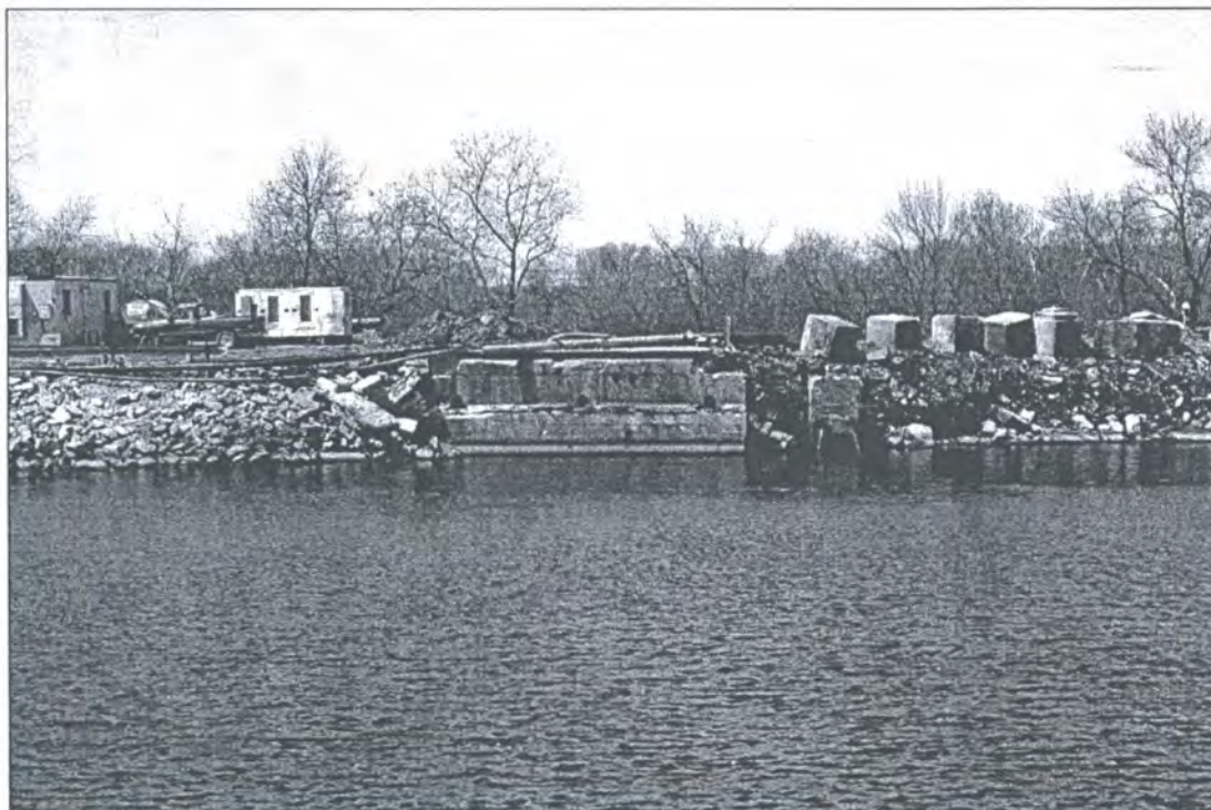
Figure 39: Old Division Street Bridge/16 th Street Bridge abutment on the right descending side of the canal, Will County, Illinois. View to the northwest. (Photographed by Eyan Bond, April 22, 2009). Digital image on file at Bear Creek Archeology, Cresco, Iowa.
