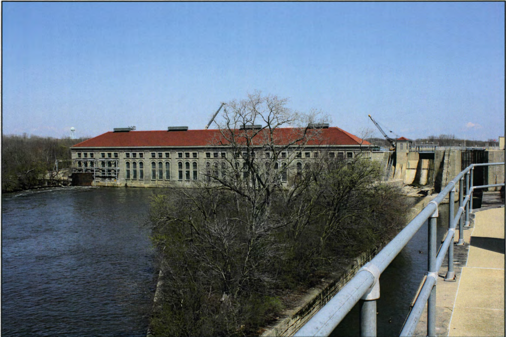
IL_Cook County_Chicago Sanitary and Ship Canal Historic District_0056
