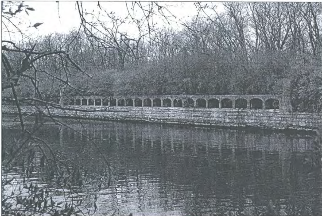
Figure 28: Current condition of the Willow Springs Spillway on the right descending side of the canal, Cook County, Illinois. View to the northwest. (Photographed by Eyan Bond, April 23, 2009). Digital image on file at Bear Creek Archeology, Cresco, Iowa.
