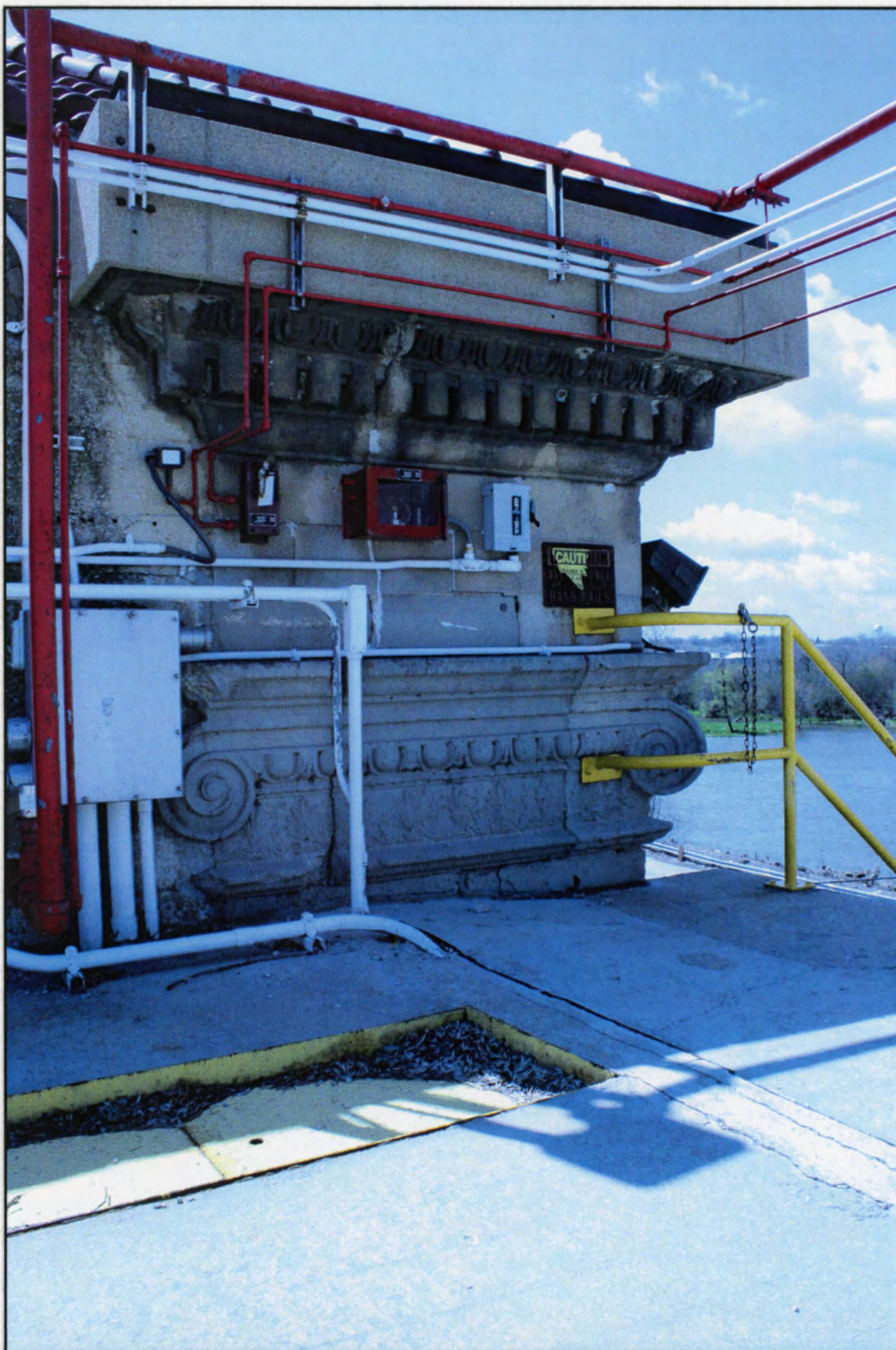
IL_Cook County_Chicago Sanitary and Ship Canal Historic District_0064
