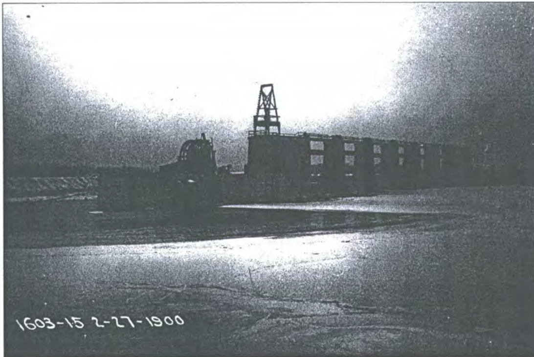
Figure 18: Historic photograph of the Lockport Controlling Works showing the north pier of the bear trap dam and sluice gates, Will County, Illinois. View to the north-northwest. (Unknown photographer, February 27, 1900). Image on file at the U.S. Army Corps of Engineers, Rock Island District.
