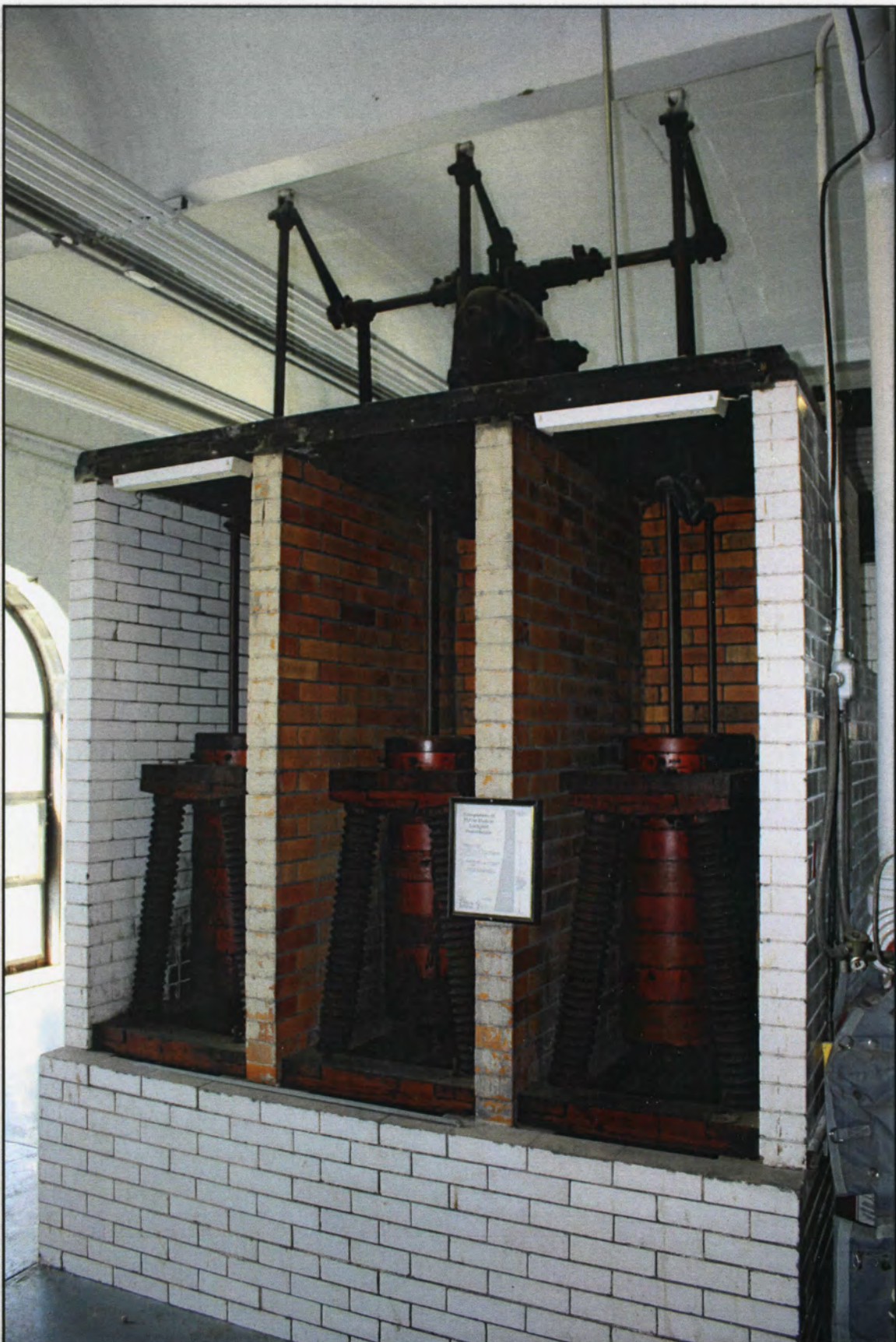
IL_Cook County_Chicago Sanitary and Ship Canal Historic District_0043
