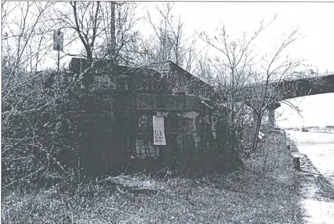
Figure 42: Lemont Street/Stephens Street Bridge abutment on the left descending side of the canal, Cook County, Illinois. View to the southwest. (Photographed by Eyan Bond, April 23, 2009). Digital image on file at Bear Creek Archeology, Cresco, Iowa.
