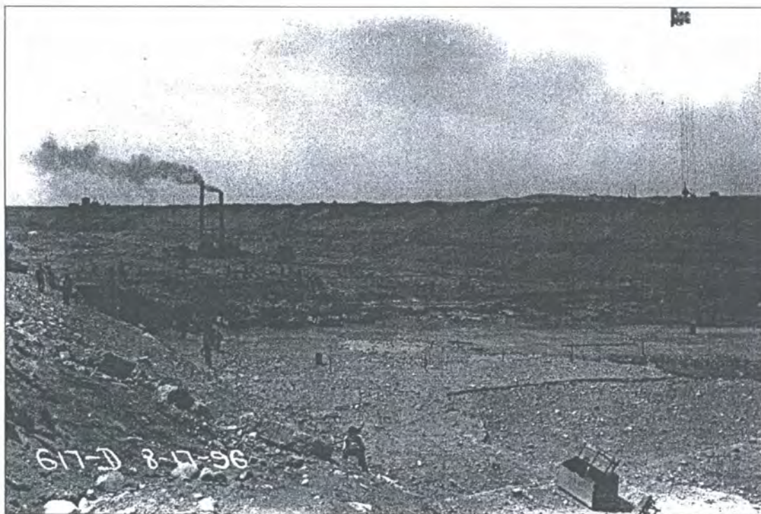
Figure 11: Historic photograph of the earth segment excavation with hoppers being loaded under cableways, Cook County, Illinois. Unknown view. (Unknown photographer, August 17, 1896). Image on file at the U.S. Army Corps of Engineers, Rock Island District.
