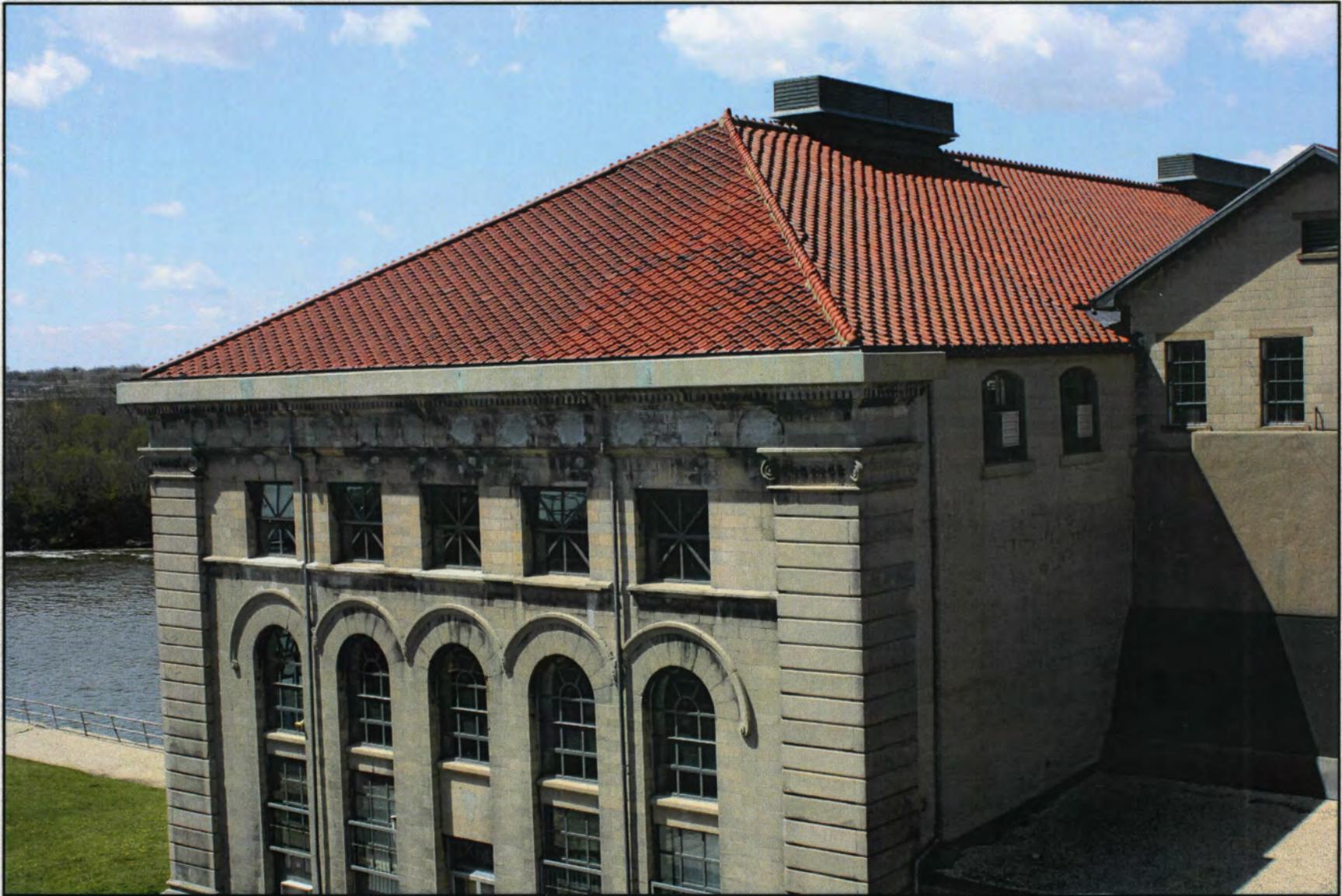
IL_Cook County_Chicago Sanitary and Ship Canal Historic District_0062
