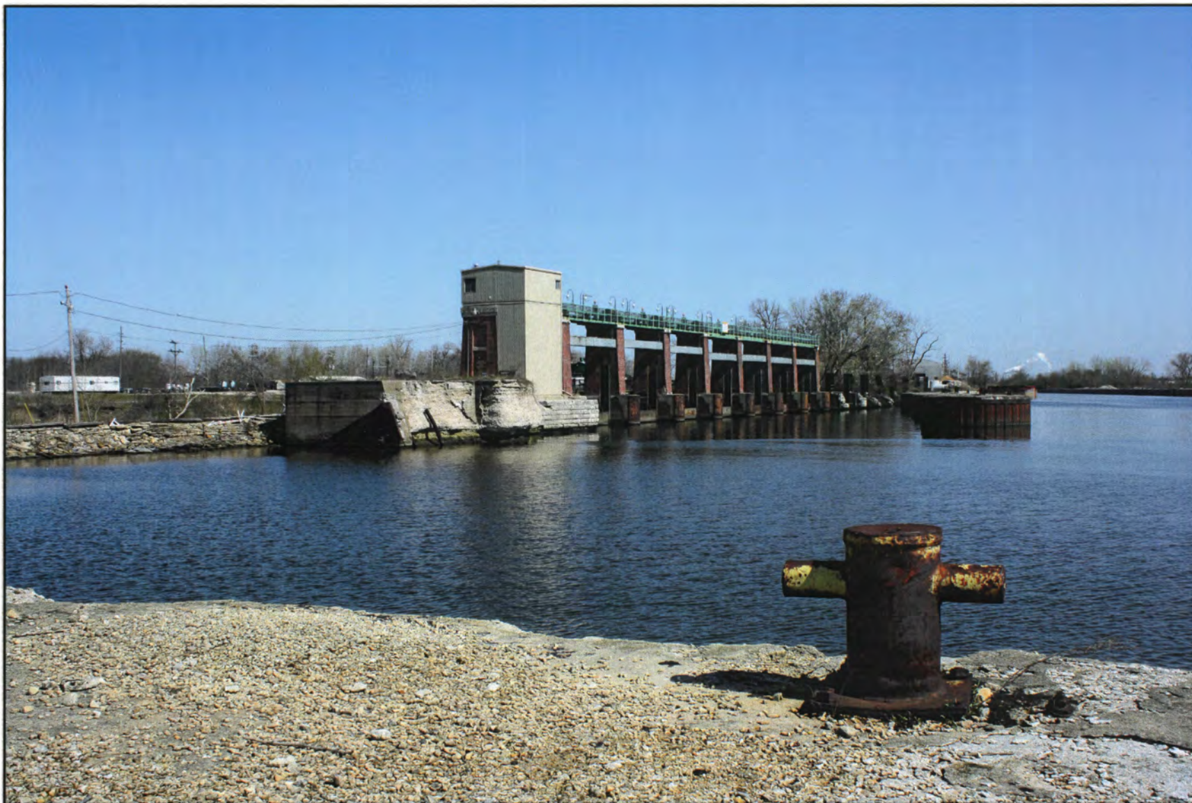
IL_Cook County_Chicago Sanitary and Ship Canal Historic District_0025
