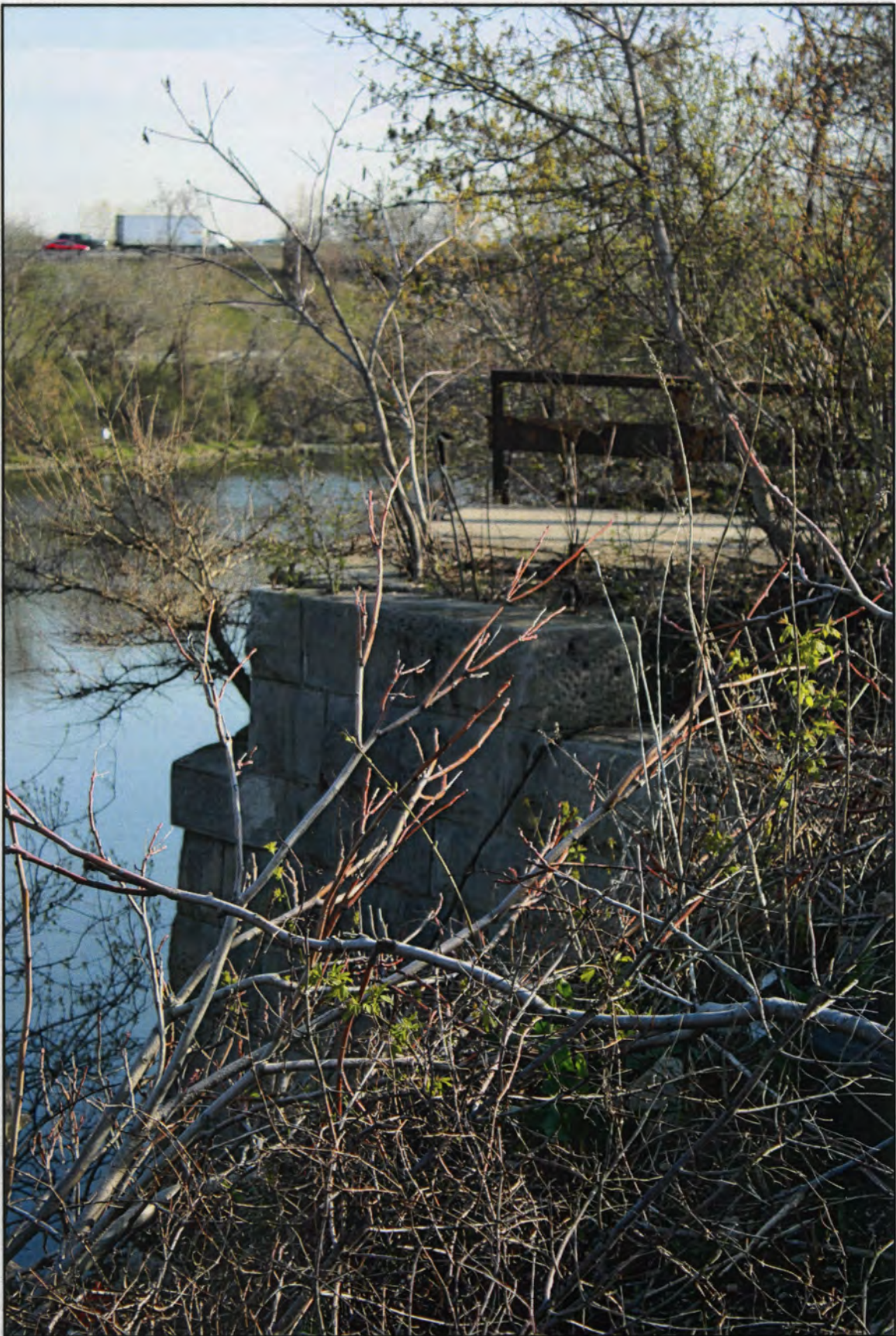
IL_Cook County_Chicago Sanitary and Ship Canal Historic District_0097
