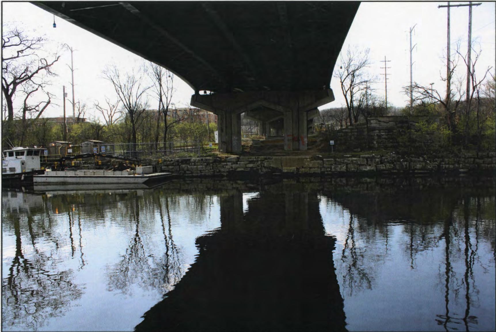
IL_Cook County_Chicago Sanitary and Ship Canal Historic District_0098
