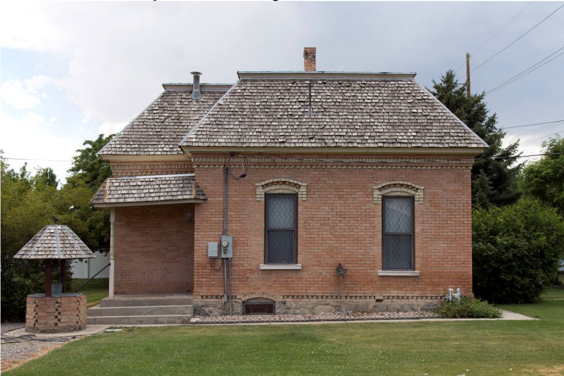
6 of 16. View of East façade. Camera facing west.
