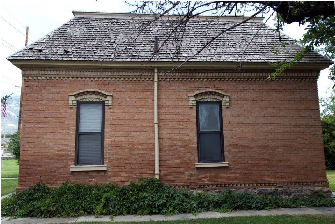
2 of 16. View of West façade. Camera facing east.
