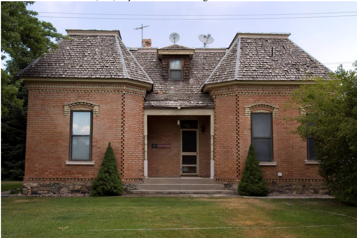
4 of 16. View of South (rear) façade. Camera facing north.
