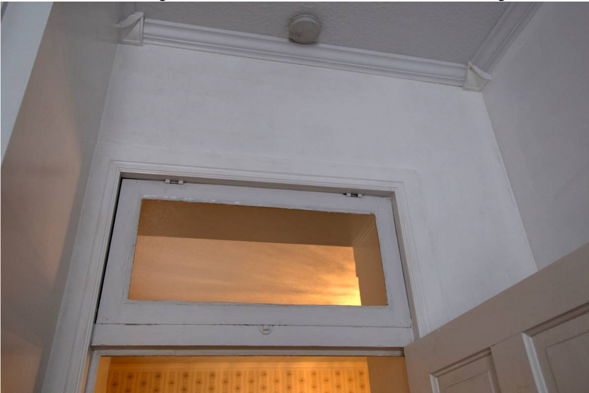
15 of 16. Crown molding and interior transom window detail. Camera facing east.
