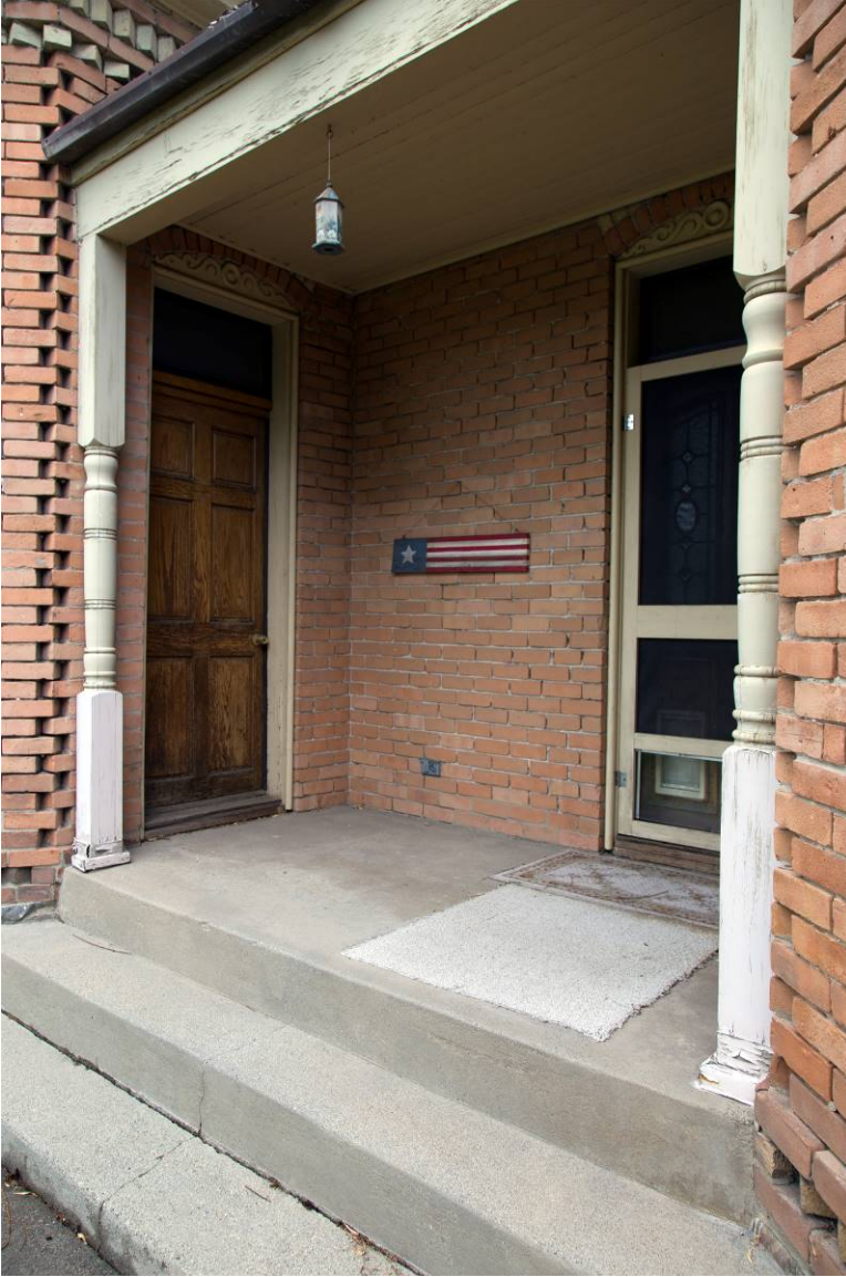
11 of 16. Rear porch detail. Camera facing northwest.
