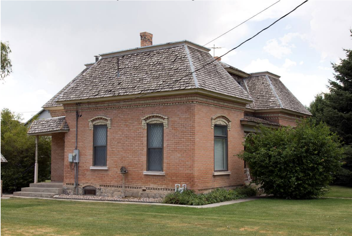
7 of 16. View of Northeast façade. Camera facing southwest.
