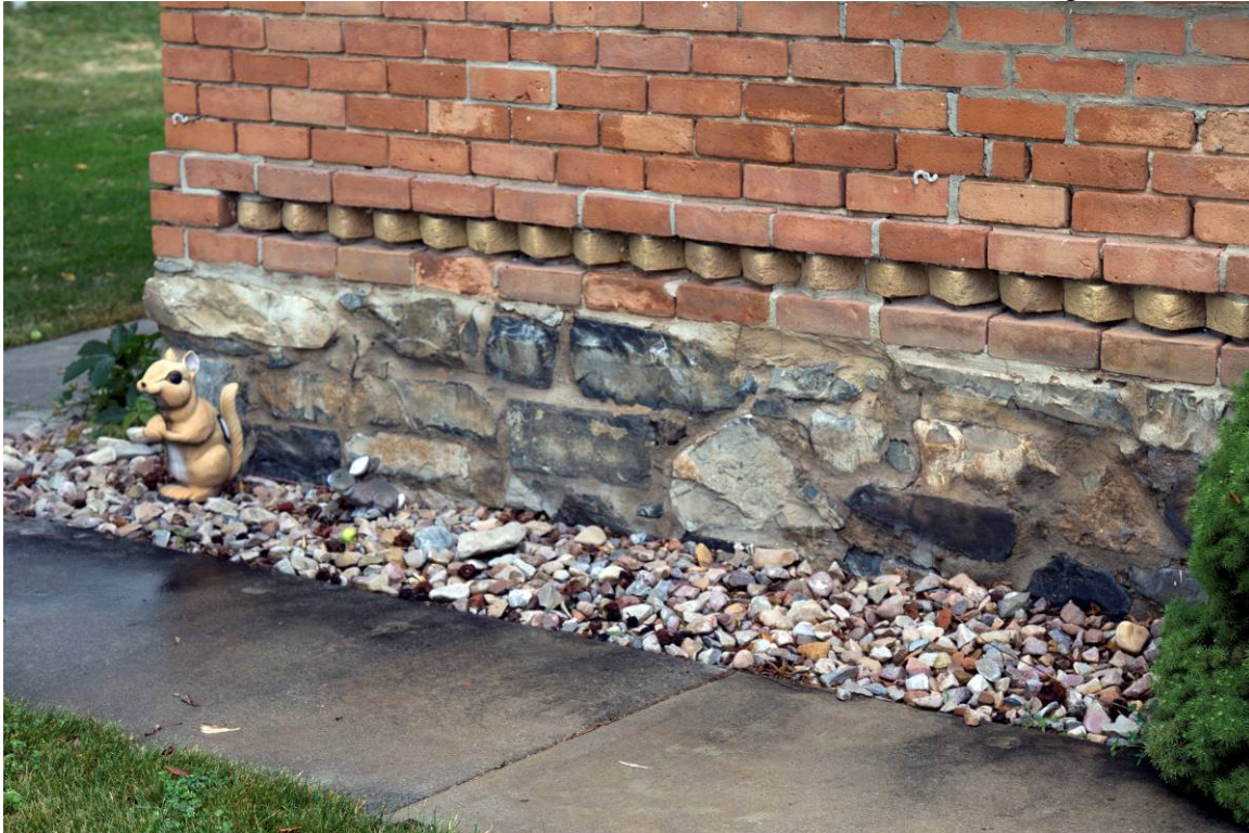
12 of 16. Foundation and lower decorative brick course detail. Camera facing north.
