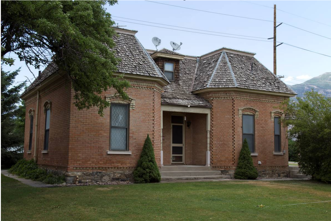
3 of 16. View of Southwest façade. Camera facing northeast.
