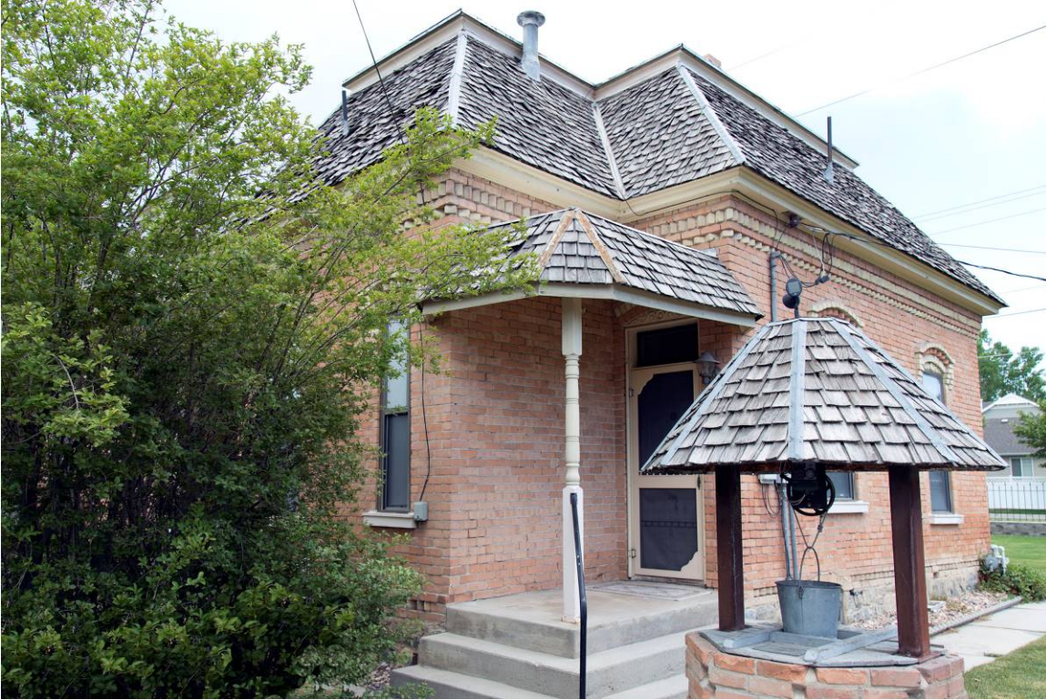
5 of 16. View of Southeast façade. Camera facing northwest.
