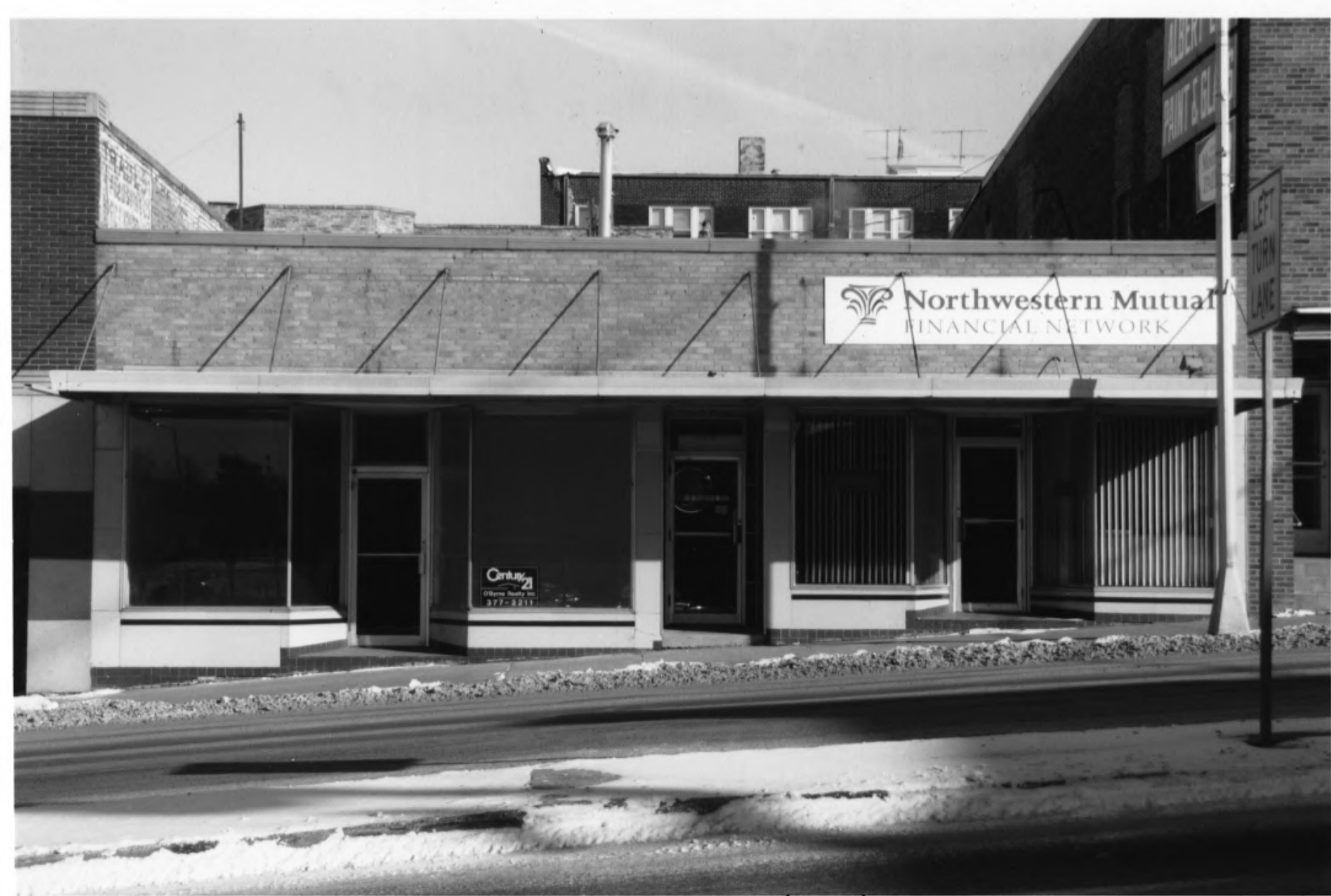
#36 Commercial Building (Contributing) Albert Lea Commercial Historic District Freeborn Co., Mn 014555-18
