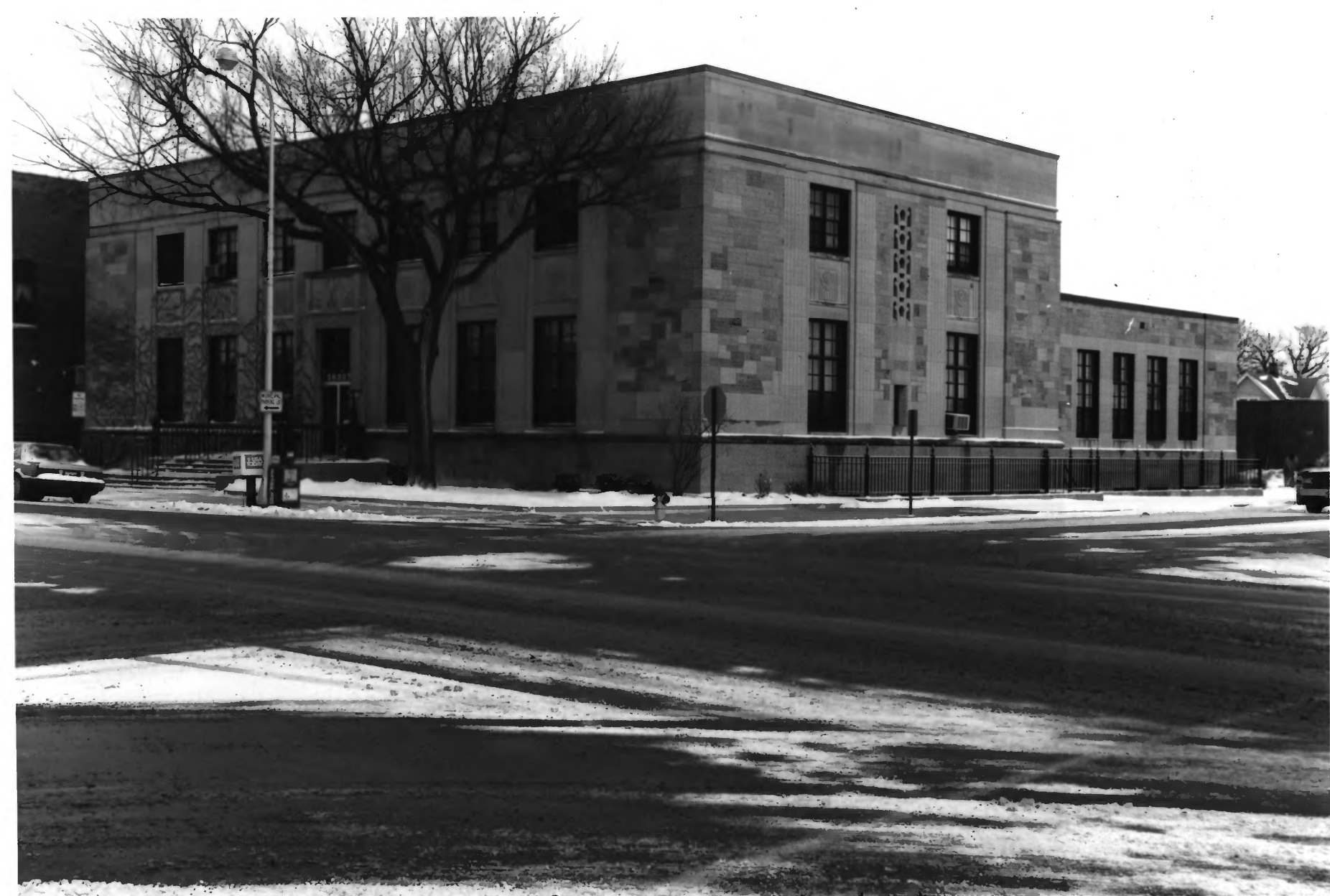
#44 United States Post Office (Contributing) Albert Lea Commercial Historic District Freeborn Co., MN 014557-6A
