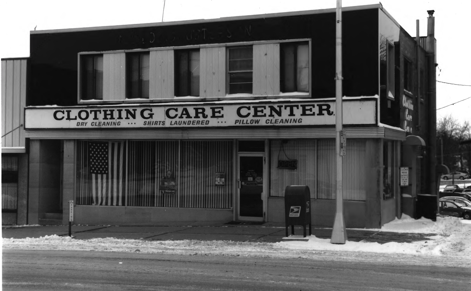
#48 Commercial Building (contributing) Albert Lea Commercial Historic District Freeborn Co., MN 014556-12
