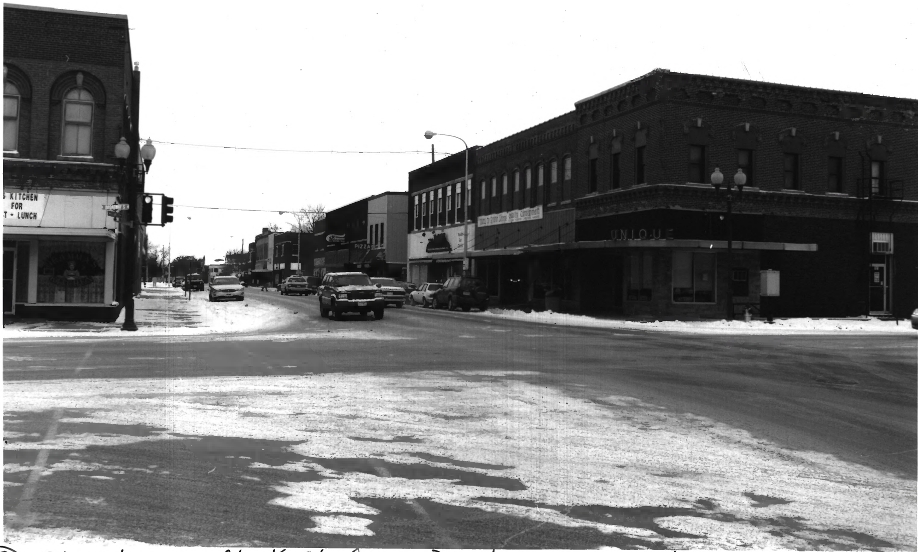
② Streetscape, Clark St. from Broadway Ave. Looking W Albert Lea Commercial Historic District Freeborn Co., Mn 014556-23
