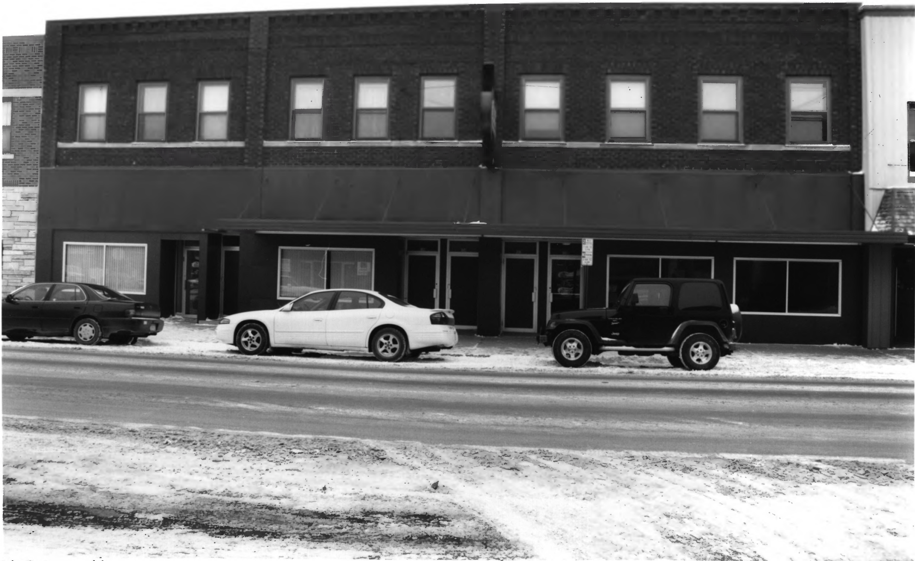
#21 + #22 Commercial Building (Contributing) Albert Lea Commercial Historic District Freeborn Co., MN 014556-4
