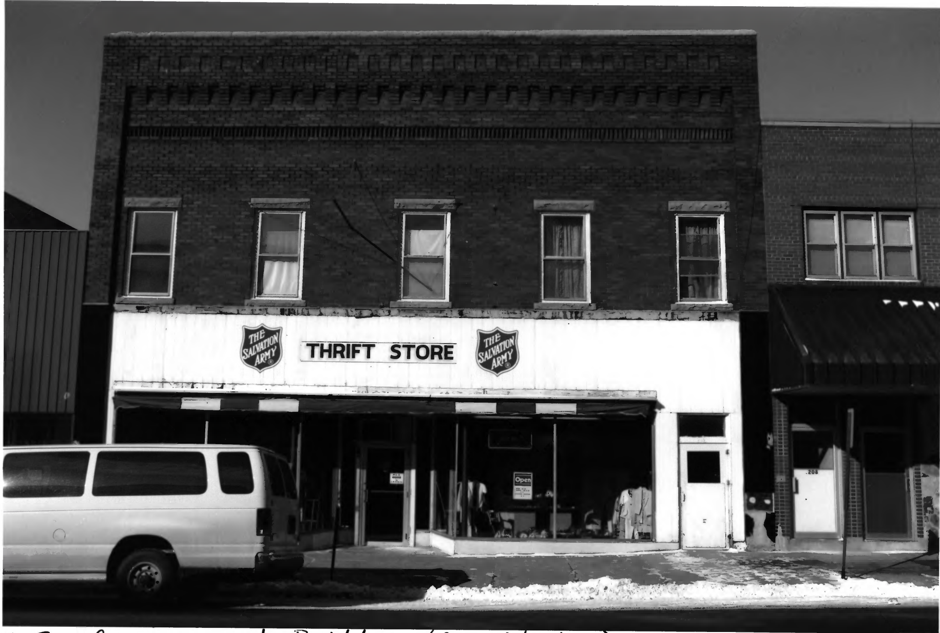
#55 Commercial Building (Contributing) Albert Lea Commercial Historic District Freeborn Co., MN 014555-24
