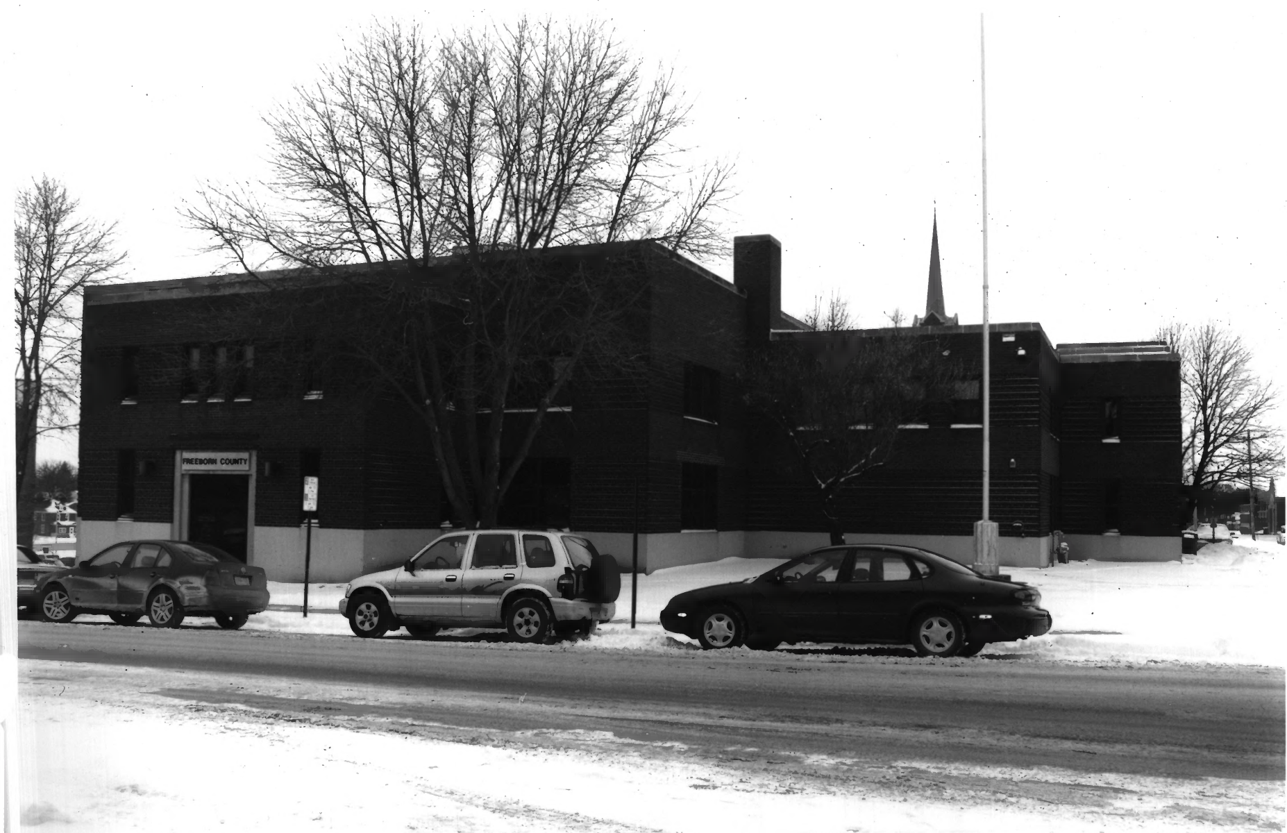
#46 Minnesota National Guard Armory (Contributing) Albert Lea Commercial Historic District Freeborn Co., MN 014556-11
