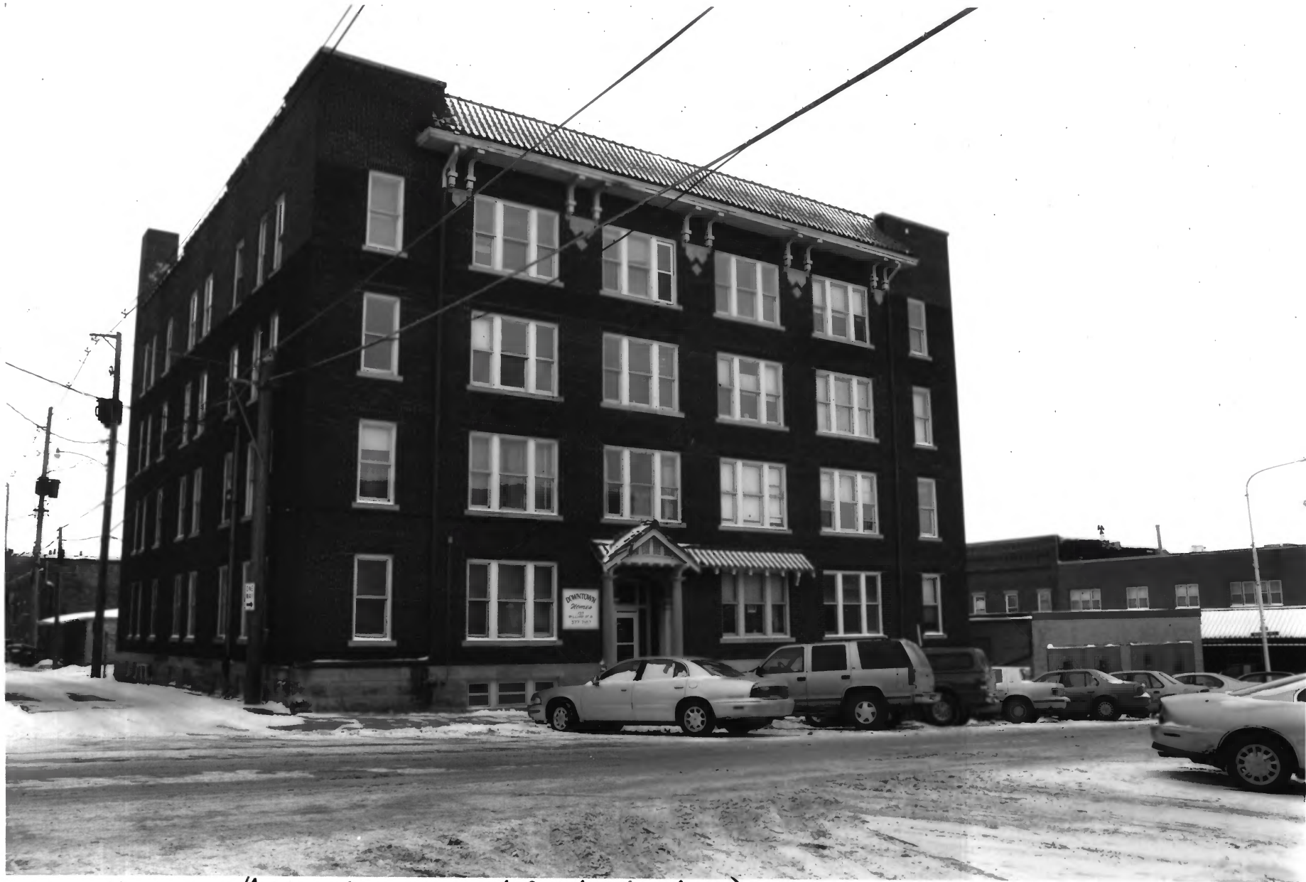
#64 Hellie Apartments (Contributing) Albert Lea Commercial Historic District Freeborn Co., Mn 014556-21
