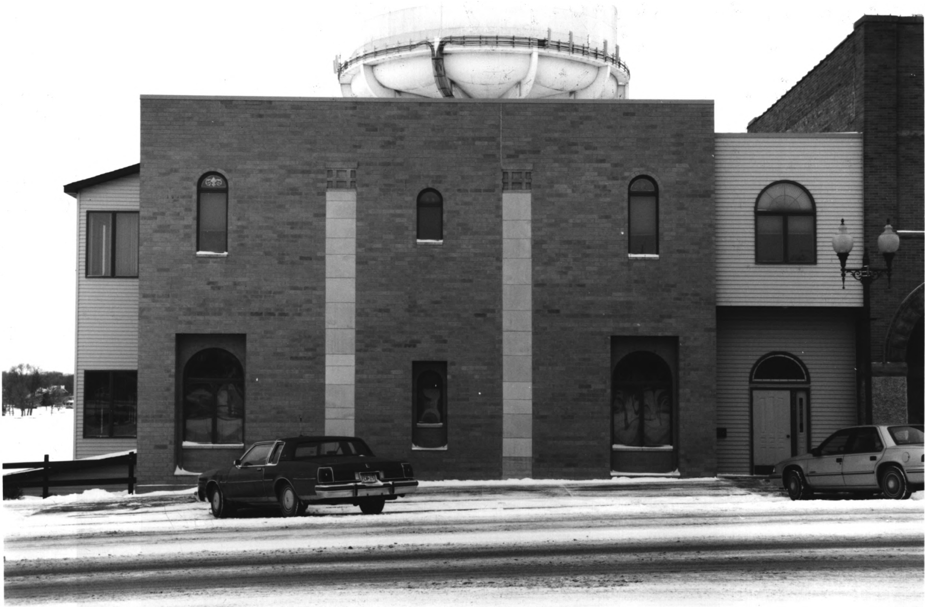
⑤ Johnson Laundry Company Building - proposed for exclusion from The District, photo taken after remodeling.
