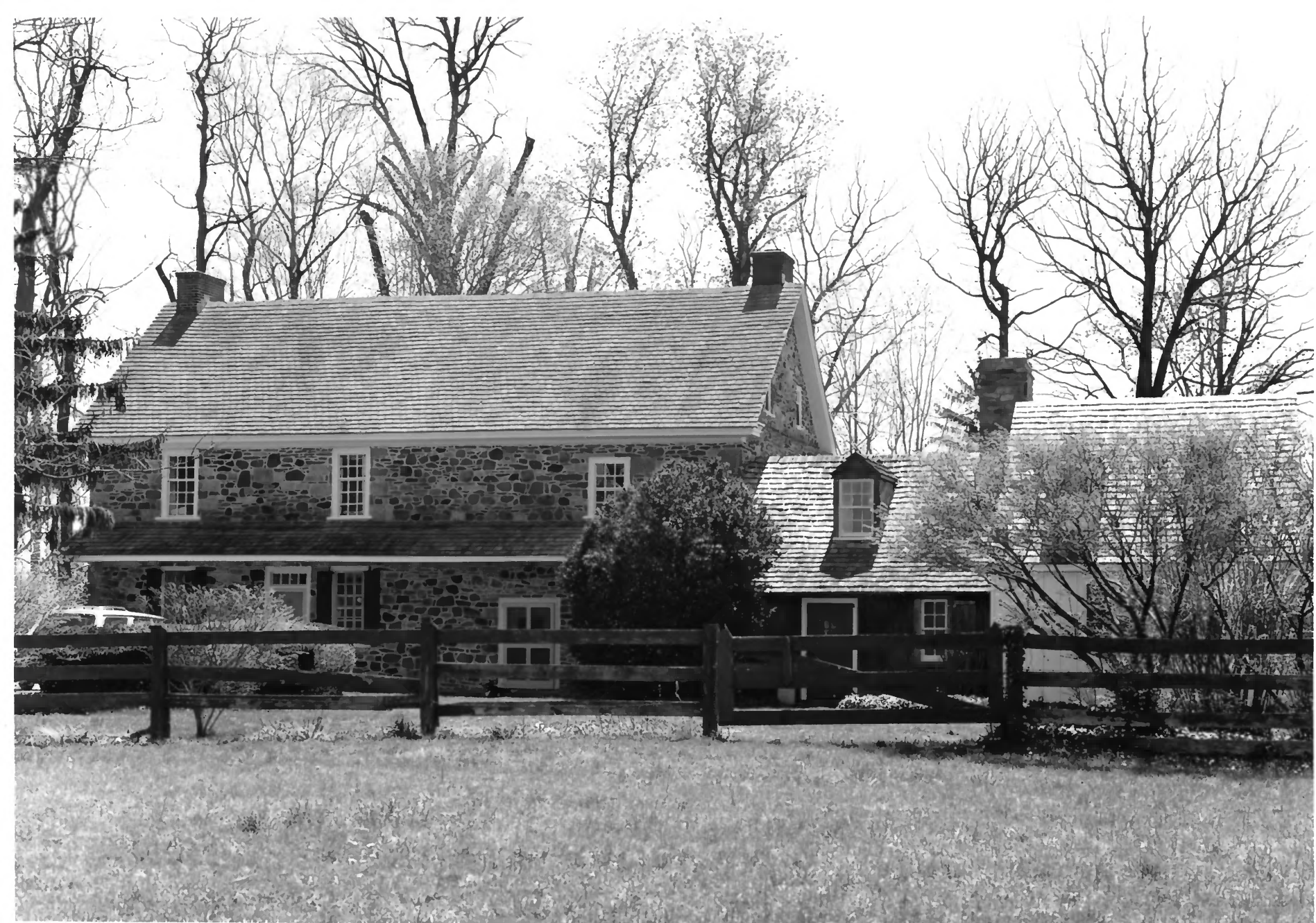
Humphry Marshall House, West Chester, Pa Main house, kitchen, and addition
