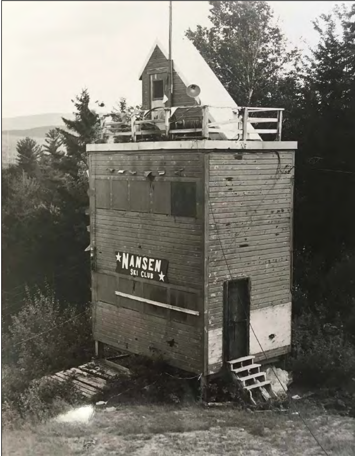
Figure 6. 1977 view of the Judge's Hut (built 1963), west elevation and south side (MacDonald 1977).
