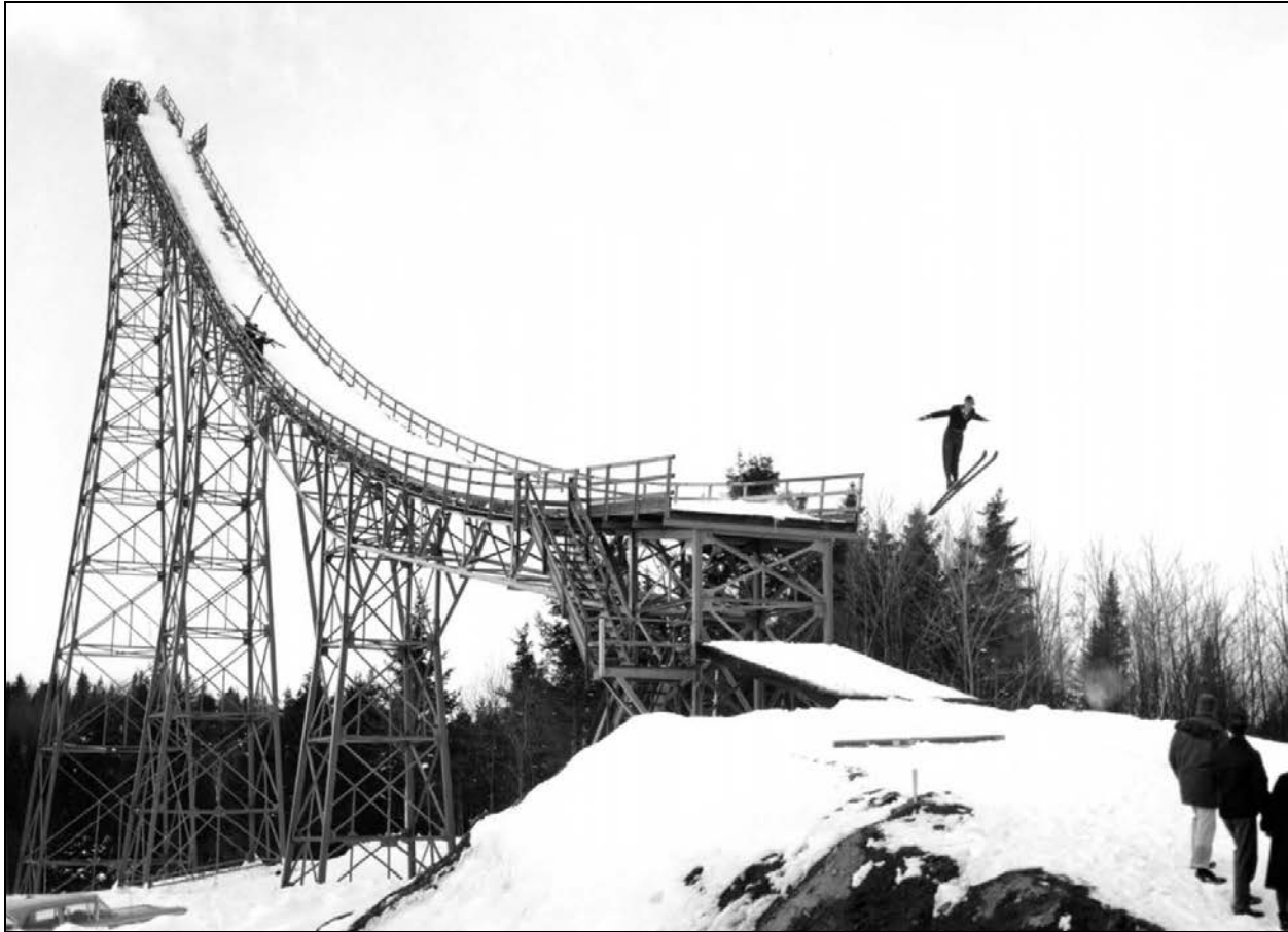
Figure 14. Nansen Ski Jump shortly after the 1963 rehabilitation. Changes to the inrun tower consisted of adding approximately 10 feet to the top of the jump to accommodate three new starting points and modifications to the takeoff, eliminating the wooden trestle structure that had been there previously (McPhaul 2018:7).
