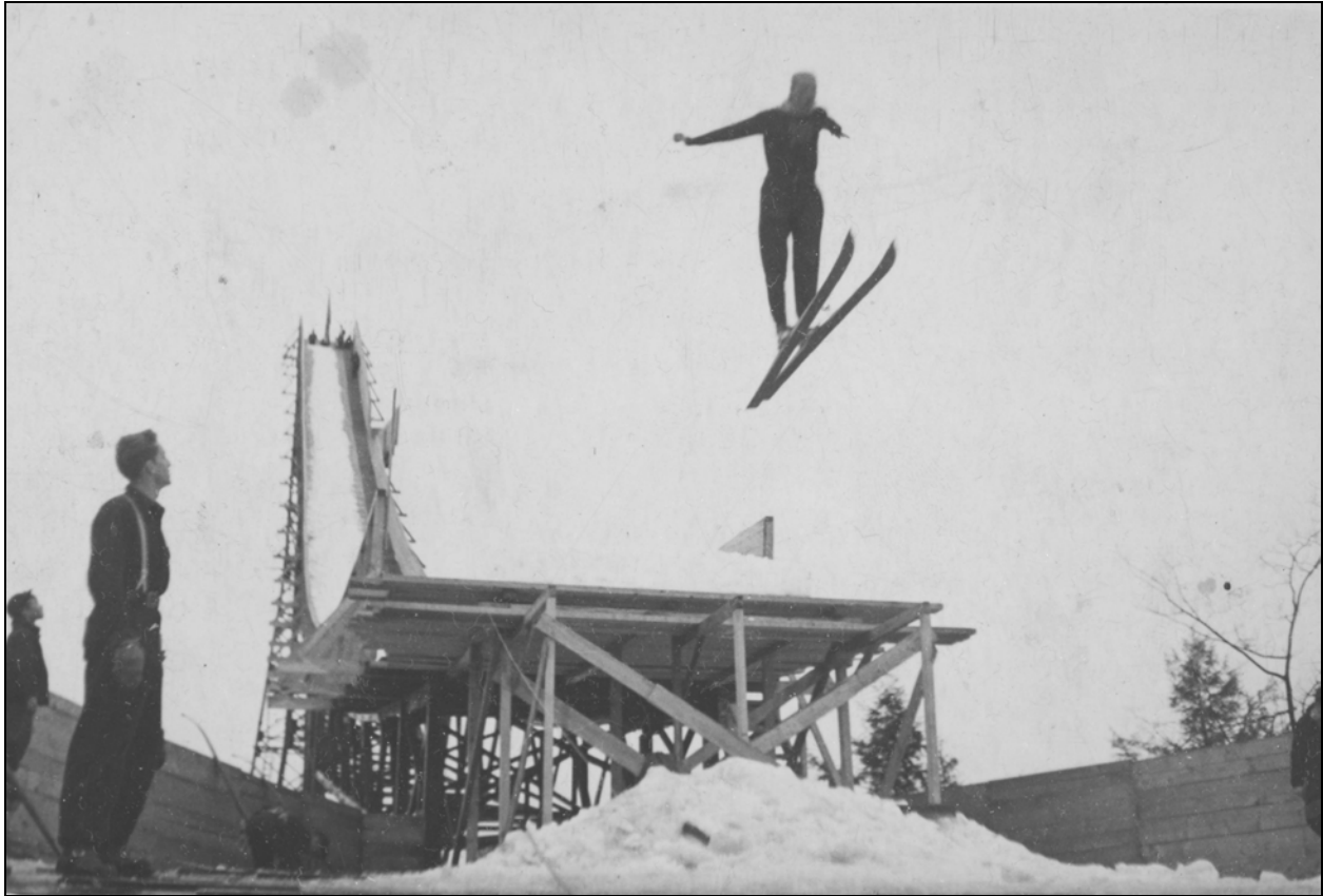
Figure 4. 1938 view showing wood frame take-off extension that was later removed (Dartmouth Digital Library).
