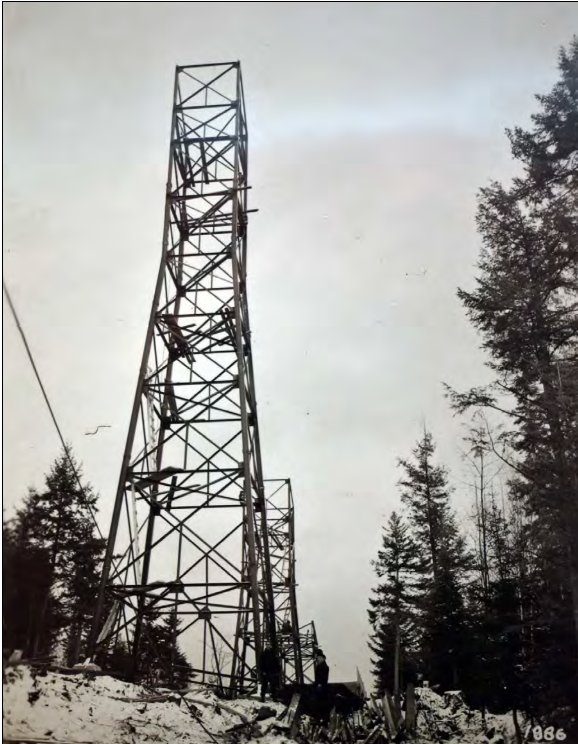
Figure 12. Steel inrun towers fabricated by the Hussey Manufacturing Company and erected by the NYA in 1937 (Berlin & Coos County Historical Society).
