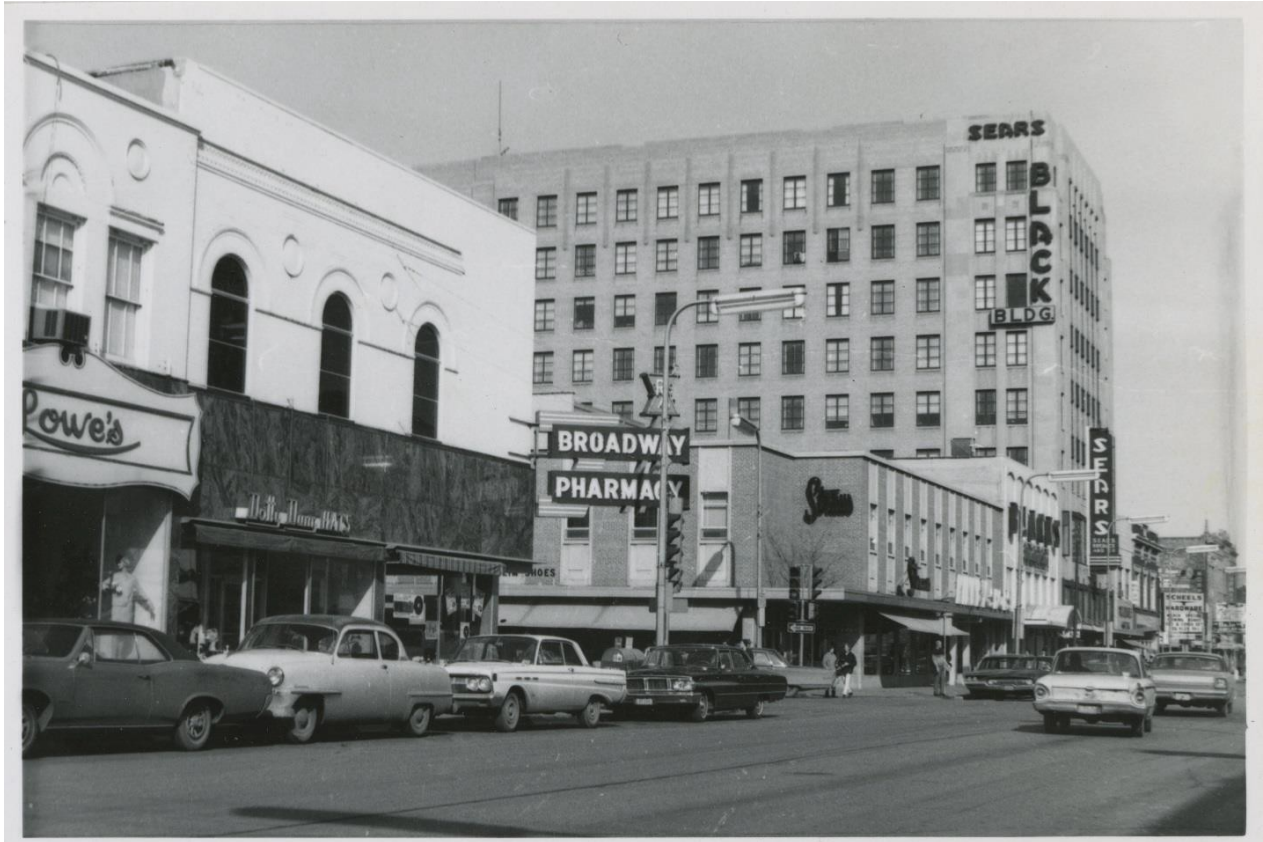
Name of Property: Black Building City or Vicinity: Fargo County: Cass State: ND Photographer: Unknown Date Photographed: 1968 View: North, south elevation Photograph 2 of 14: ND_Cass County_Black Building_0002.tif
