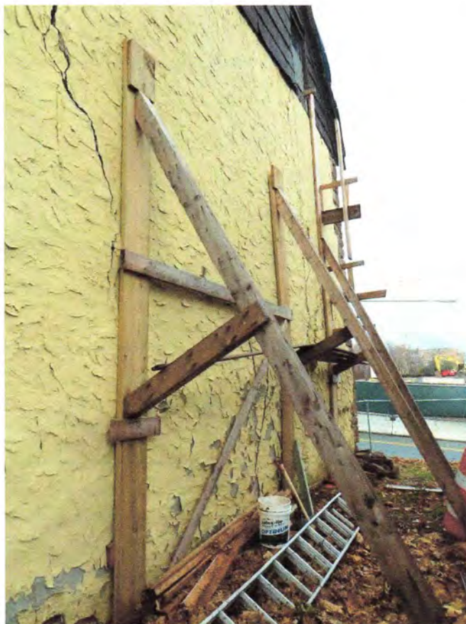
Photo 03 – General view of east side of house showing bracing and cracks in masonry. The concrete masonry unit (CMU) infill and concrete bond beam installed at the north end of this wall has been covered with stucco.
