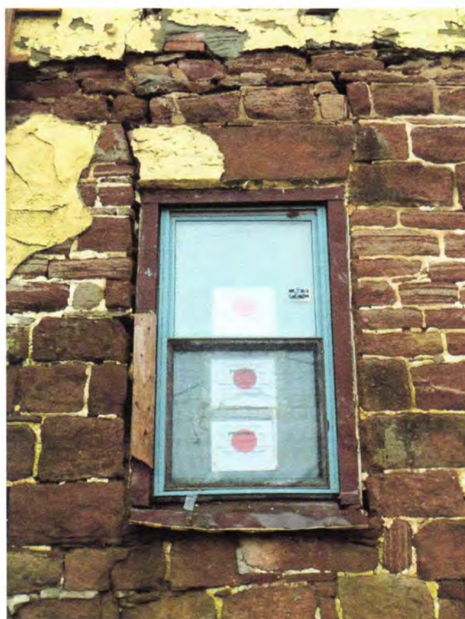
Photo 08 – Typical single-piece “jack arch” lintel in the exterior leaf of stone. Where the wall has been rebuilt, the arches have not been replaced. Temporary 2x lintels were placed in the wall until the stones can be replaced.
