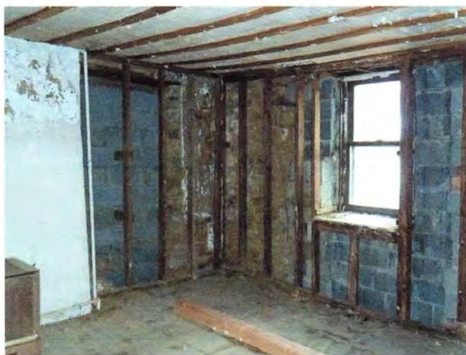
Photo 07 – General view of southeast corner of house at interior showing existing “liner wall” along south and east elevations and the remains of the original masonry butted to the CMU built following local collapses of the original masonry.
