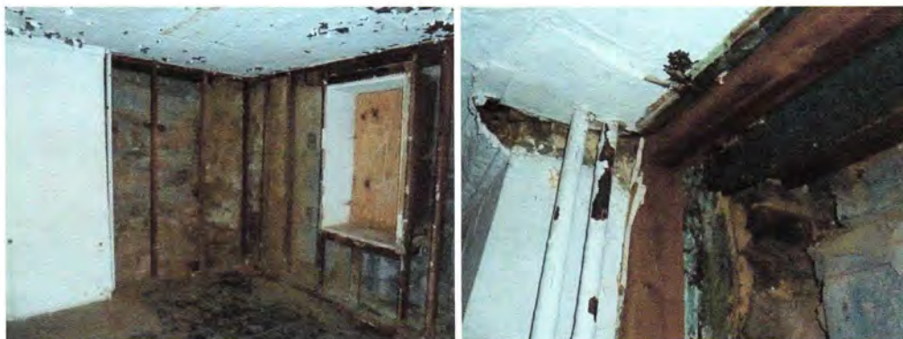
38. Southeast corner (brownstone) with concrete block infill at East & South walls 39. Interior finishes & trim, inner wood-framed wall, finishes & trim on interior of masonry wall, brownstone & concrete block infill at East wall, South (right) of chimney in Figure 38
