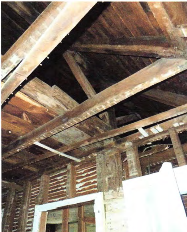
Photo 16 – General view of “truss” framing over post at mid-span (east to west). Post appears to bear on floor, not on beam in floor.
