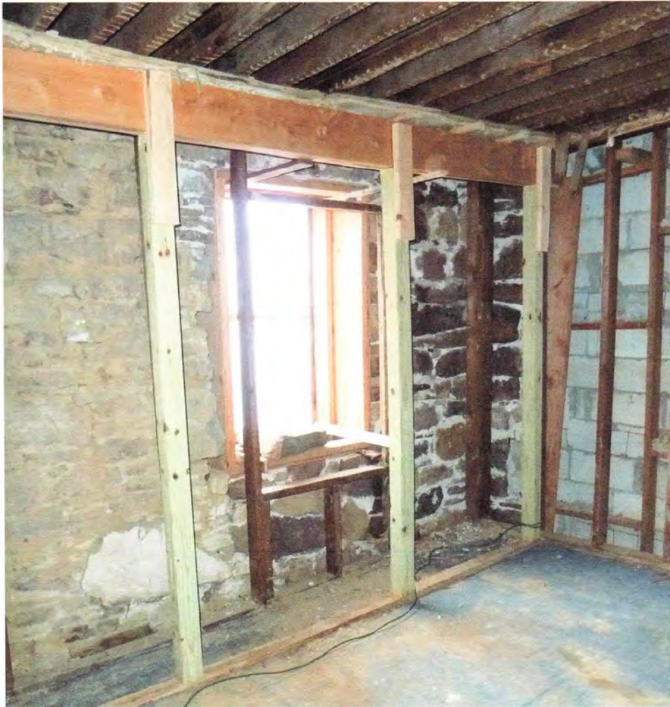
43. Second Floor, Northeast corner with original construction West (left) of the window, reconstructed brownstone masonry wall to the East (right) of the window, and concrete block construction on the East Wall (far right)
