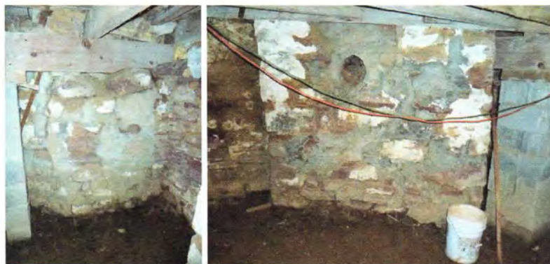
30. Back of triangular chimney mass, with joist cut to accommodate masonry
