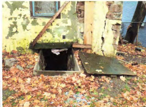
12. Lower portion of bracing and masonry separation at Southeast corner
