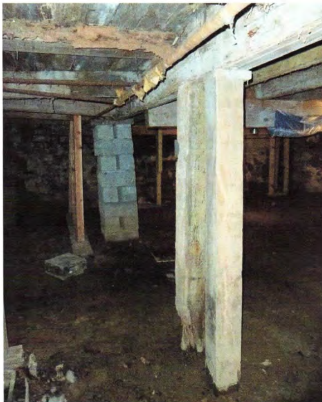
Photo 06 – General view of first floor framing and the girders, posts, and piers that support the first floor framing. Most, if not all of the first floor framing is severely deteriorated.
