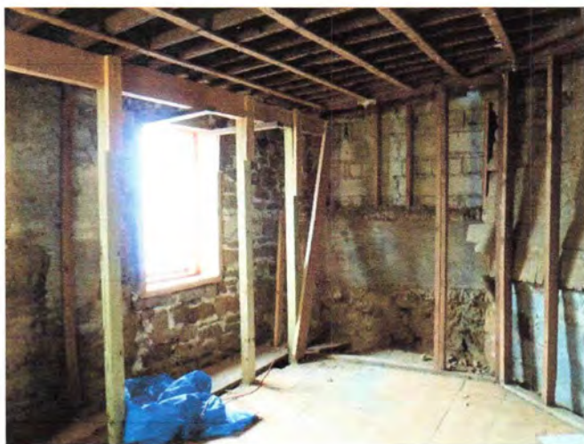
Photo 09 – General view of northeast corner from the interior showing rebuilt corner and the CMU and concrete bond beam at the south wall. The masonry at the firebox has partially collapsed.
