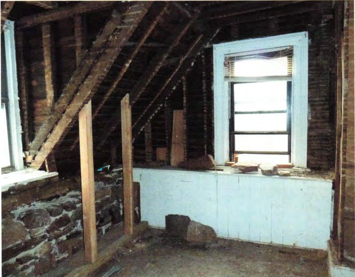
53. Attic, Northeast corner with reconstructed brownstone masonry wall below the dormer window (North wall)
