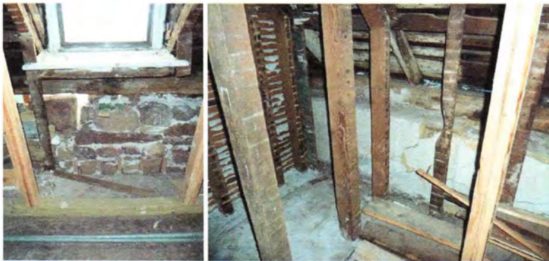
54. Reconstructed brownstone wall beneath Eastern dormer window (North wall) 55. Original plaster-finished masonry knee wall (North wall)
