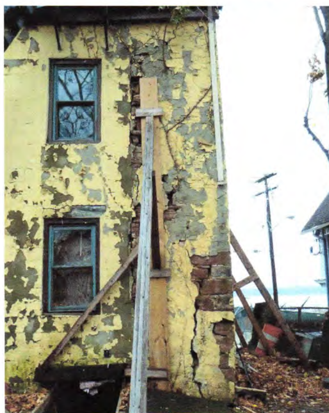
Photo 04 – General view of southeast corner of house showing shoring at east and south walls, as well as the large crack that has developed. The joint between the original masonry and the CMU at the south wall is along the right or east jamb of the windows.
