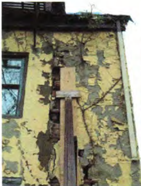
11. Upper portion of bracing
