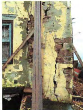
12. Lower portion of bracing and masonry separation at Southeast corner
