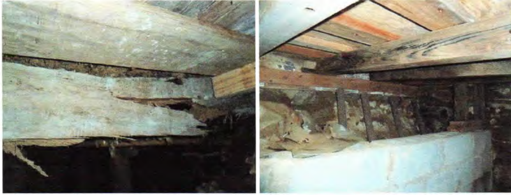
25. Failing First Floor joist at West wall of Cellar
