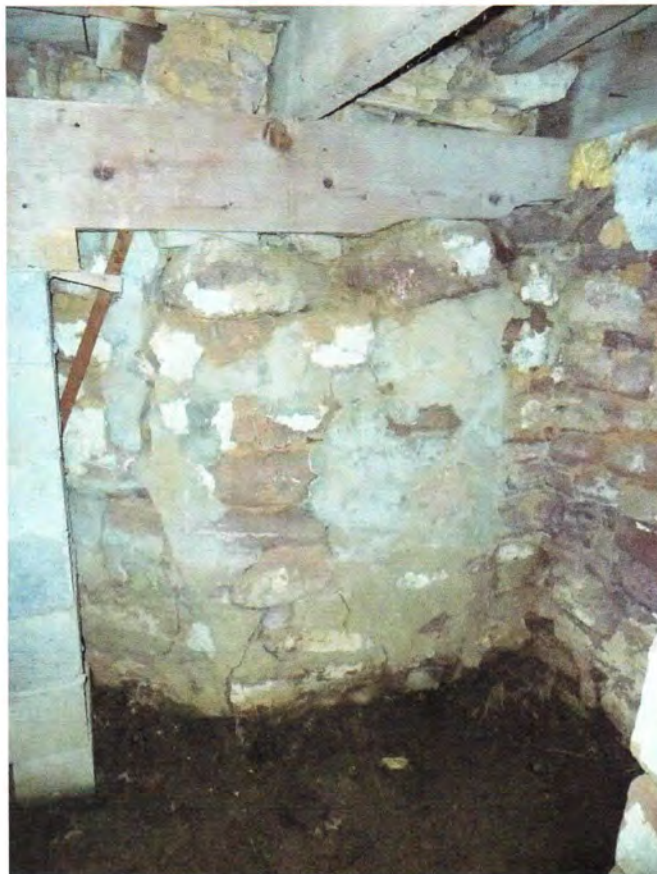
Photo 05 – Bulge at the northwest corner (west wall) of the foundation. There is a door opening to the left of the bulged section of wall that has been filled with masonry.
