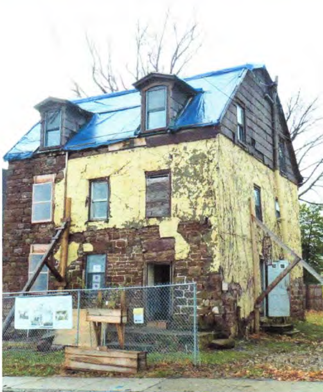
Photo 02 – General view of northwest corner of house showing shoring at west and north walls. There is an open joint / crack in the north wall, just west of the entry door. The masonry wall is leaning / bulged at the brace on the west wall.
