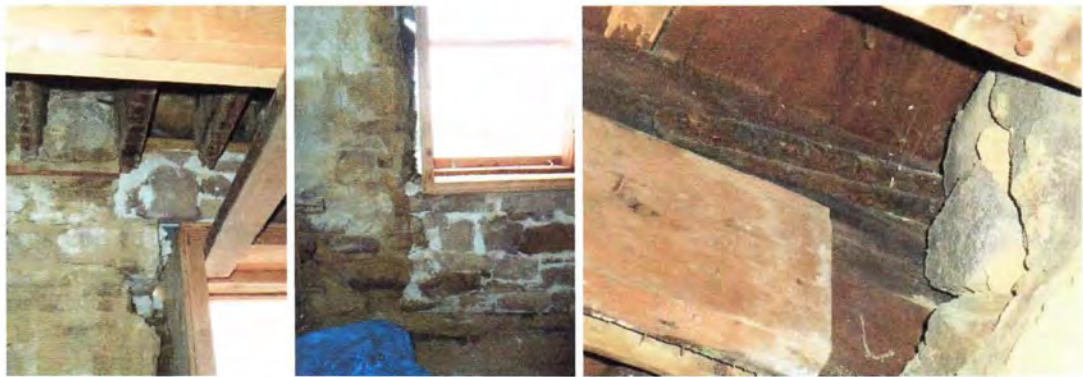
33. Joint between existing and reconstructed North wall at East window head 34. Joint between existing and reconstructed North wall below East window 35. Tie at Second floor joist level
