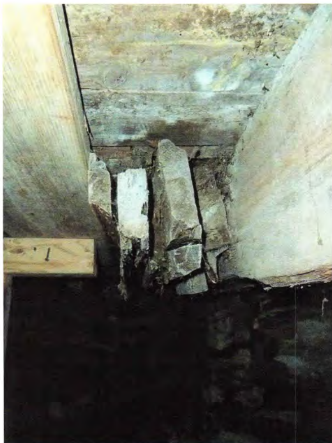
Photo 11 – Typical condition of first floor framing. Pressure-treated material (left in image) has been installed to shore both the joist and the flooring. The flooring is shown supported in this image. See Photo 06 for shoring at joists, in background.
