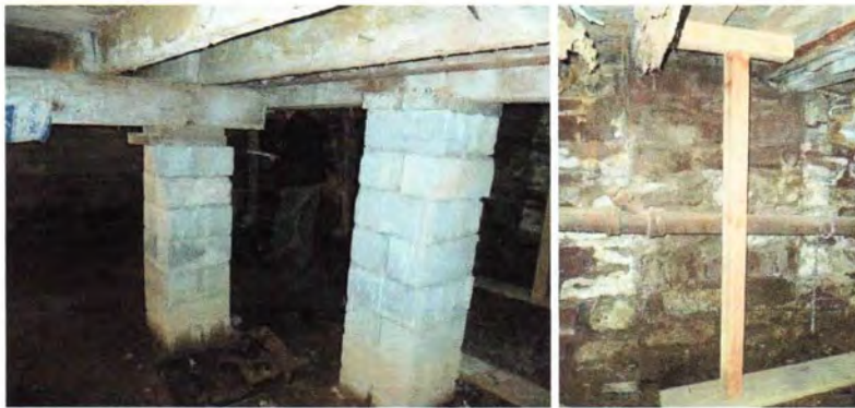
23. Concrete masonry piers, looking Northwest from Cellar entry 24. Outline of masonry infill of previous opening at West wall
