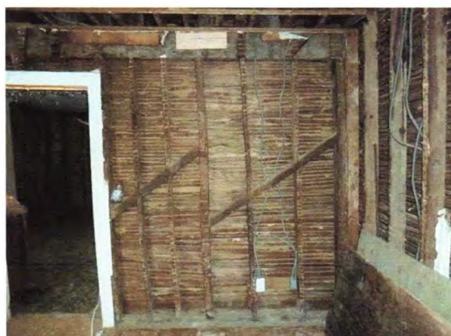
Photo 12 – Bearing partition between north and south rooms at the first floor. Once vertical studs and square door opening are now skewed to the east.
