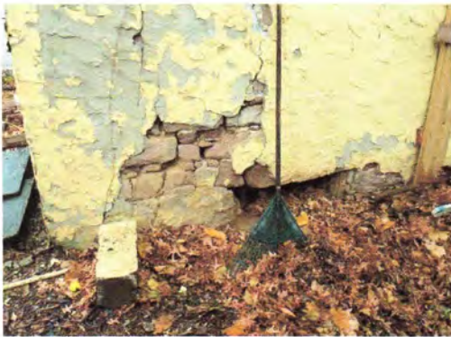
15. Failing plaster and masonry at Southeast corner
