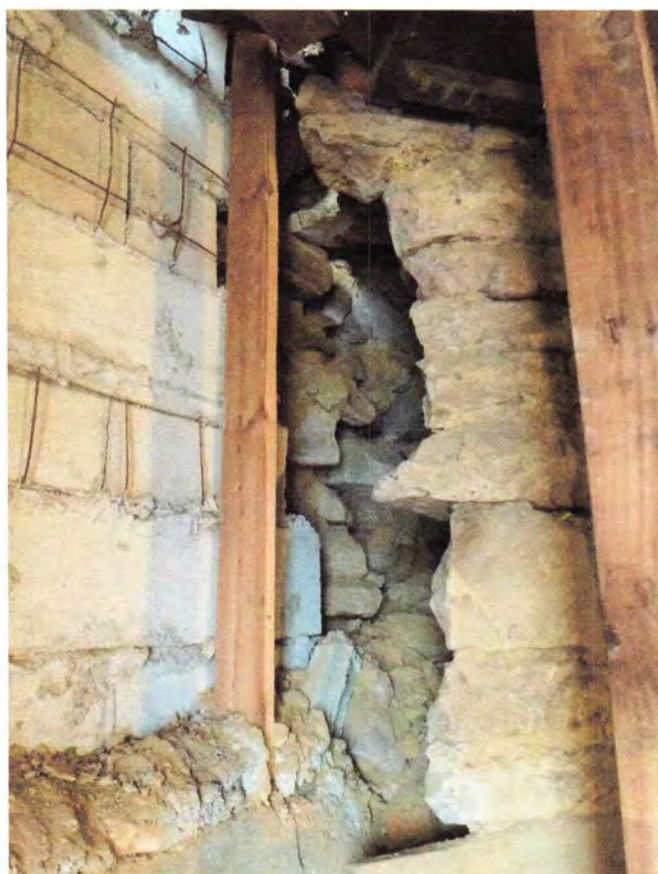
Photo 10 – Separation between the exterior wall (left in image) and the chimney mass is evident at the first floor, north room.
