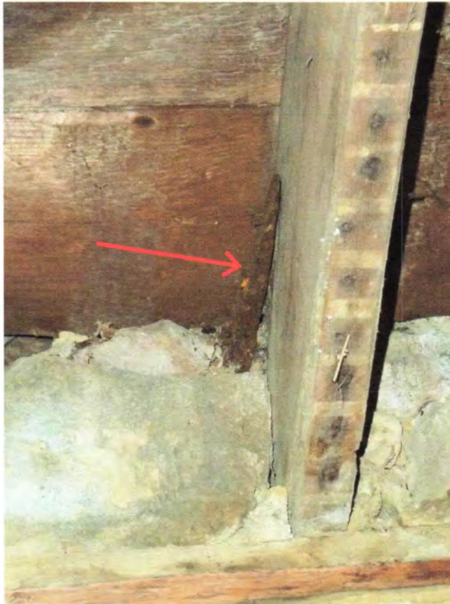
Photo 13 – Close-up view of interior leg of anchors at facades (arrow).
