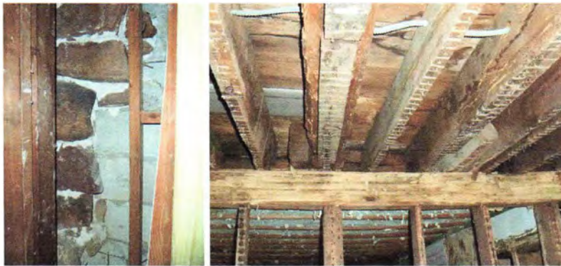
44. Joint between brownstone & concrete block construction at East wall
