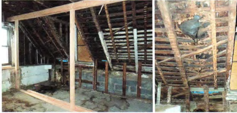
58. Deteriorated roof and dormer framing & concrete block knee wall at Southeast corner
