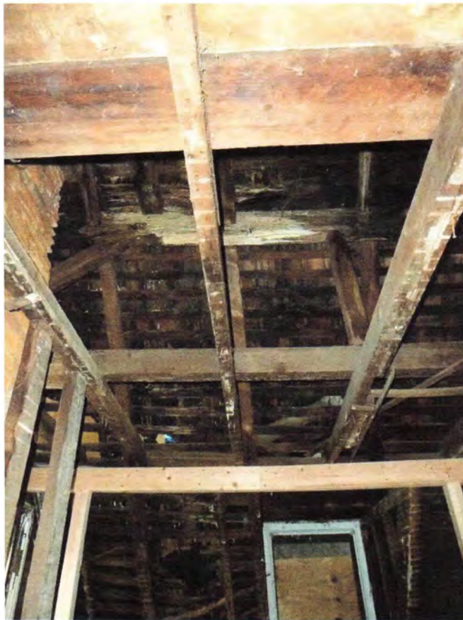
Photo 15 – General view of roof framing, looking south at east end of south slope of roof. Water damaged “upper chord” of “truss” is visible at the center of the image.
