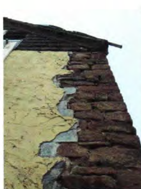
21. Bulging (stuccoed) lower East wall and rebuilt corner
