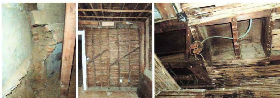
40. Failing brick structure at interior chimney, North room 41. Interior partition wall studs and bracing, between North & South rooms 42. Charred lath at walls and ceiling at Stair Hall
