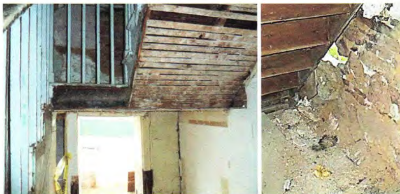
36. Stair landing just above head of North door & upper run to Second Floor 37. Missing masonry at West wall beneath stair, just North of West entry door
