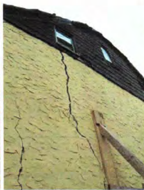
17. Bulge at Western portion of East Wall, adjacent to chimney
