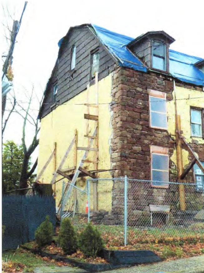
Photo 01 – General view of northeast corner of house showing shoring at east and north walls. Northeast corner of masonry wall has recently been rebuilt.
