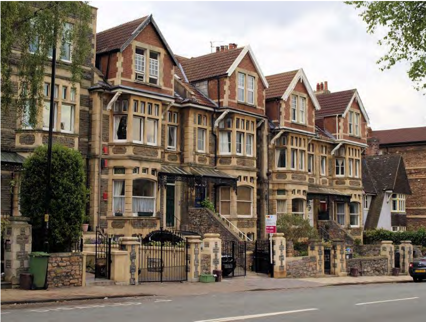
Figure 12 Circa 1890 semi-detached builder townhouses. Note the contrasting masonry, tall window bays, and multi-pane sash windows. Credit: University of the West of England on 5/30/2018
