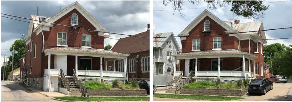
Figures 19-20 114 N. Gilbert. Clearly a free classic variation of the Queen Anne style, this house is now a student rental and has some minor alterations, especially to side windows. References to classical architecture include dentils and pediment returns in the gables, the round-arched gable window, and the front porch's smooth columns. May 2018
