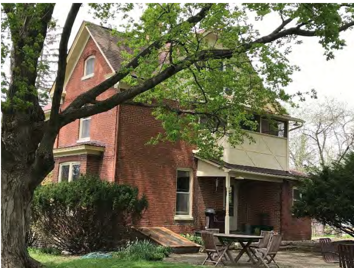
Figure 3 View of the south side and the east rear walls. Note the patio and the basement storm door near the south corner of this east elevation, both from the 1970s (see Alterations section). May 2018
