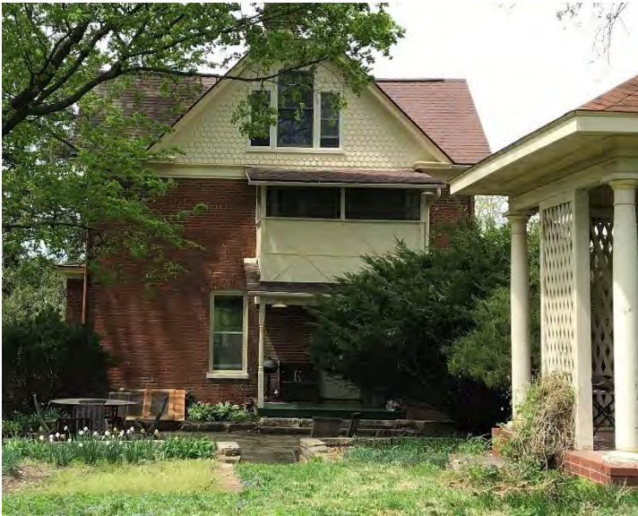
Figure 4 Another view of the east rear wall, with the open-air modern gazebo at the right edge in the photograph. May 2018
