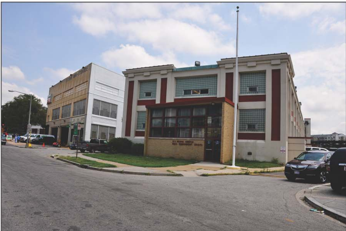
PHOTO 2: View of Southwest Elevation, Looking Northeast
