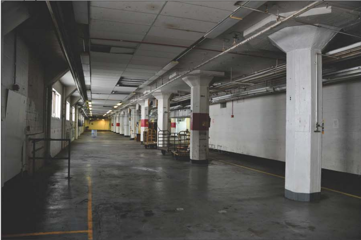
PHOTO 18: First Floor, View of Manufacturing and Storage Areas Looking Southeast Toward Press Room
