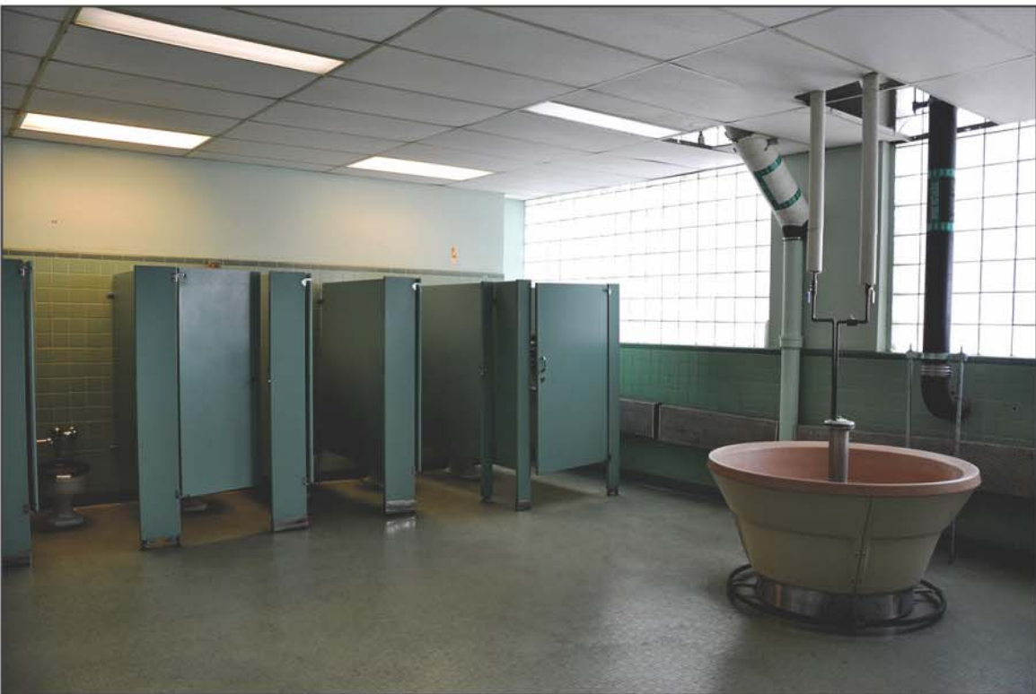
PHOTO 25: Second Floor, Western Portion of Building, Women's Toilet
