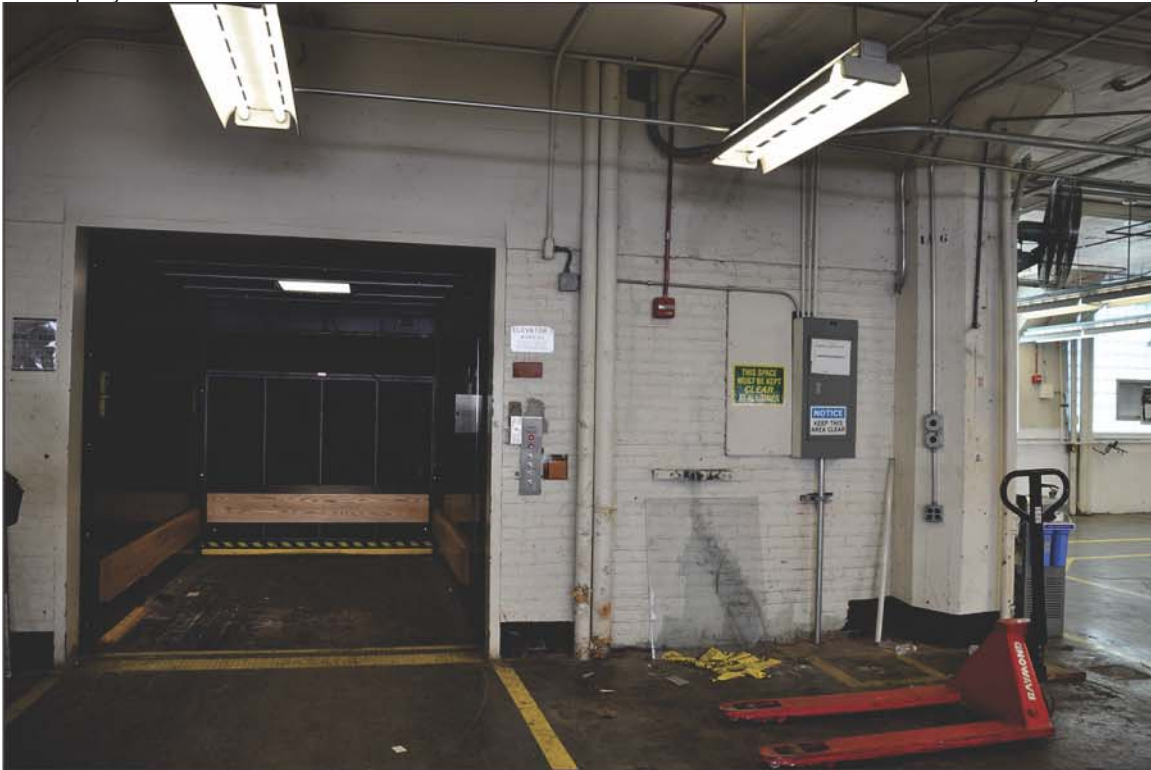
PHOTO 16: First Floor, View of Elevator No. 1
