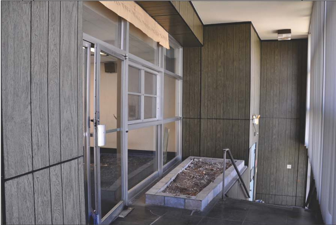
PHOTO 11: First Floor, Entrance Vestibule (ca. 1965) Looking South
