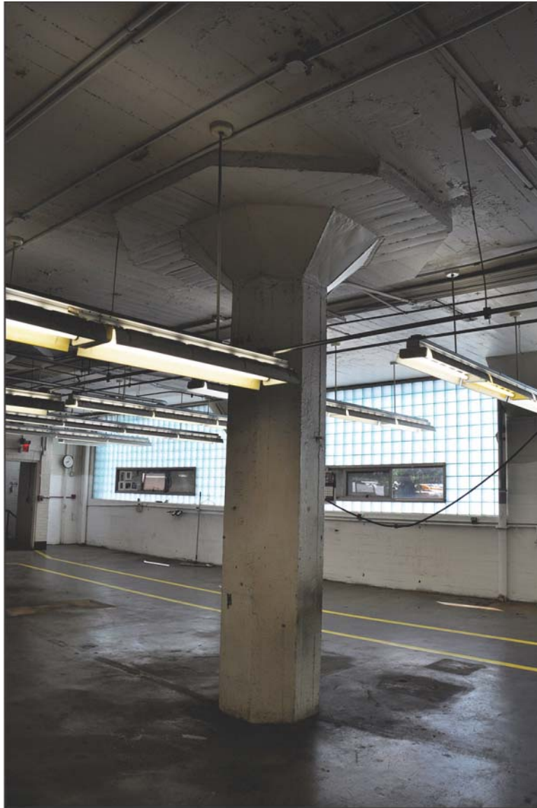
PHOTO 15: First Floor, Detail of Column
