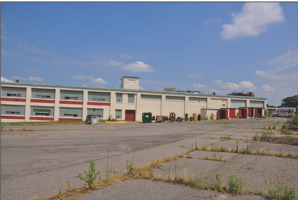
PHOTO 6: View of Southeast Elevation East End, Looking Northeast
