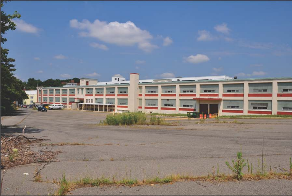
PHOTO 7: View of Southeast Elevation, Looking Northwest
