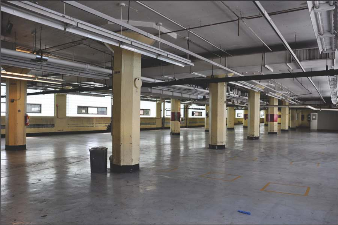
PHOTO 24: Second Floor, Key/Lock Manufacturing Area, Looking Southwest
