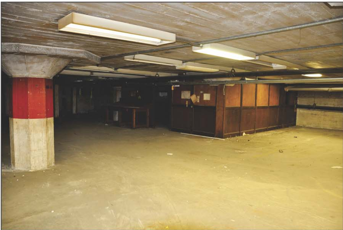
PHOTO 10: Basement, View of Storage Area
