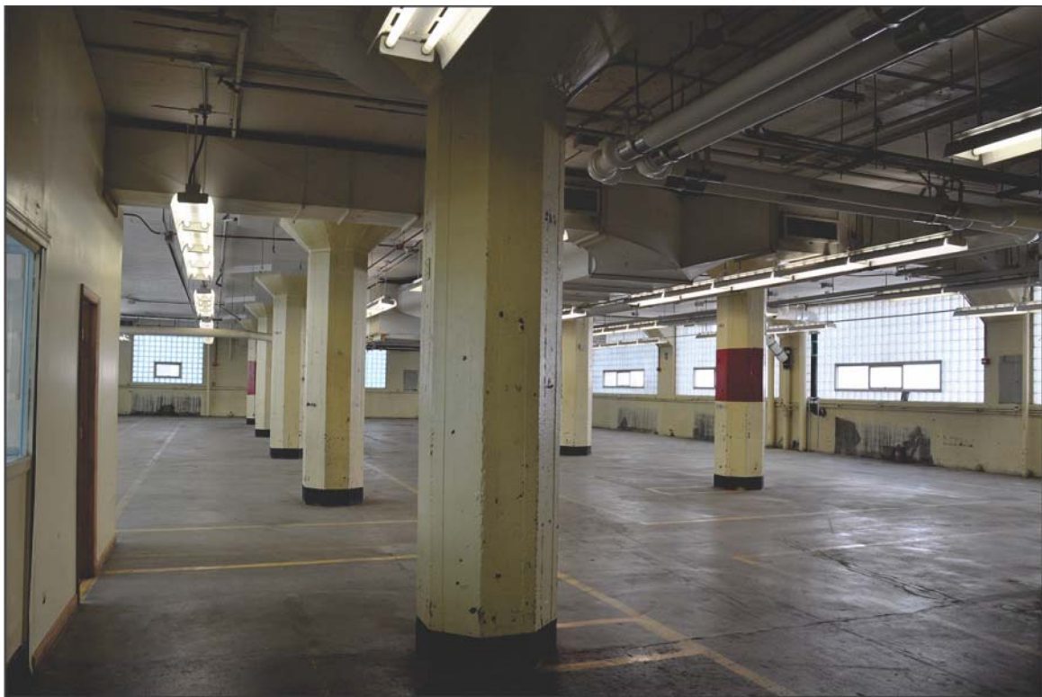
PHOTO 26: Second Floor, Western End of Building, Looking Northwest
