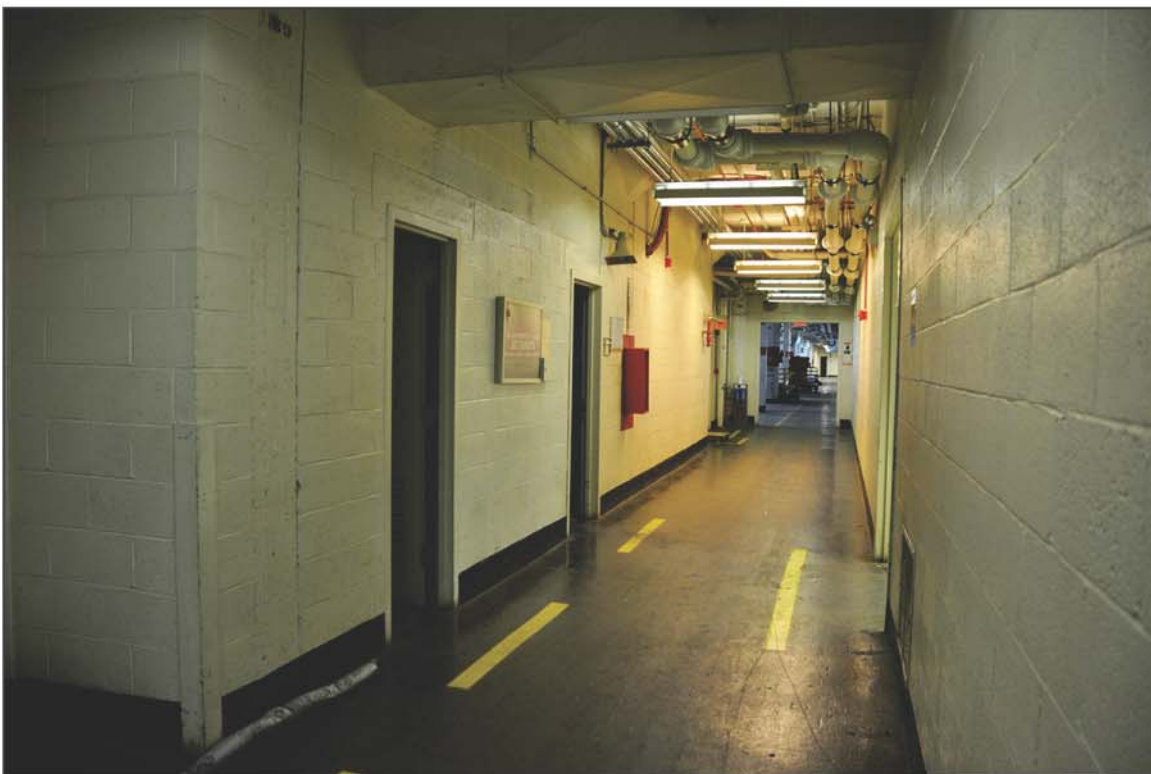
PHOTO 17: First Floor, Western Portion of Building, Corridor Adjacent to Cafeteria, Looking Southeast
