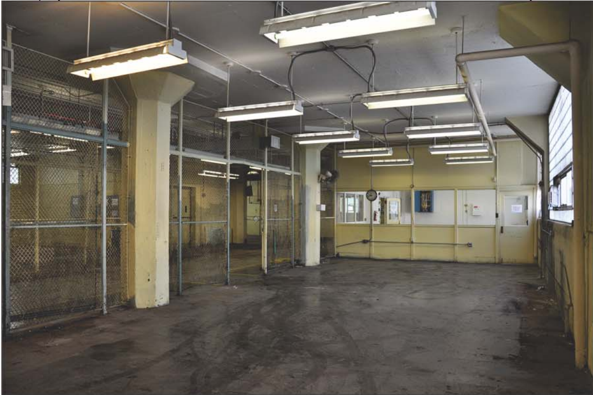
PHOTO 22: Second Floor, Storage Area, Looking East Toward Stock Room Office
