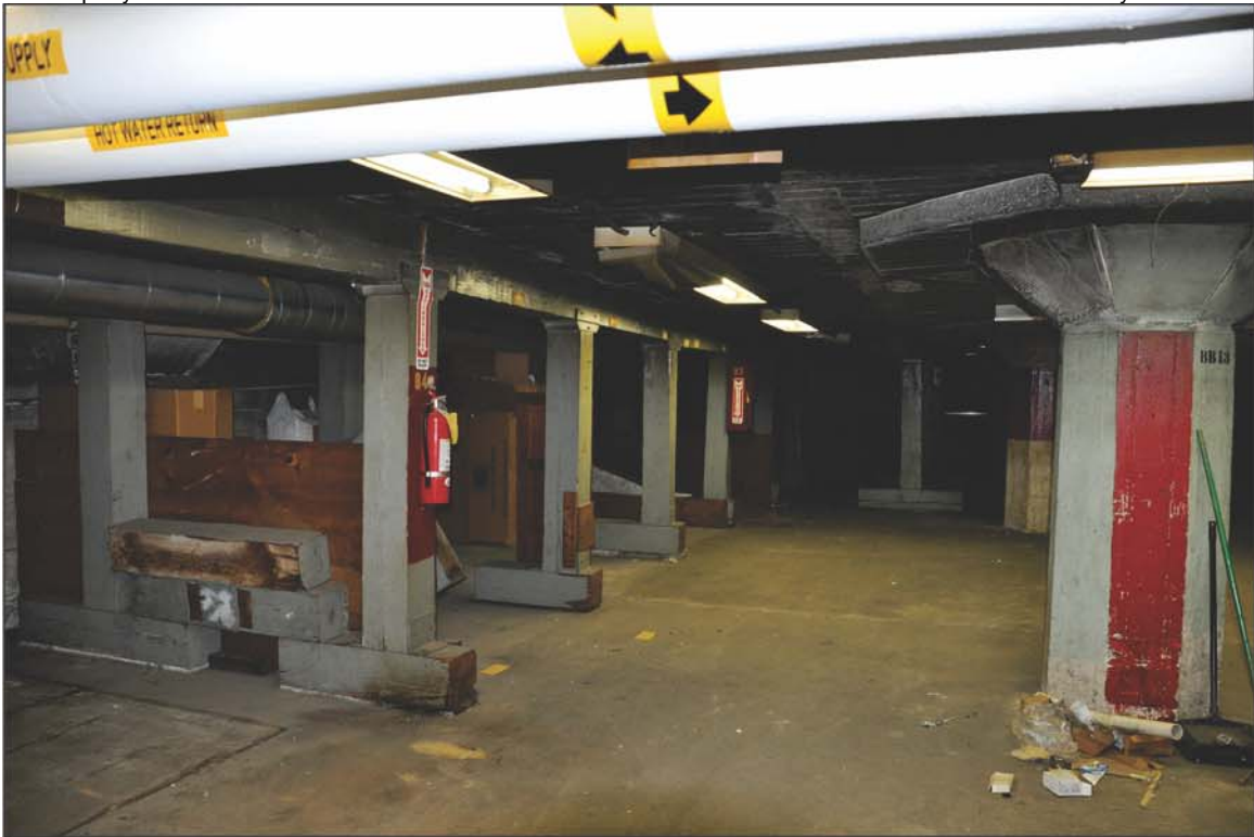
PHOTO 9: Basement, View of Storage Area, Wooden Supports
