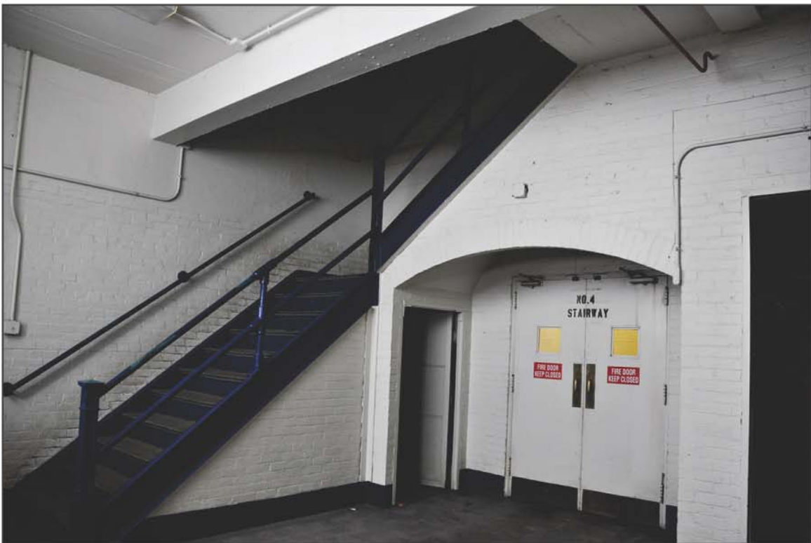
PHOTO 19: First Floor, Stairway No. 4
