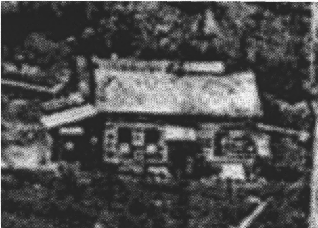
Enlarged, cropped detail from early 20 th century panorama of Lion and Cleve Mountains. Photo shows the Hecla Residence. Note the shed roof above the entrance and the lean-to at the west side of the building.
