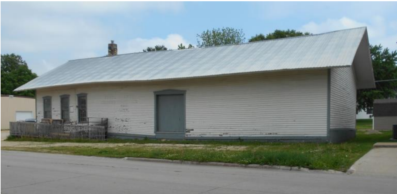
Figure 3 Long northwest elevation with three passenger-waiting-area windows and wide door into the freight room. To the right is the narrow gabled southwest end wall.
