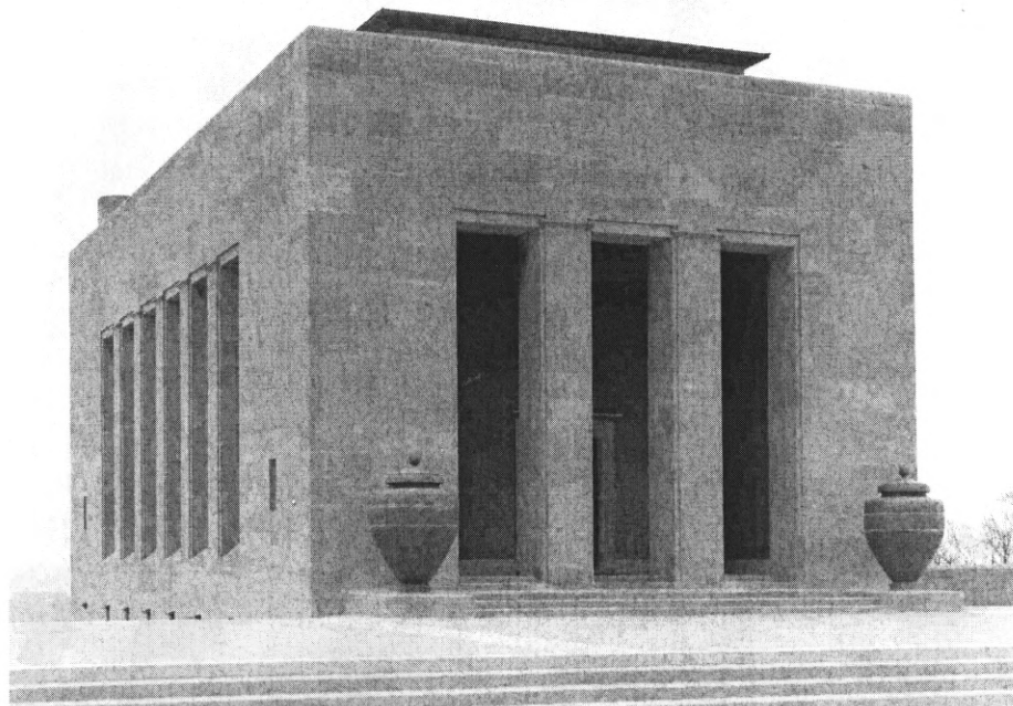
Museum building east façade, view facing northwest. Photograph by Len Fohn, Summer/Fall 2003.
