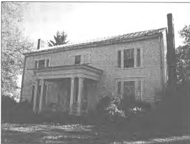
Plate 6. Main dwelling, front (west) façade
