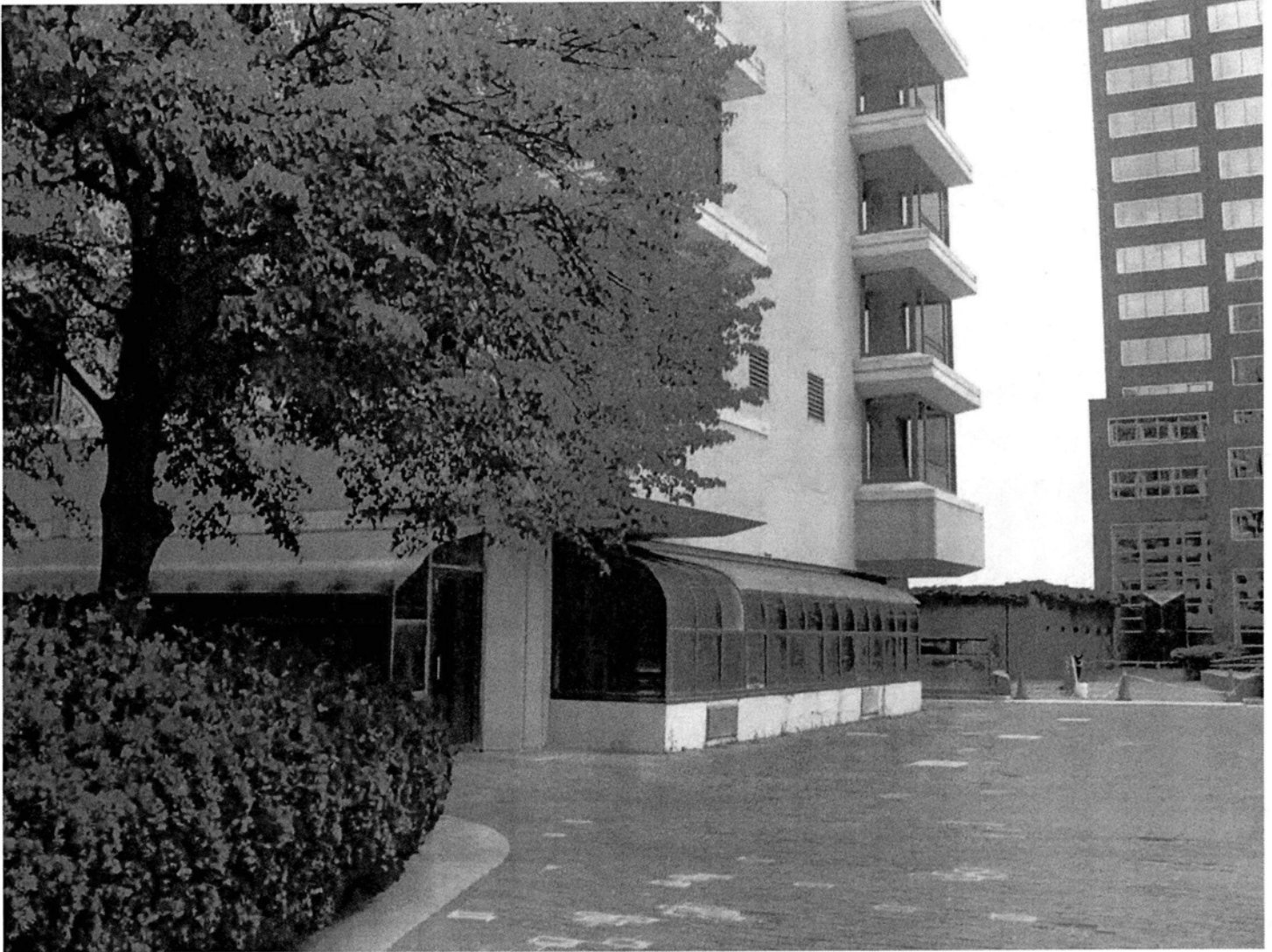
West (rear) and south (side) elevation of hotel from Constitution Plaza, showing enclosed terrace details.
