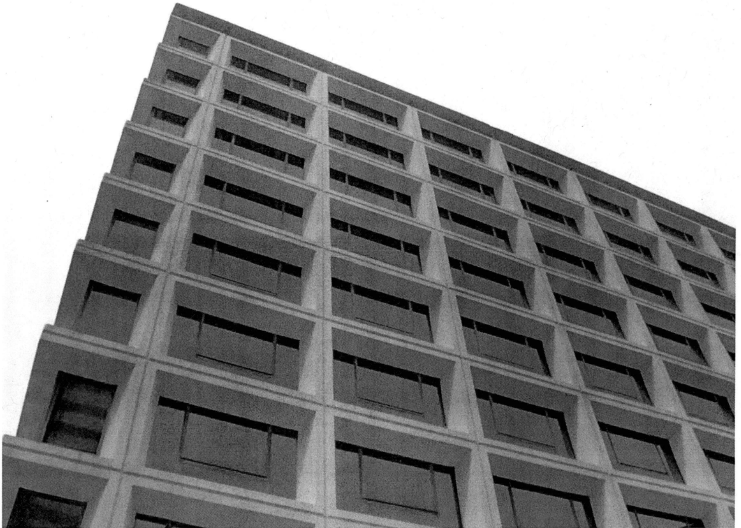
East (front) elevation of hotel from Columbus Boulevard, showing window and wall details. Camera facing northwest. Photograph 10 of 28.
