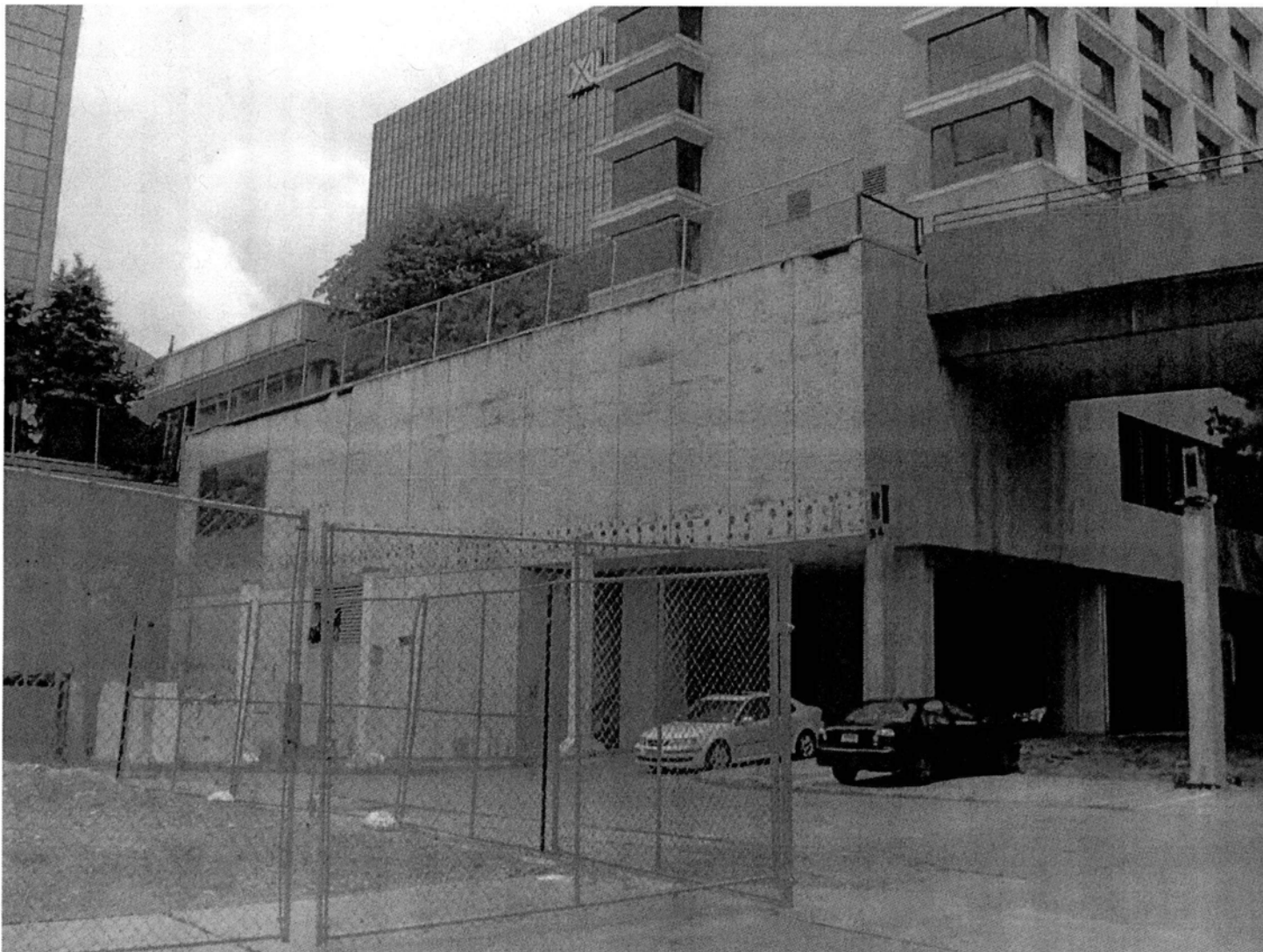
East (front) and south (side) elevations of hotel from Columbus Boulevard, showing window, column, and wall details. Camera facing northwest. Photograph 4 of 28.
