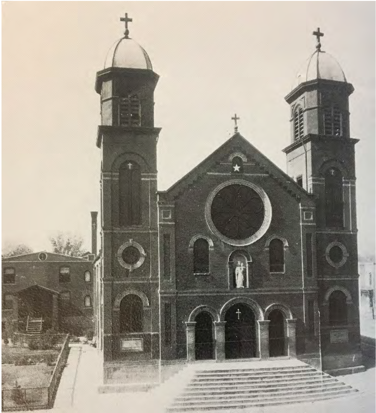
H3. Undated (circa 1910), showing Church prior to alterations to entrance stair, Rectory, or memorial garden. Source: Our Lady of Mount Carmel (1975) 16.
