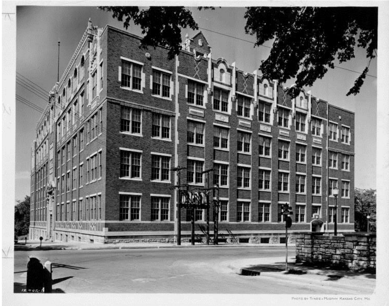
Figure 14: Westport Junior High School, south and west elevations, n.d. Source: Missouri Valley Special Collections, Kansas City Public Library, Kansas City, Missouri.
