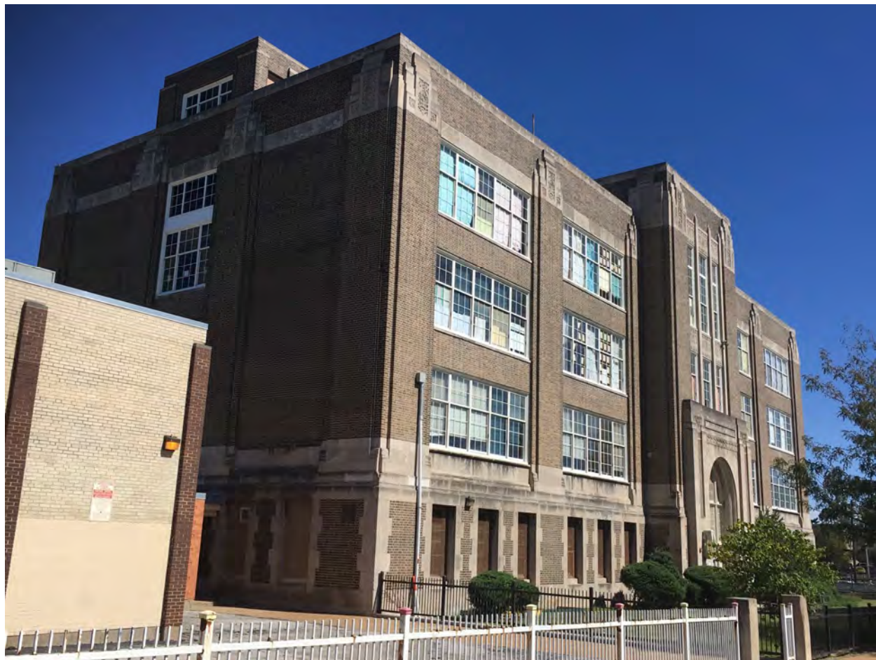
Figure 25: Cole School (1931; George W. Sanger). Source: Preservation Research Office Photograph, September 2016.
