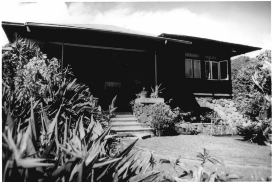
BURNINGHAM RESIDENCE, HONOLULU, HI
