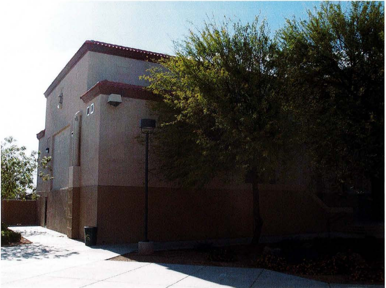
Photo 6. Auditorium, facing east.
