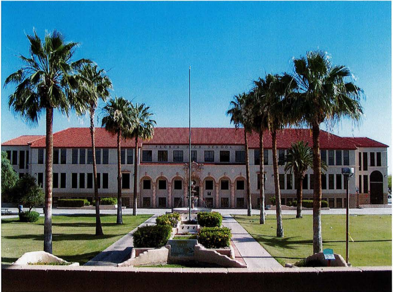
Photo 1. Front façade, facing north.
