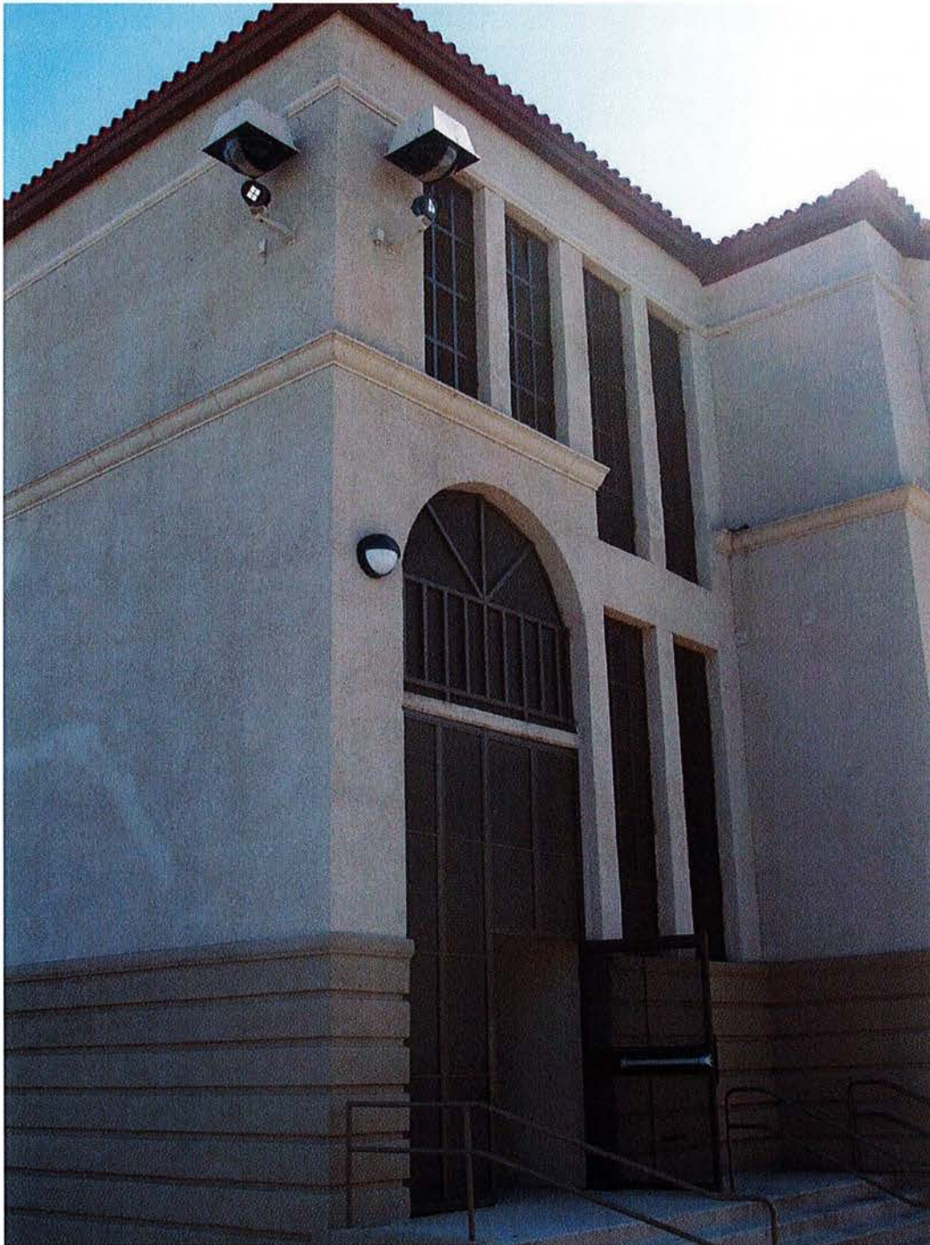
Photo 7. Enclosed staircase on west end, facing northeast.
