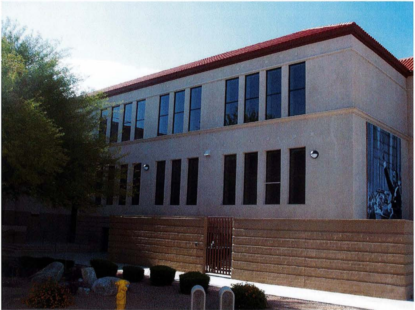
Photo 5. Rear of building, facing southeast.
