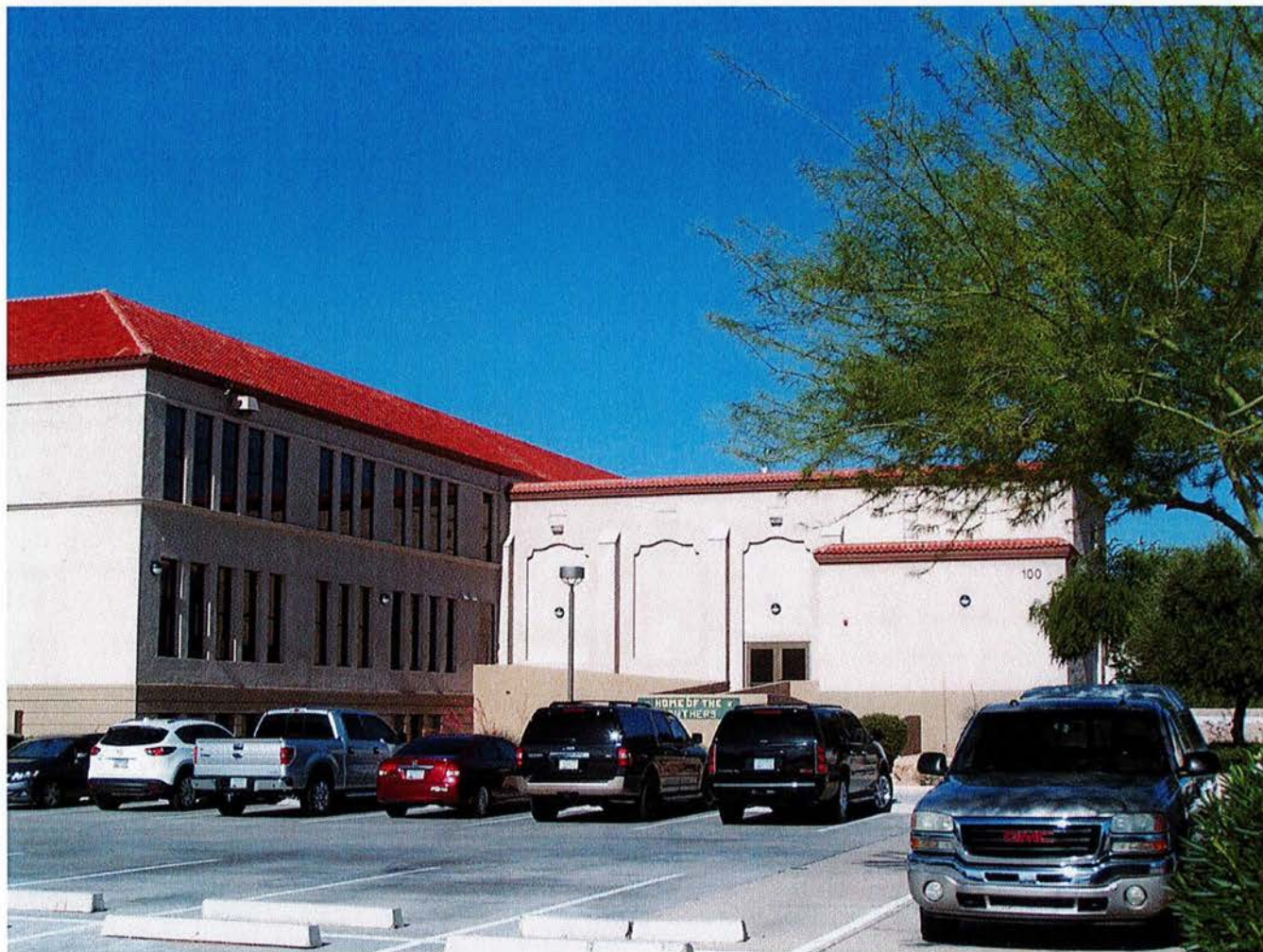
Photo 3. Rear and auditorium, facing southwest.
