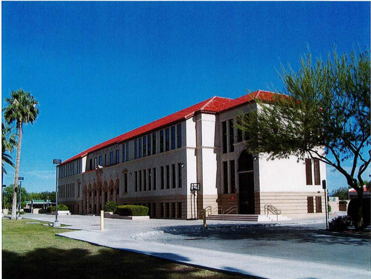
Figure 5. The eastern 1958 stairwells, facing west.
