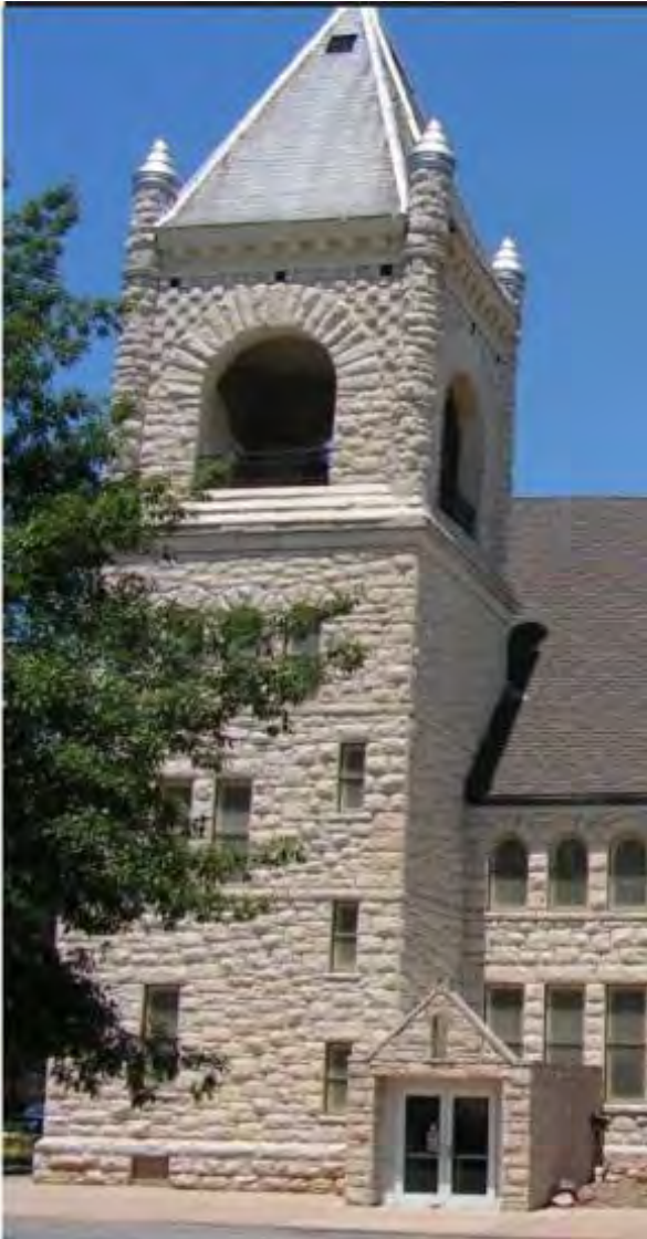
Figure 13: Entry and stairwell to old fellowship hall
