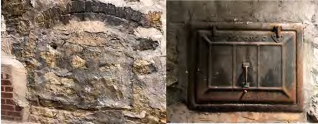
Figure 14: Original coal chute (left) and ash clean out door (right)
