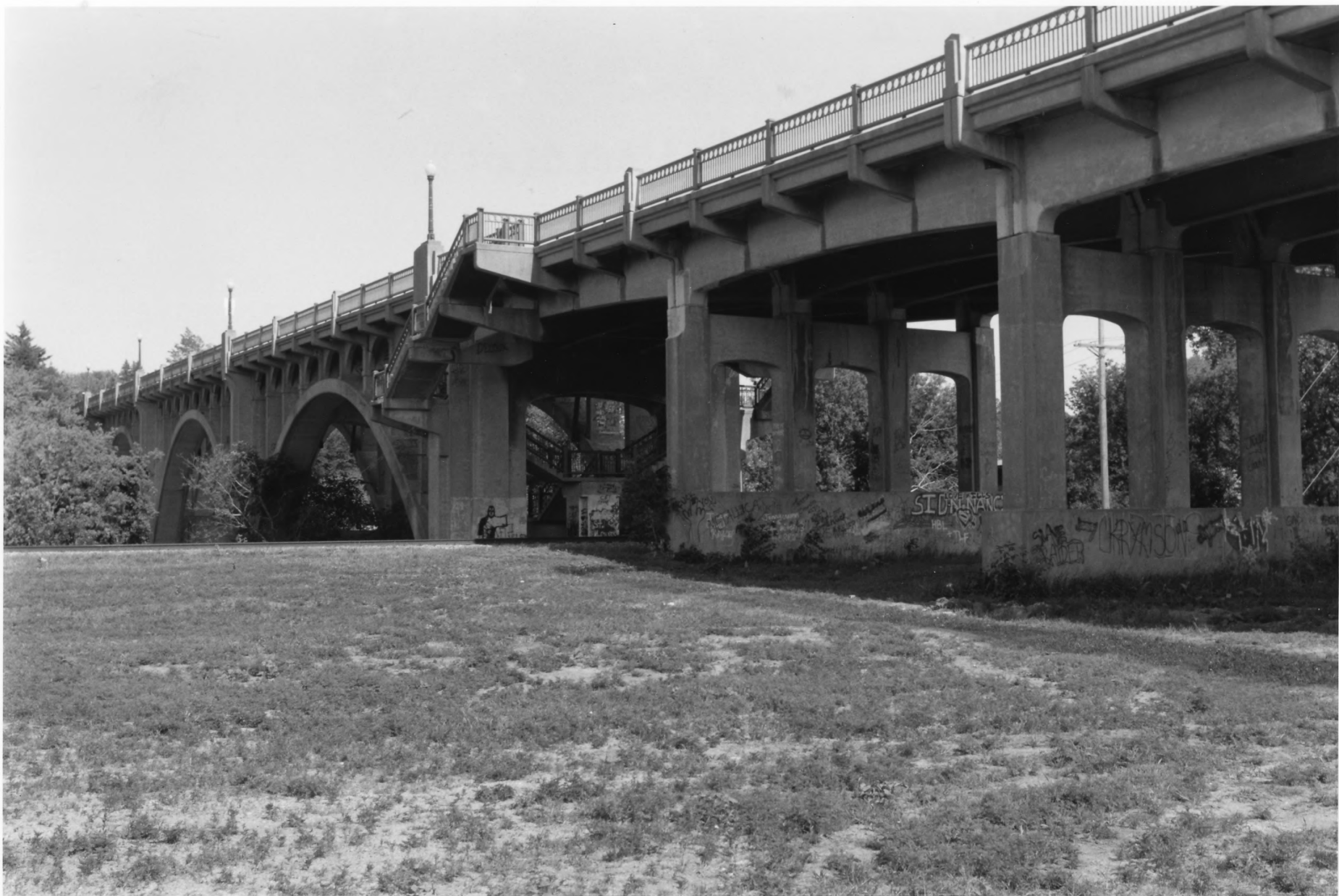
FARIBAULT VIADUCT, NO. 5370 FARIBAULT, RICE CO., MN. PHOTO I.D. 09972 #19
