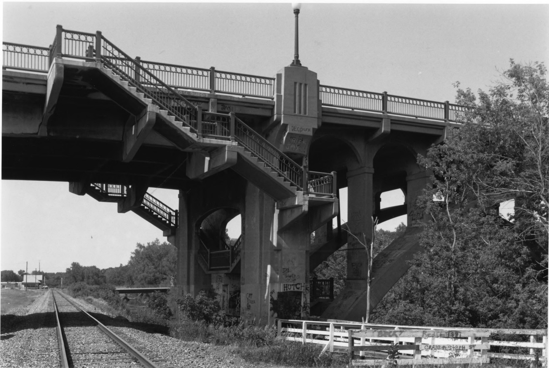
FARIBAULT VIADUCT NO. 5370 FARIBAULT, RICE CO., MN PHOTO I.D. 09972# 9
