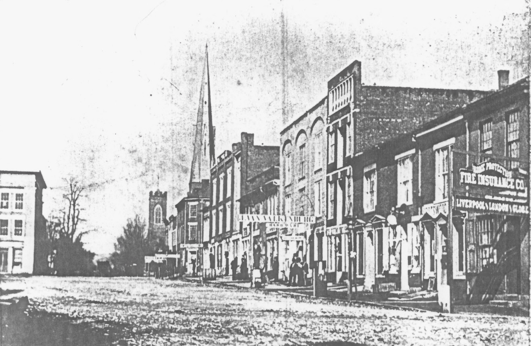
SOUTH SIDE SQUARE (#24-33) Huntsville, Alabama Photographer unknown; before 1878 Huntsville Public Library View from the west
