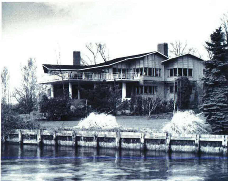
Lionel H. Pries, Max and Helen Gurvich house, Seattle, 1964-65; view from pier in Lake Washington; photo courtesy of Helen Gurvich.
