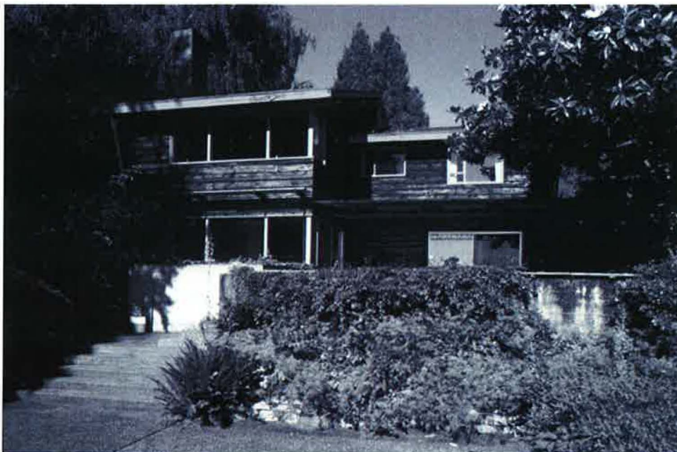
Lionel H. Pries, Richard and Ruth Lea house, Seattle, 1956-57 (destroyed); view of side facing Lake Washington; photo by Jeffrey Karl Ochsner.
