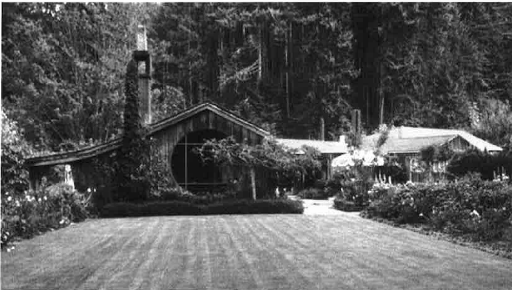
Lionel H. Pries, Ernest and Anne Gayler house, on Hood Canal, 1937-41, 1945-46 (altered--addition to rear); early example of a regional approach to modernism; photo by William Matchett.
