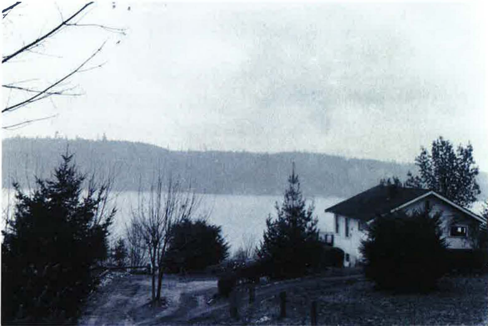
Barksdale cottage, Seattle, ca. 1940-41; relocated cottage on new concrete block daylight basement; photograph given to current owners by Tucker Barksdale.
