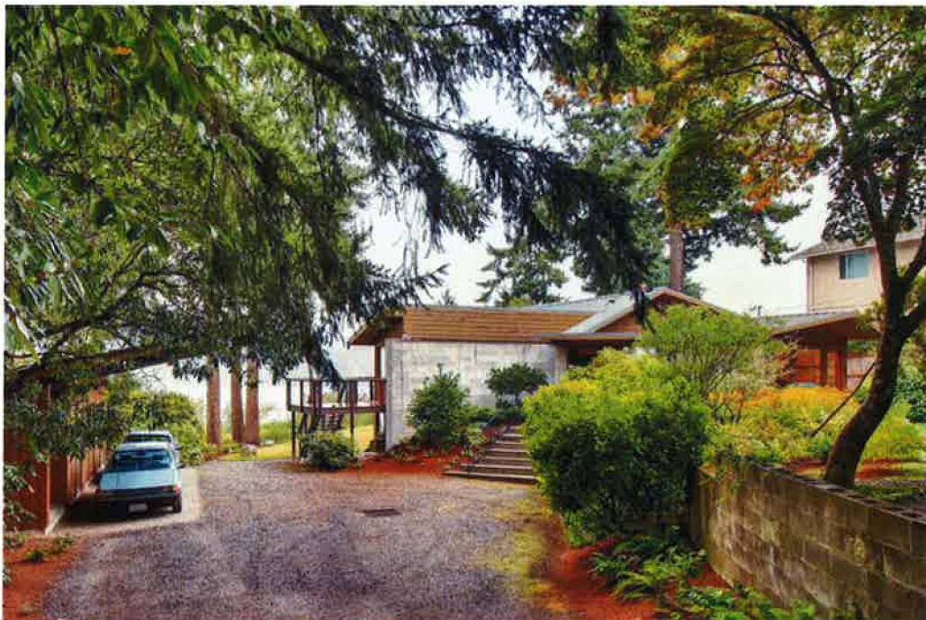
3 of 19: Driveway to Barksdale house, on right; carport [non-contributing] on left; camera facing east; photo by Vista Estate Imaging, September 2010.
