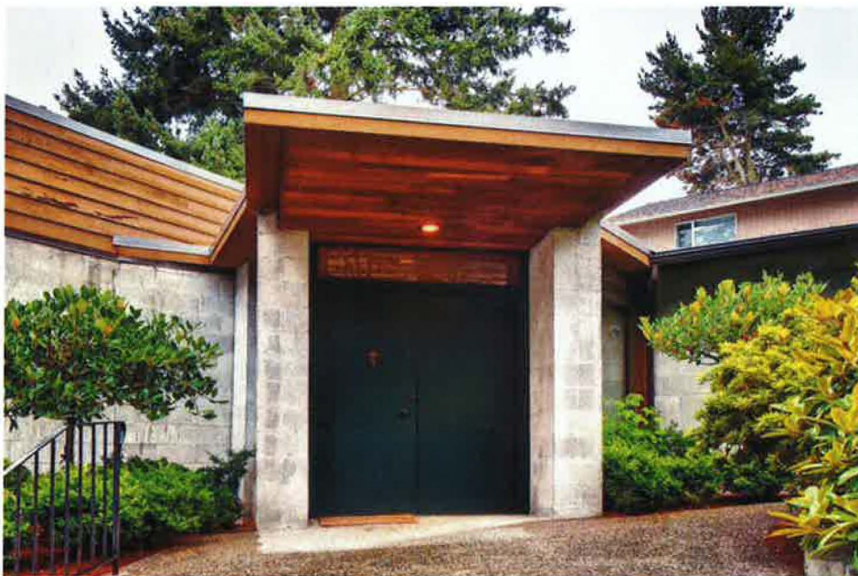
9 of 19: Barksdale house, front entry; camera facing southeast; photo by Vista Estate Imaging, September 2010.
