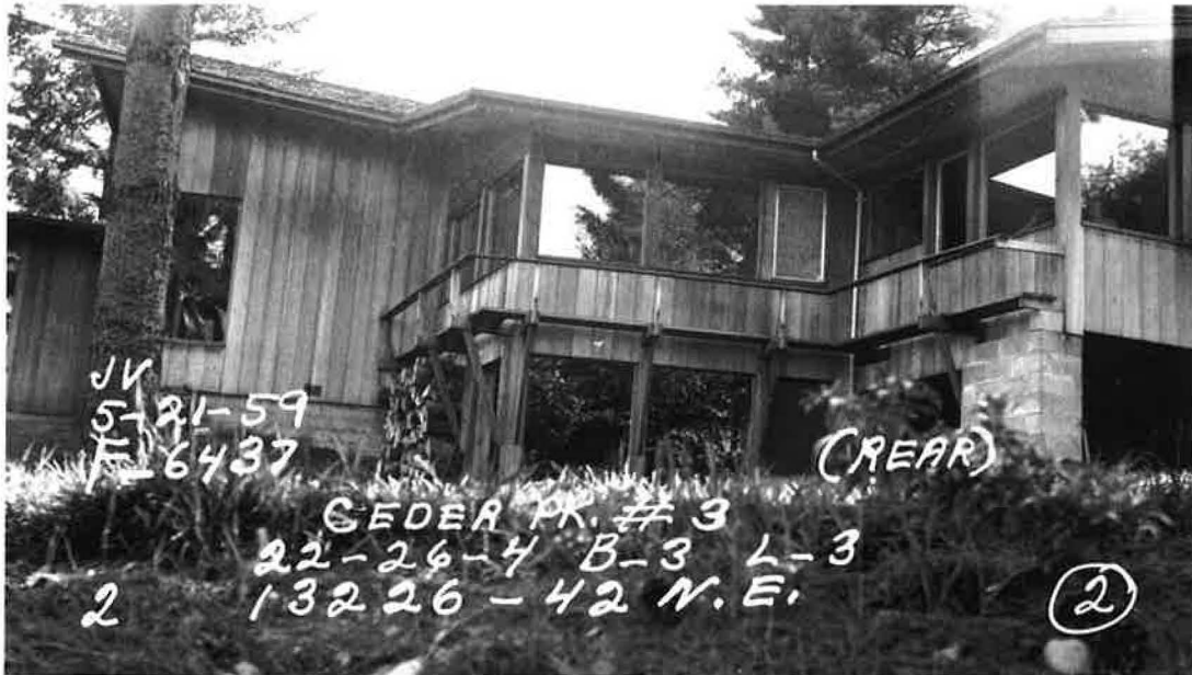
Lionel H. Pries, architect; Barksdale house, Seattle, 1949-50; view of northeast elevation (1955 addition to far left, living room and dining area in center, kitchen to right; note that space below kitchen is not yet enclosed to become utility room); photographed 21 May 1959; Washington State Archives, Puget Sound Regional Branch.
