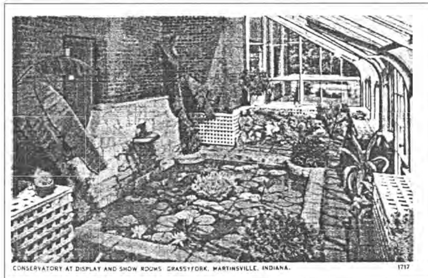
HP4. Interior of conservatory, c. 1940. Camera facing north.
