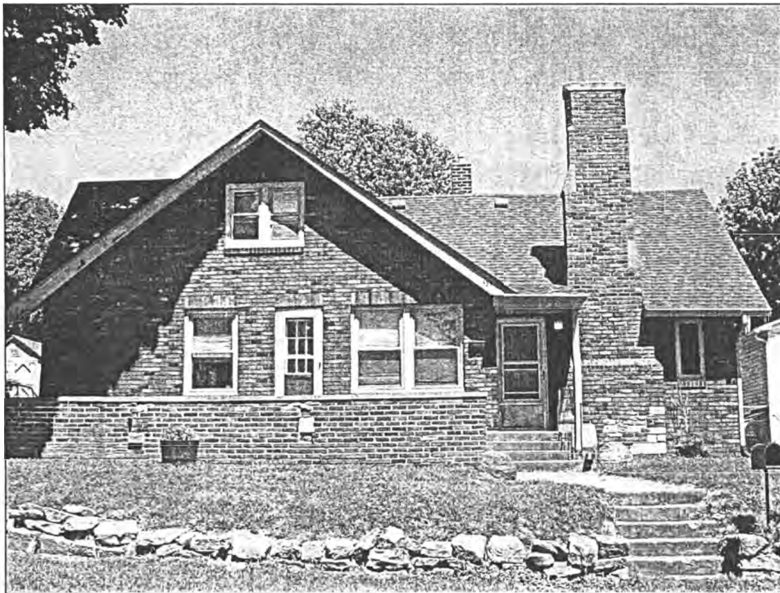
JC 8. 389 N. Grant St., c.1940. This house was built by the Cramer brothers for their mother, June. Cramer signatures include the mosaic mallard duck in the chimney face (made by Julian), hand-forged iron railing, landscape features such as rock concretions and the sandstone stone retaining wall, and on the interior, arched openings, handmade hall light fixture, textured stucco walls, and hand-forged railing (missing).
