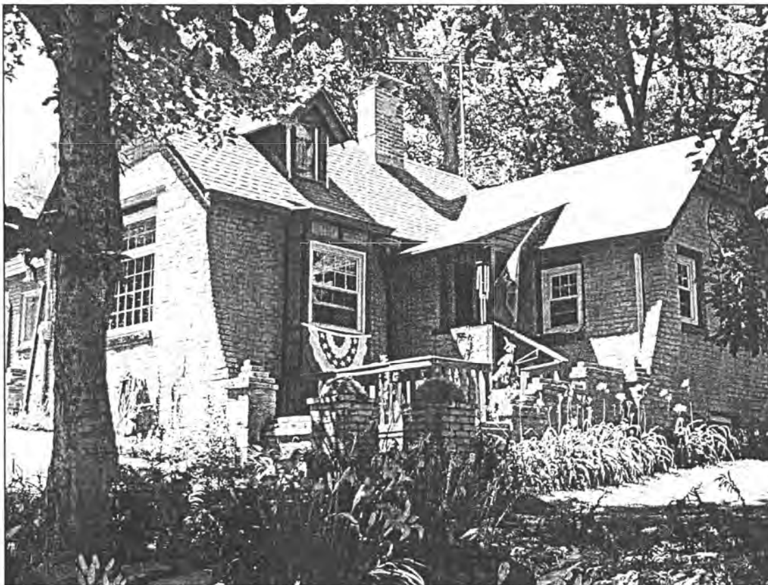
JC 9. 410 N. St. Clair St., c.1946. The house that Julian Cramer designed and built for himself features eccentric and whimsical elements, including brick courses "laid off the line," a door made from a cobbler's bench salvaged from the Old Hickory Furniture Co., a concrete relief image of his dog, Ruby, on the chimney face, hand-forged ironwork, and concretions used in the designed landscape. The house is an excellent example of folk art.
