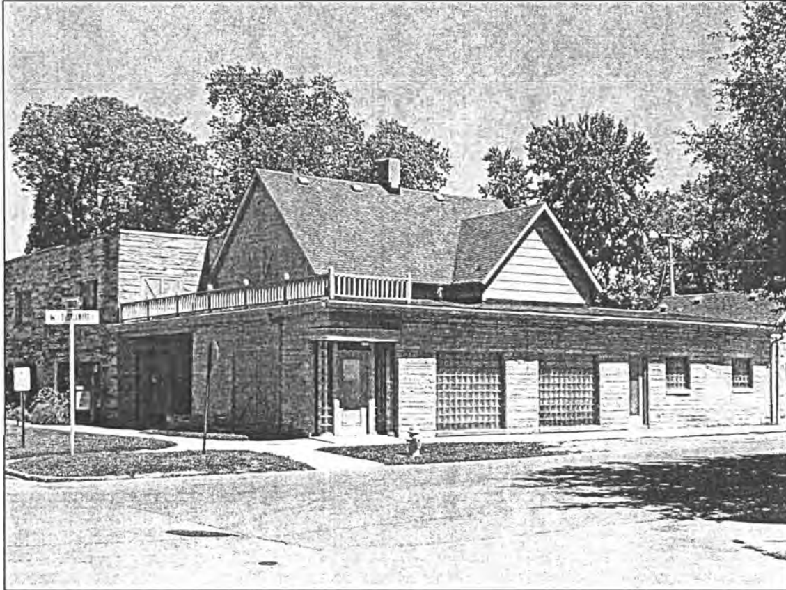
JC 10. 219 E. Washington St., c.1940. Julian combined several buildings for Dr. Wolf, an optometrist, by constructing a new commercial front made of limestone and glass block. The corner entrance features a floor of colored and incised concrete. The Washington Street entrance has a wall face of water struck Norman brick. Dr. Wolf was involved with the development of Lake Lemon in Monroe County. Julian built sea walls and buildings for him on the lake's north shore.
