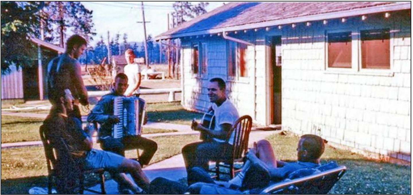
Figure 7: 1954 Barracks Building, west entrance looking northeast, nd. Jerry John Collection.
