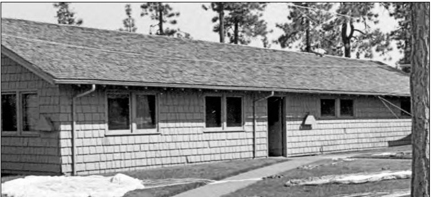
Figure 8: 1954 Barracks Building, north facade, looking south, 1960s or 1970s. Doug Beck Collection.
