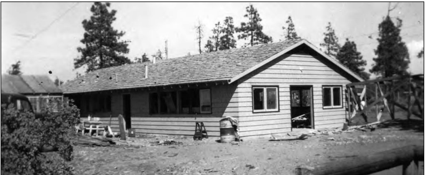
Figure 6: 1954 Messhall during Construction, 1954. Bill Buck photo.
