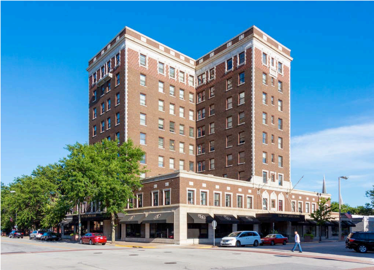
Figure 21: The Fort Armstrong Hotel as it stands today, view toward southeast. Source: Brandon Bartoszek photograph on Flickr, taken July 8, 2016.
