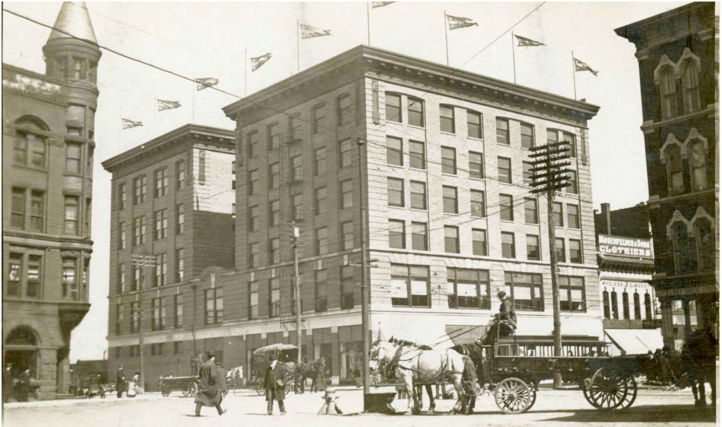
Figure 16: Historic photograph of Best Building, undated. Source: Rock Island Preservation Society.
