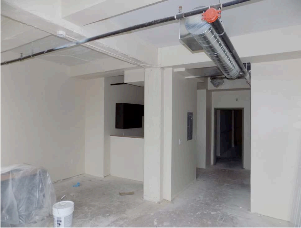
Figure 13: Interior of building showing exposed concrete structural system. Source: Michael Allen photograph taken June 20, 2016.
