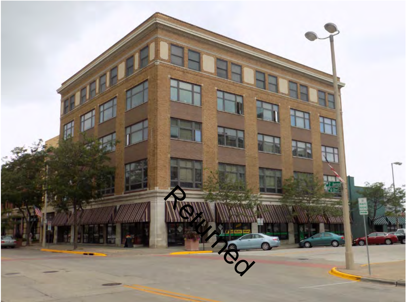
Figure 19: The Goldman Building, view toward the northwest. Source: Michael Allen photograph taken June 24, 2016.
