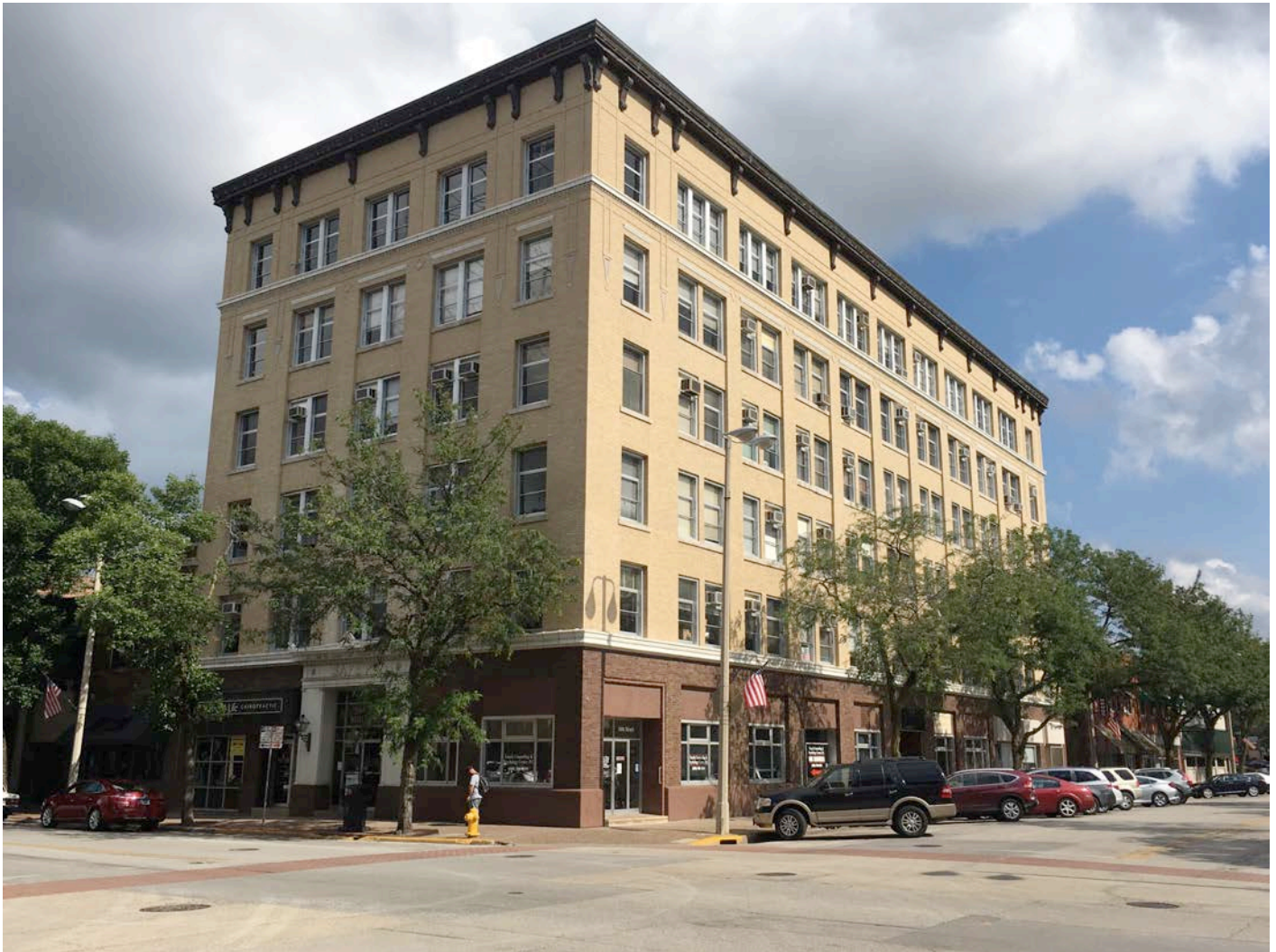
Figure 17: Safety Building, view toward southeast. Source: Michael Allen photograph taken June 24, 2017.
