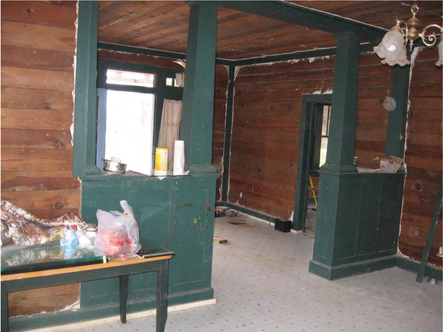
Figure 16. 2009 photograph taken from the kitchen door into the Living Room towards the front door (just left of center in background). The green “boxes” are the backs of the two built-in book shelves. Notice that even the ceiling is made of cypress planks. Image courtesy of Kerry Lincoln.
