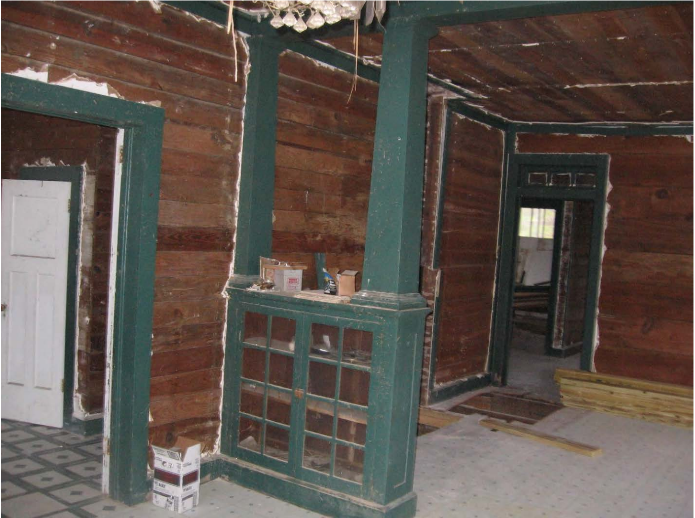
Figure 13. 2009 photograph taken from inside the front door facing slightly south towards bedroom door (far left). A built in book shelf is noticeable in the center. The door in back right of photo goes into the hall where two bedrooms and a bath connect to a small hall to back door. The sheet rock had been peeled off exposing solid cypress walls. Image courtesy of Kerry Lincoln.
