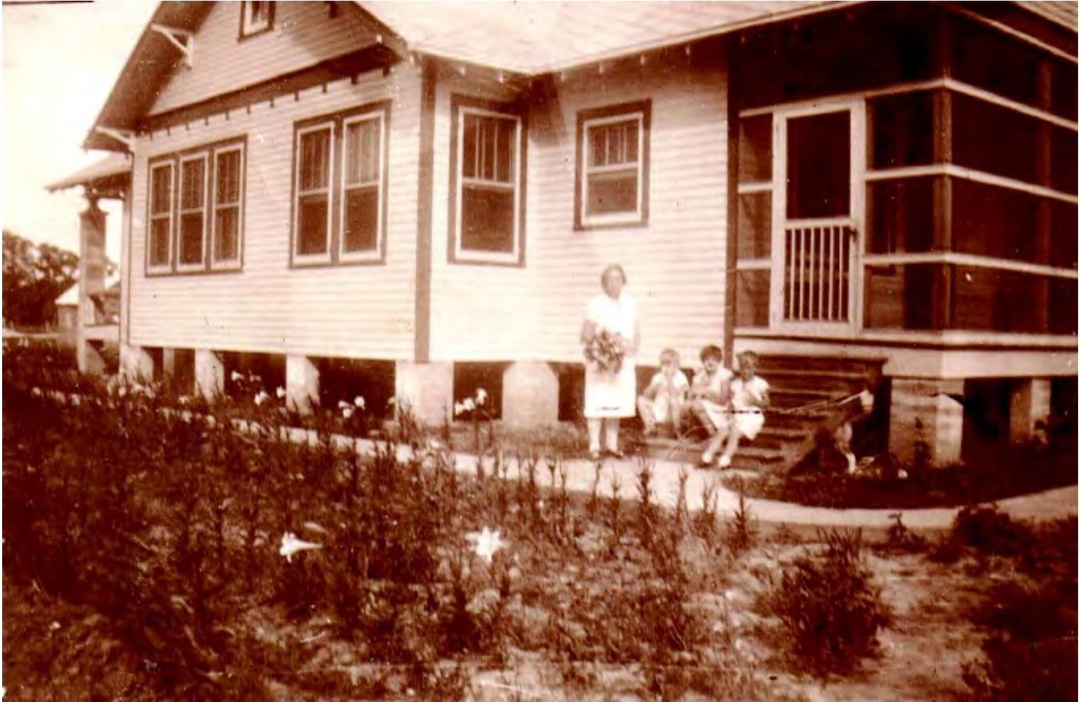
Figure 7. 1932 photograph of the rear and side elevation showing the rear porch once the screening had been installed. The screening has since been removed, but the original framing and door remain in place. Image courtesy of Rod Lincoln.
