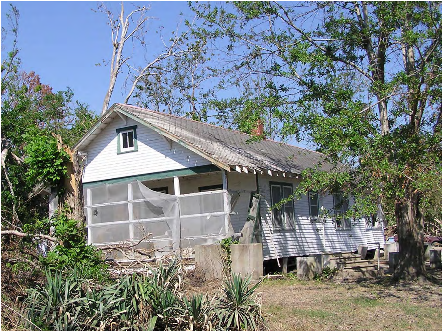
Figure 8. The Lincoln House in 2006. Notice the concrete structure on the right corner of the house. This was the cistern support. To the right of that are the steps that went onto the back porch. The house was still off its piers when this photo was taken. Image courtesy of Rod Lincoln.
