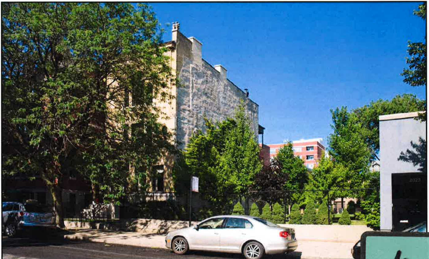
Photo 3 - Reid House and Replacement Parcel
