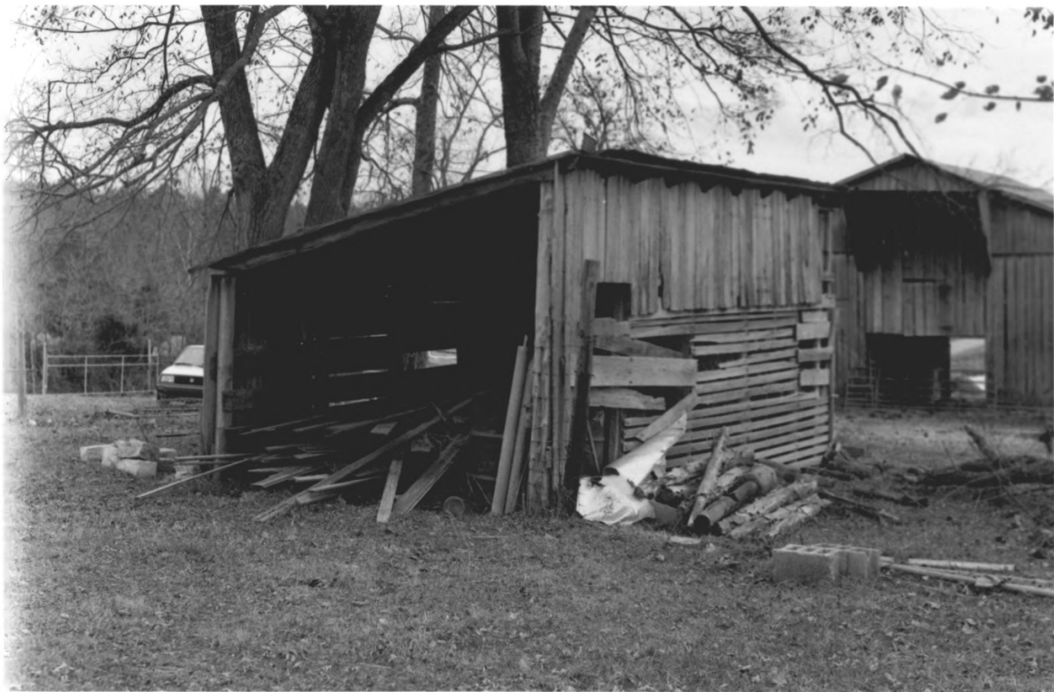
BRITAIN, JOSEPH, HOUSE MARSHALL COUNTY TN 27 of 29
