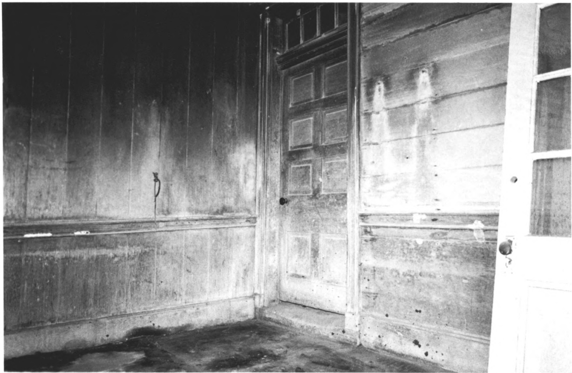
BRITAIN, JOSEPH, HOUSE MARSHALL COUNTY, TN 19 of 29
