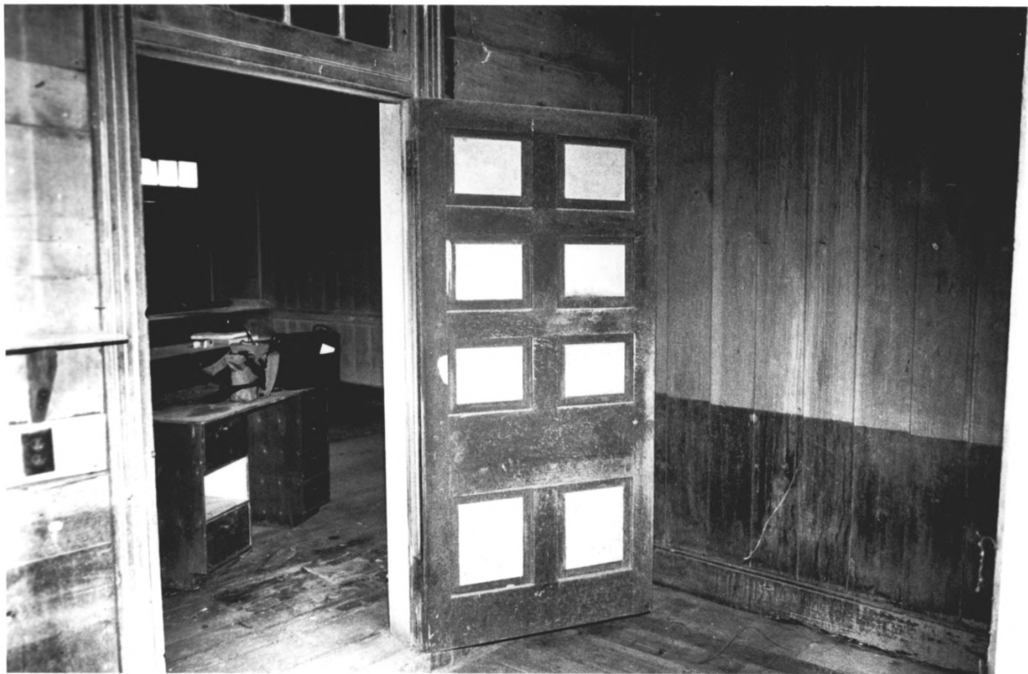
BRITAIN, JOSEPH, HOUSE MARSHALL COUNTY TN 18 of 29
