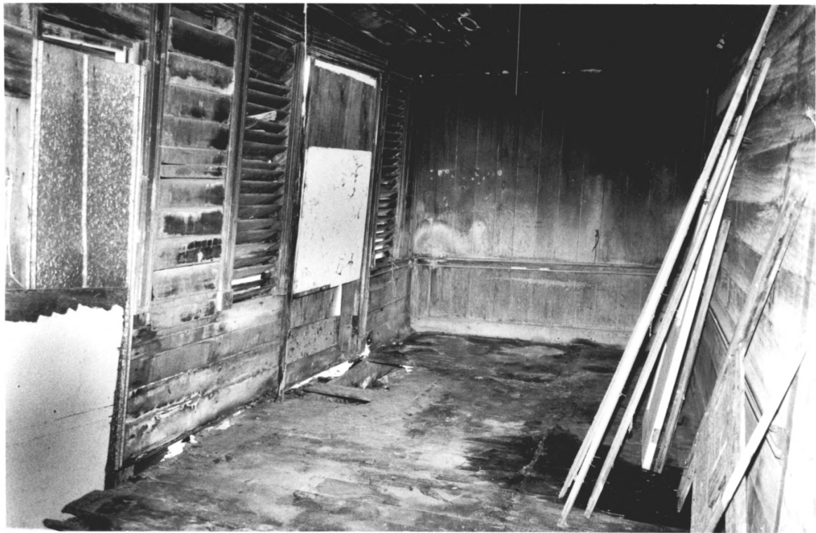
BRITAIN, JOSEPH, HOUSE MARSHALL COUNTY TN 21 of 29
