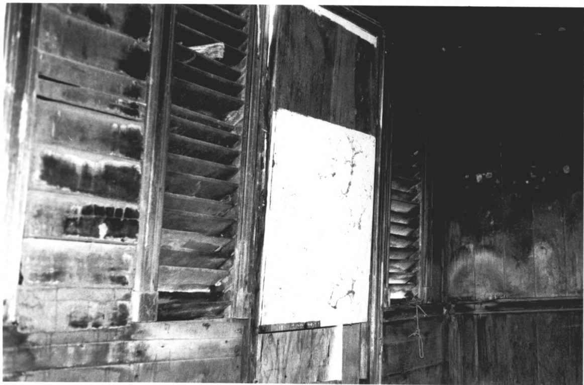
BRITTAİN, JOSEPH, HOUSE MARSHALL CO. TN 20 of 29
