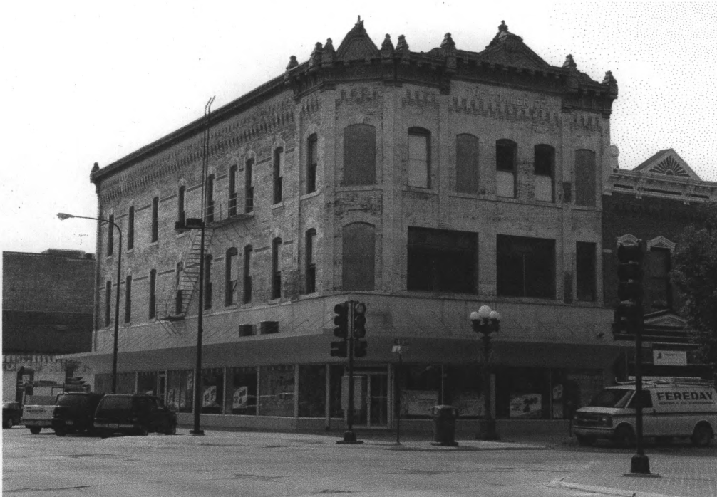
Figure 4 The Fowler Co. Building in 2005, before the present rehabilitation. The building's brick and stone walls were painted gray with the ornate cornice a darker battleship gray. Note the large second story window on the East 4th Street façade (right) and the heavy-looking hanging canopy over the sidewalk on both elevations. All these alterations were reversed. Photo by Tallgrass Historians L.C., 2005
