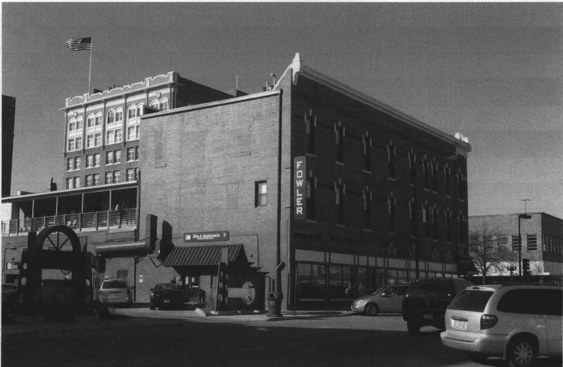
Figure 6 The rear wall of The Fowler Co. Building once closely faced a second Fowler warehouse and office building, erected in 1894. Bridgeways were created between the two buildings and their locations are faintly visible in this photograph. The second brick Fowler building was damaged by fire and is nonextant. The bridgeway openings and the remaining upper level windows on this rear wall have been filled in. Photo by Tallgrass Historians L.C., 2008
