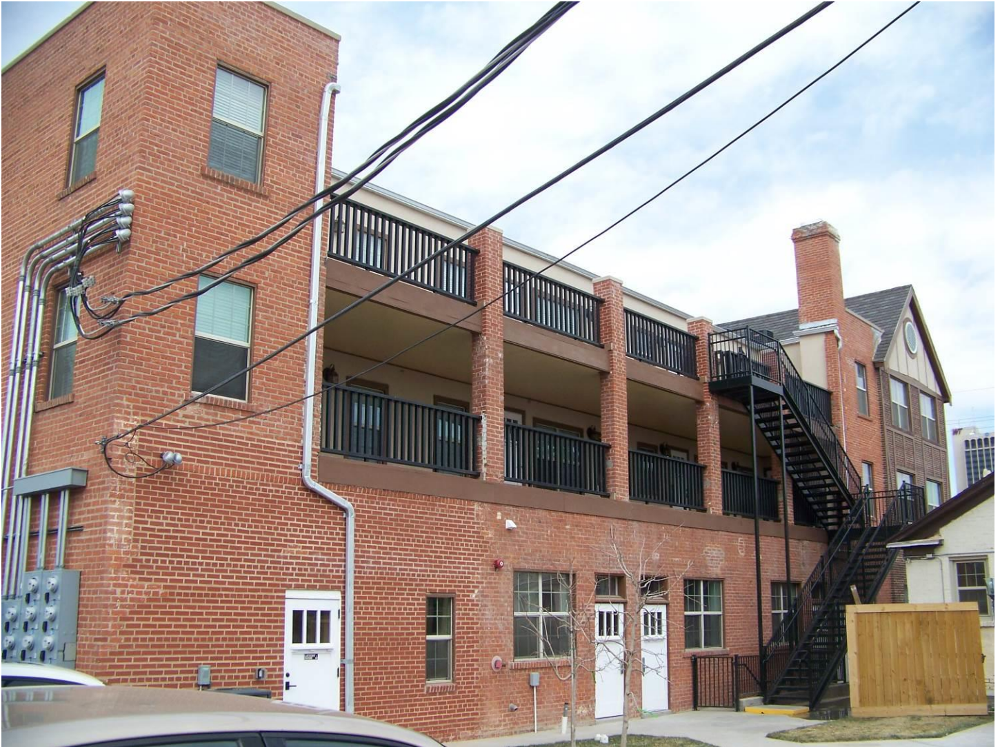
TX_Potter County_Vineyard Manor_0003.tif East (rear) elevation. Camera facing approximately northwest.
