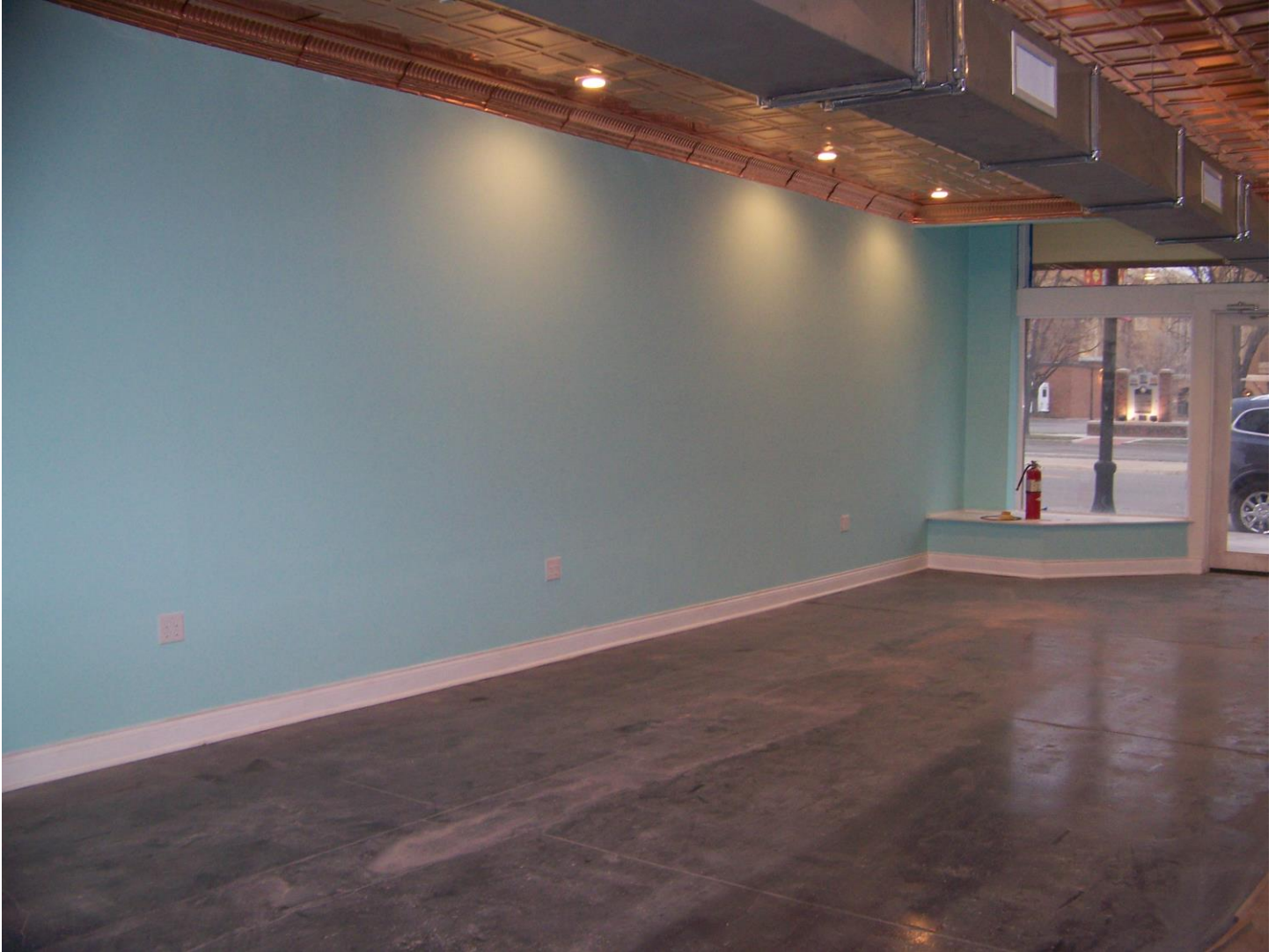
TX_Potter County_Vineyard Manor_0006.tif Interior, first floor retail space. Camera facing west. Photo taken on November 22, 2013.
