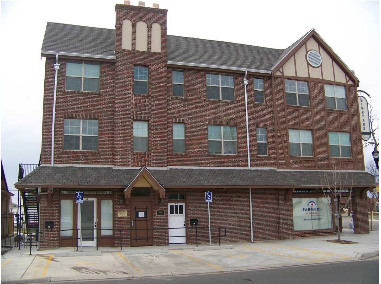
TX_Potter County_Vineyard Manor_0002.tif North elevation. Camera facing south.
