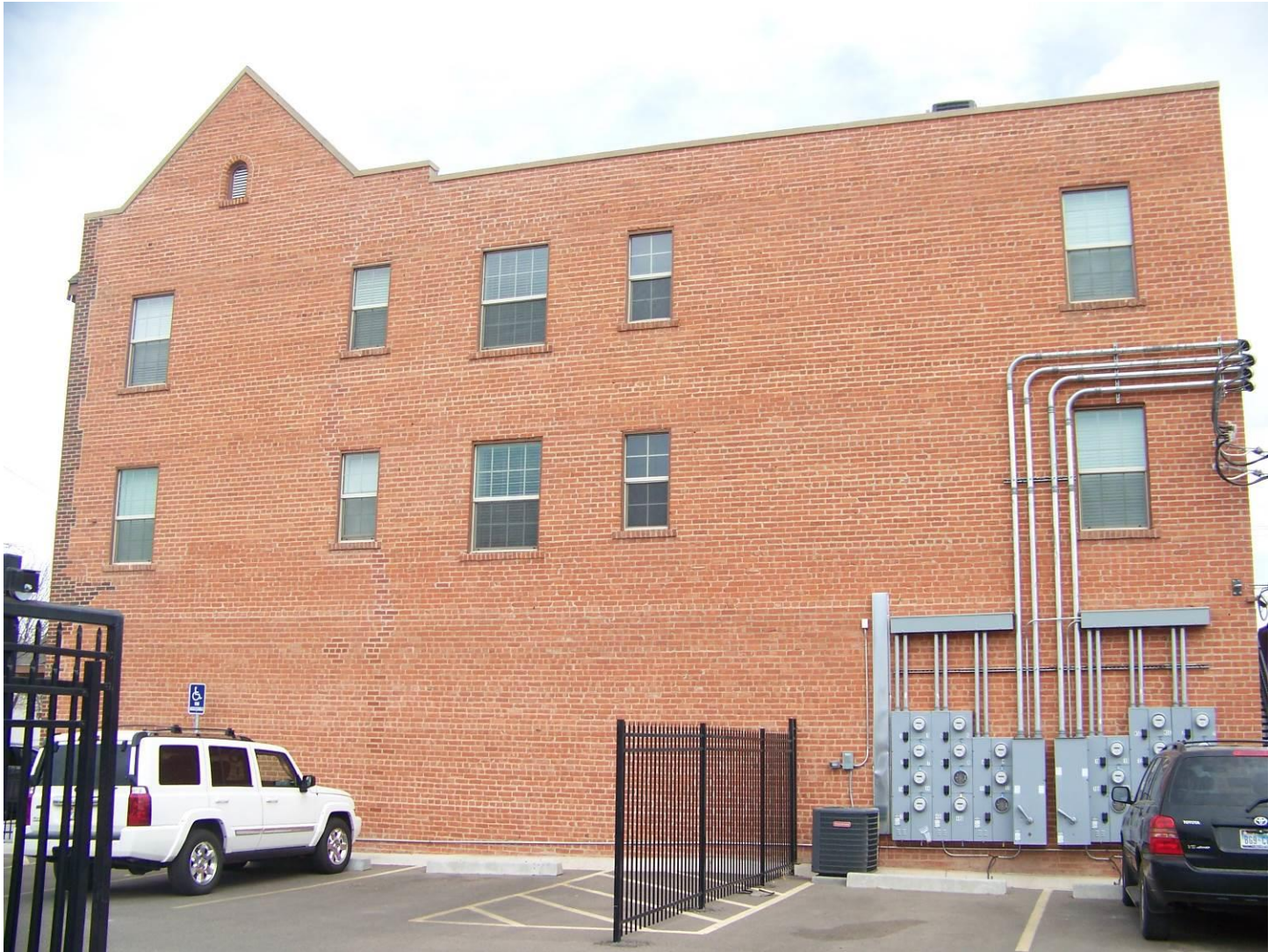
TX_Potter County_Vineyard Manor_0004.tif South elevation. Camera facing approximately north.
