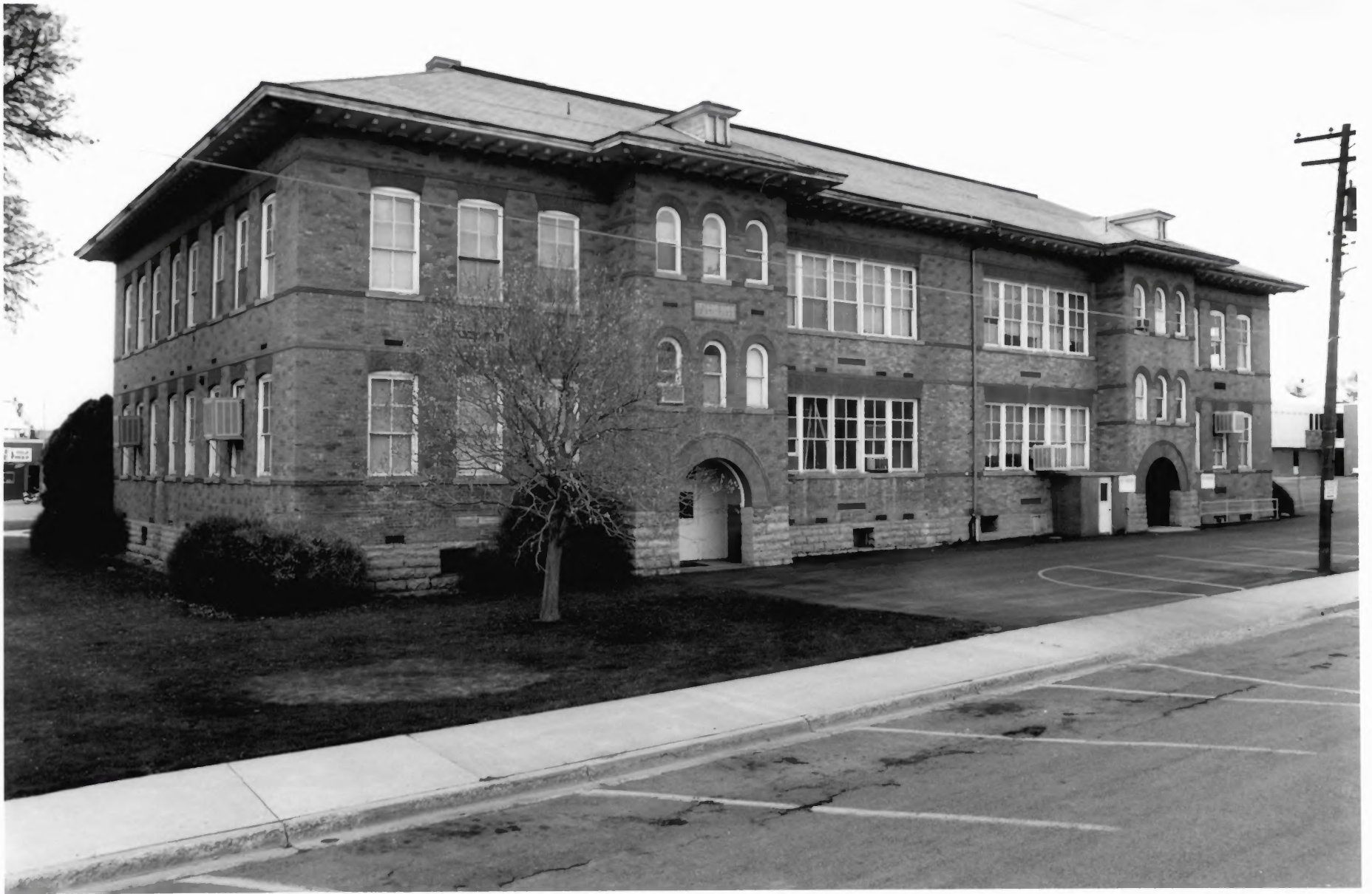
HARRINGTON ELEMENTARY SCHOOL AMERICAN FORK, UTAH CO., UT PHOTO#1
