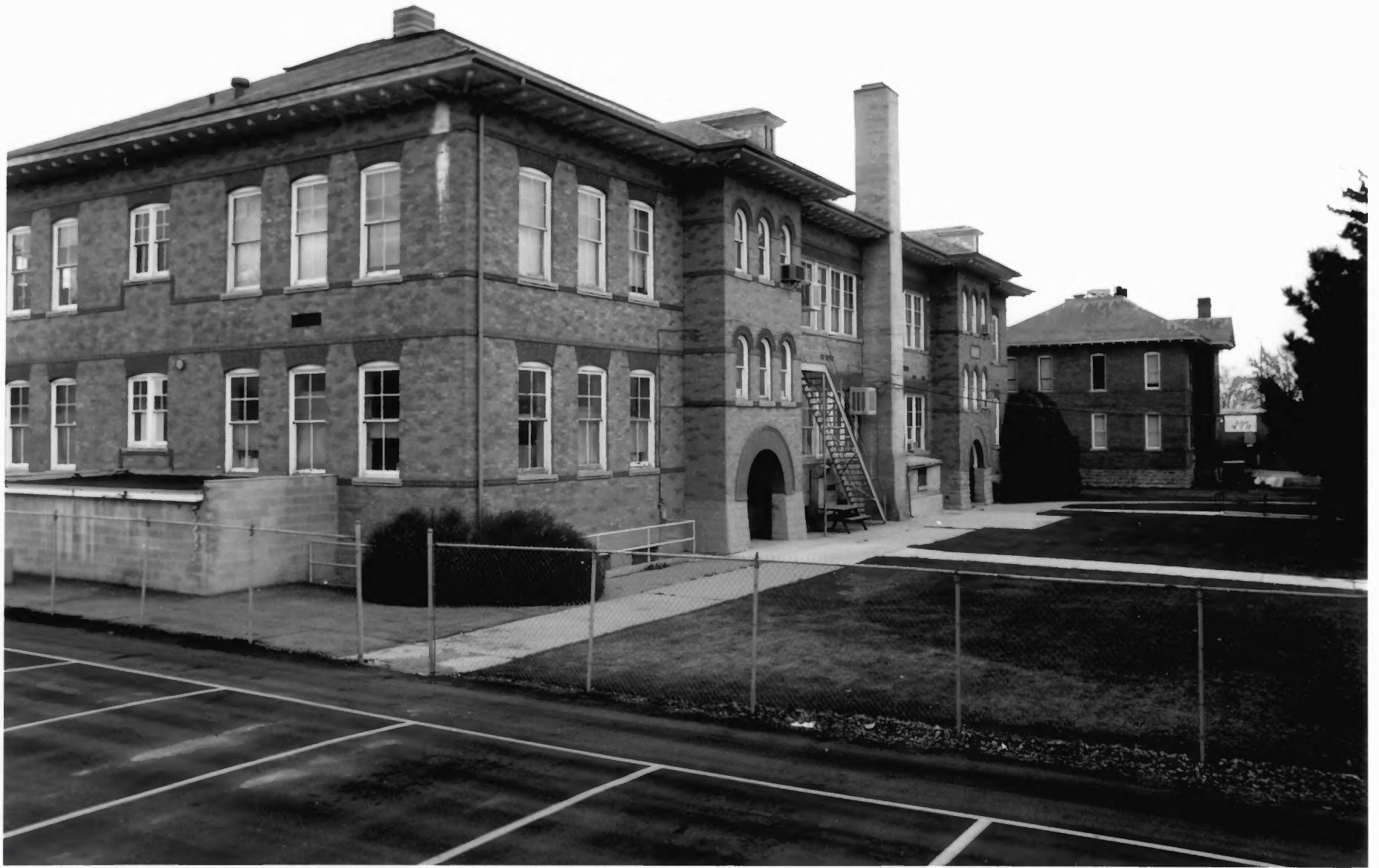
HARRINGTON ELEMENTARY SCHOOL AMERICAN FORK, UTAH CO., UT PHOTO #2
