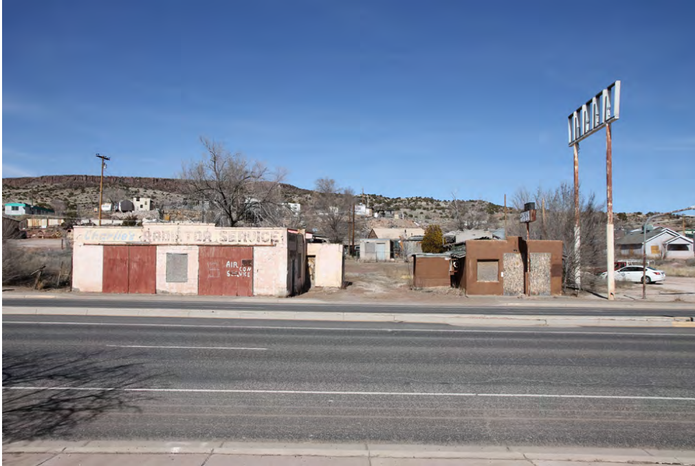
1 of 18. Diaz property with garage (left), Star Café (right), and Diaz House (rear of property), with U.S. 66 (foreground) and Black Mesa (background), photographer facing northeast.
