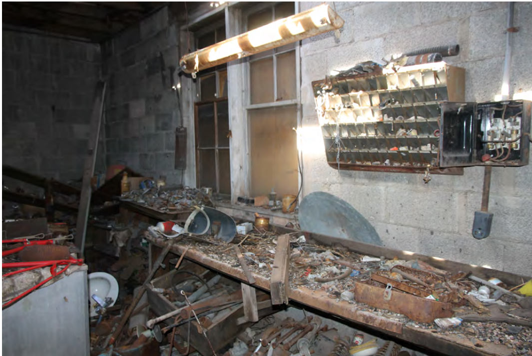
11 of 18. Interior, work bench on north wall, photographer facing northwest.
