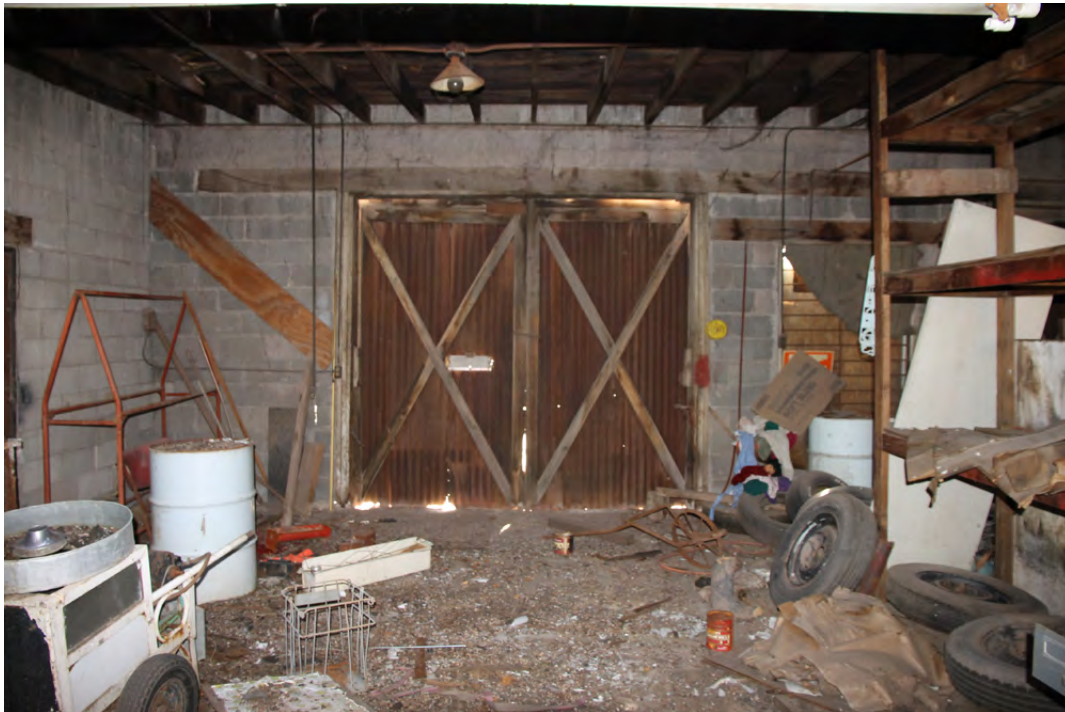
8 of 18. Interior, west service bay, photographer facing southwest.
