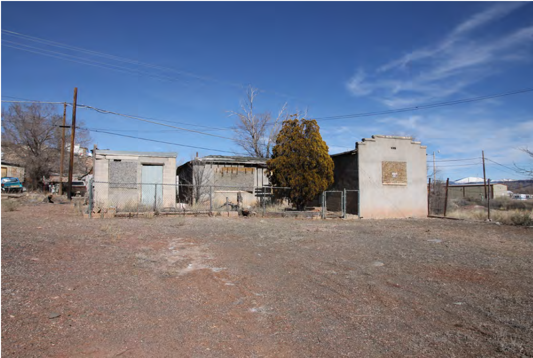
17 of 18. Diaz House and shed (left), rear facade, photographer facing northeast.
