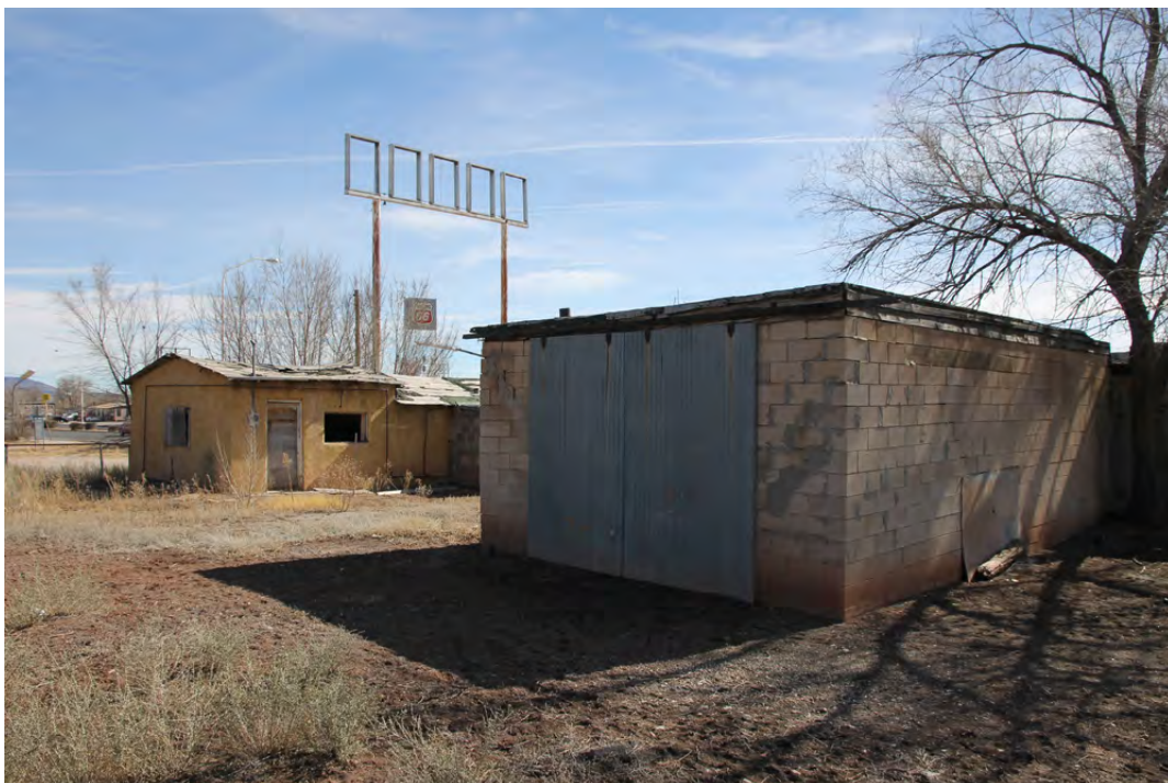
6 of 18. Rear of Star Café (left) and rear of Charley's Automotive Service (right), photographer facing southeast.
