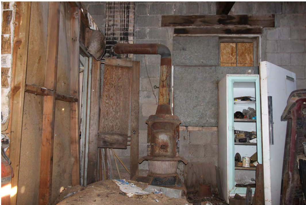
10 of 18. Interior, cast-iron stove in west service bay, photographer facing southeast.
