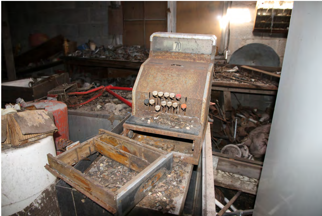
13 of 18. Interior, cash register, photographer facing northwest.
