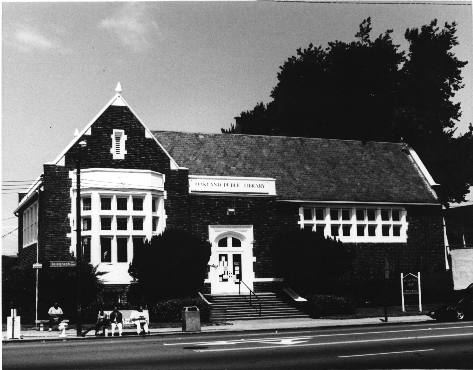
Oakland Free Library, Alden Branch; Oakland, Alameda County CA #1
