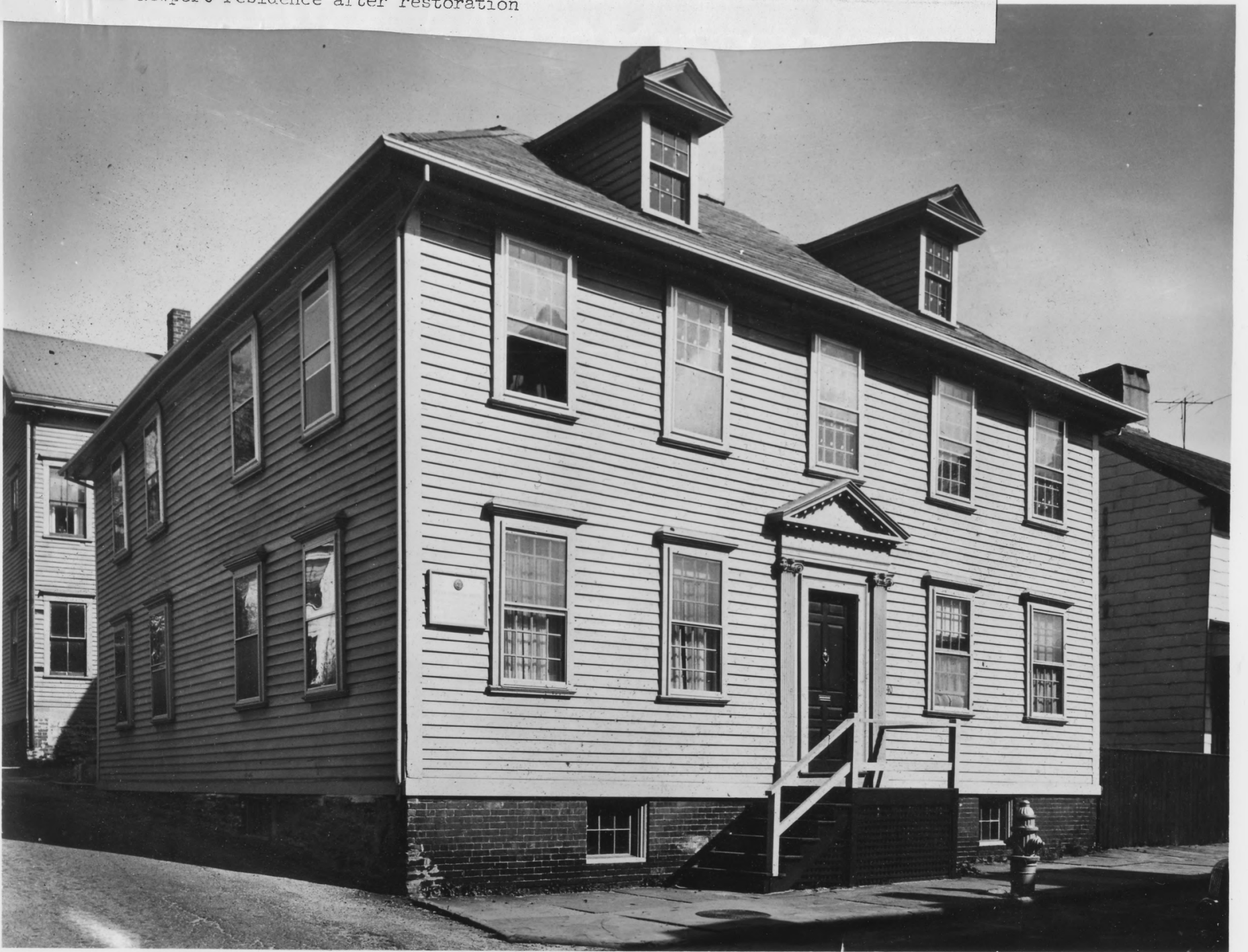
The same Newport residence after restoration
